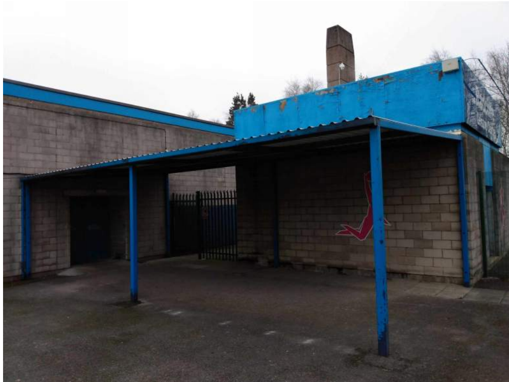
57) West end of boiler house of Leisure Centre
