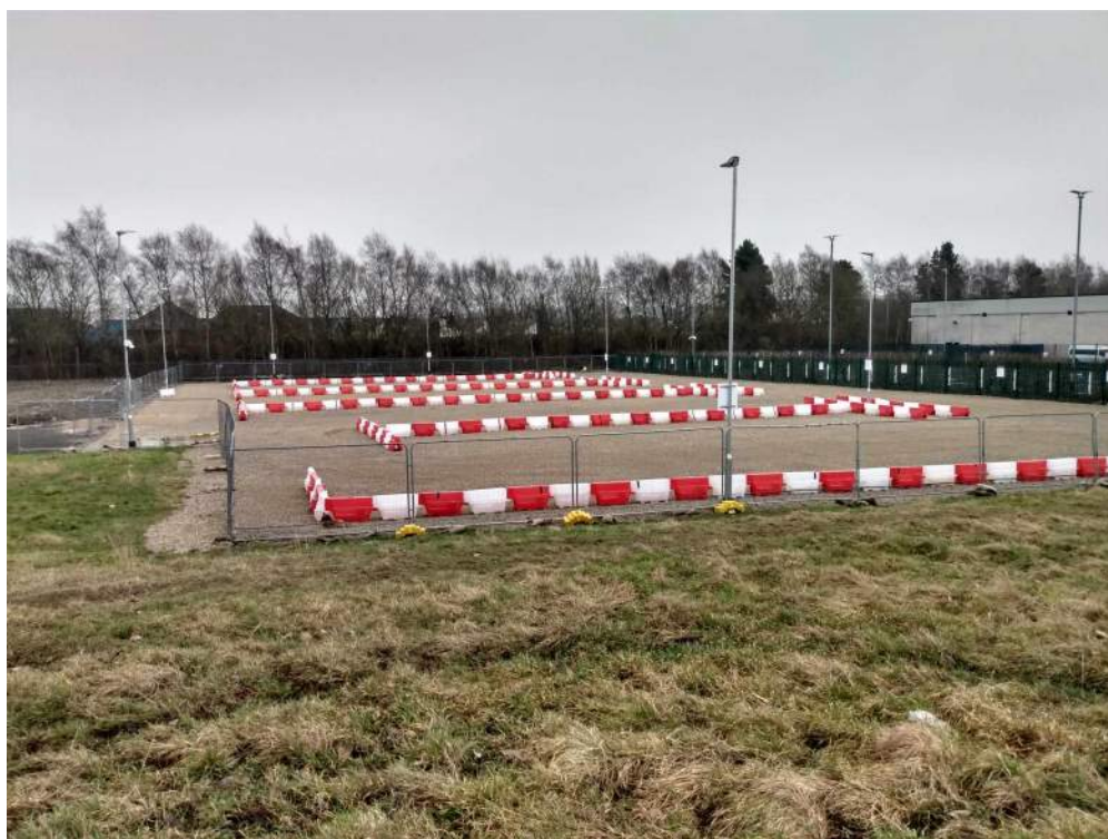
32) New gravel-surfaced car parking area north of car park adjacent to Spring Lane School
