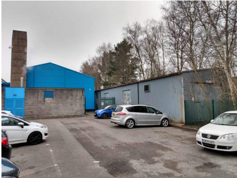
11) Boiler house, chimney and grey disused Radcliffe Sub Station on east (right) side
