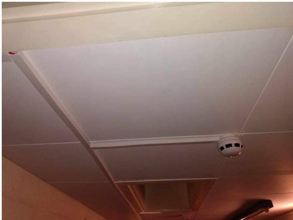
8) Asbestos cement ceiling tiles of Leisure Centre building with overhead hatch in background
