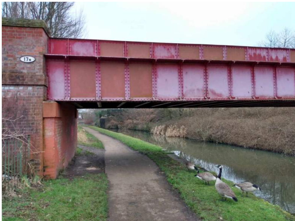
20) Bridge 17e of the Manchester. Bolton & Bury Canal
