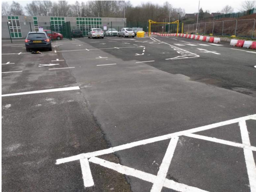
35) Tarmacadam car park on former tennis courts north of Spring Lane School
