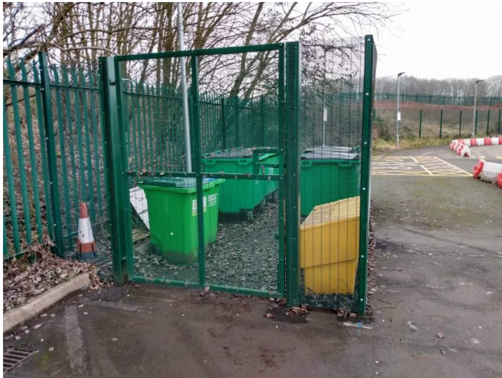
39) Recycling bin store near entrance to Spring Lane School (looking north)
