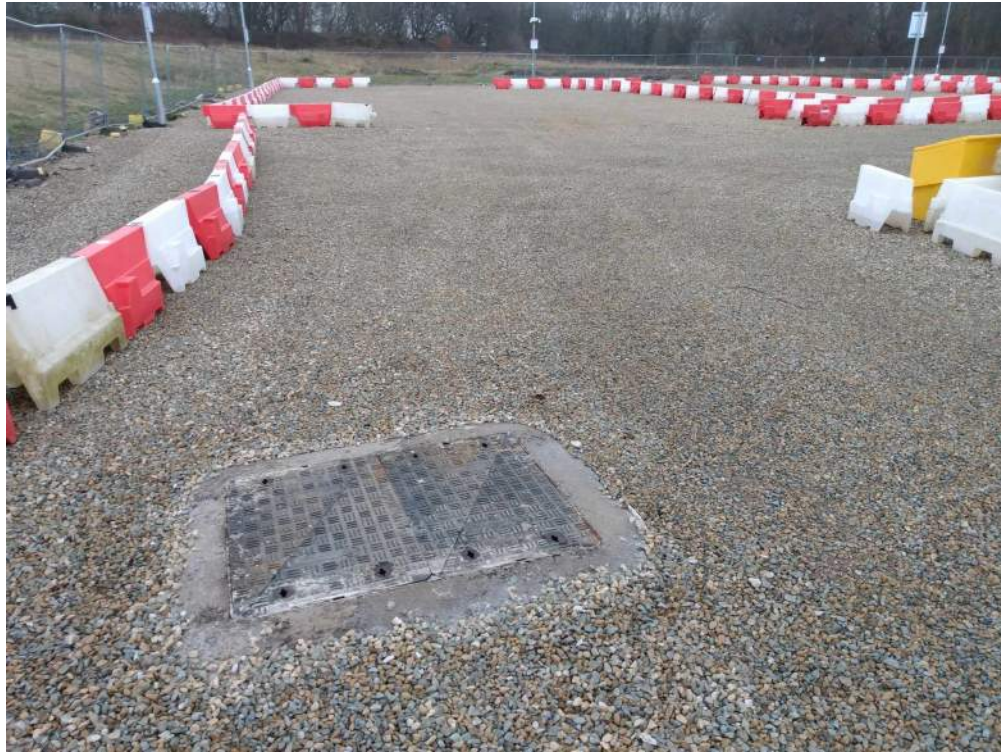
33) Looking north over new gravel-surfaced car parking area
