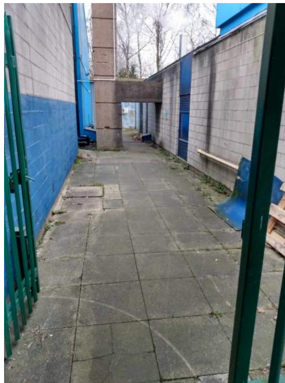
58) Looking east along passage to boiler house chimney
