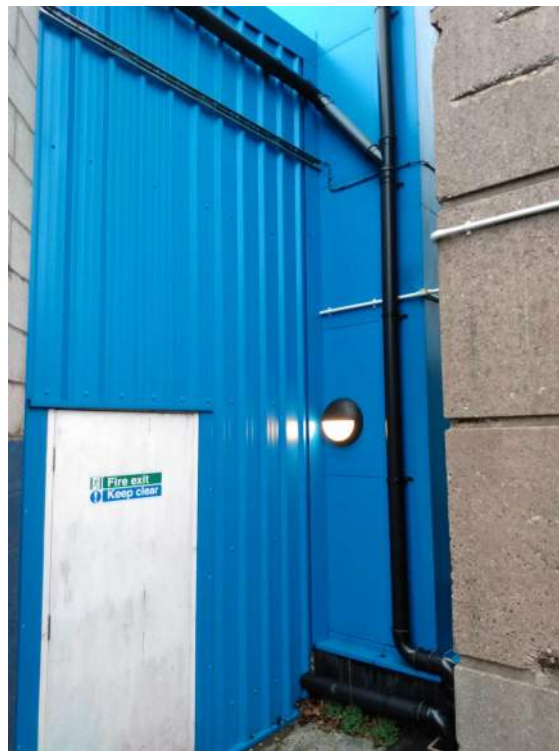
60) Fire exit from blue swimming pool building
