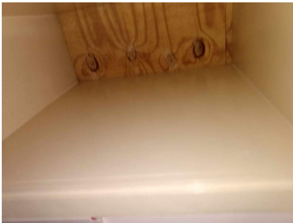
9) Plywood boards blocking overhead hatch in Leisure Centre building
