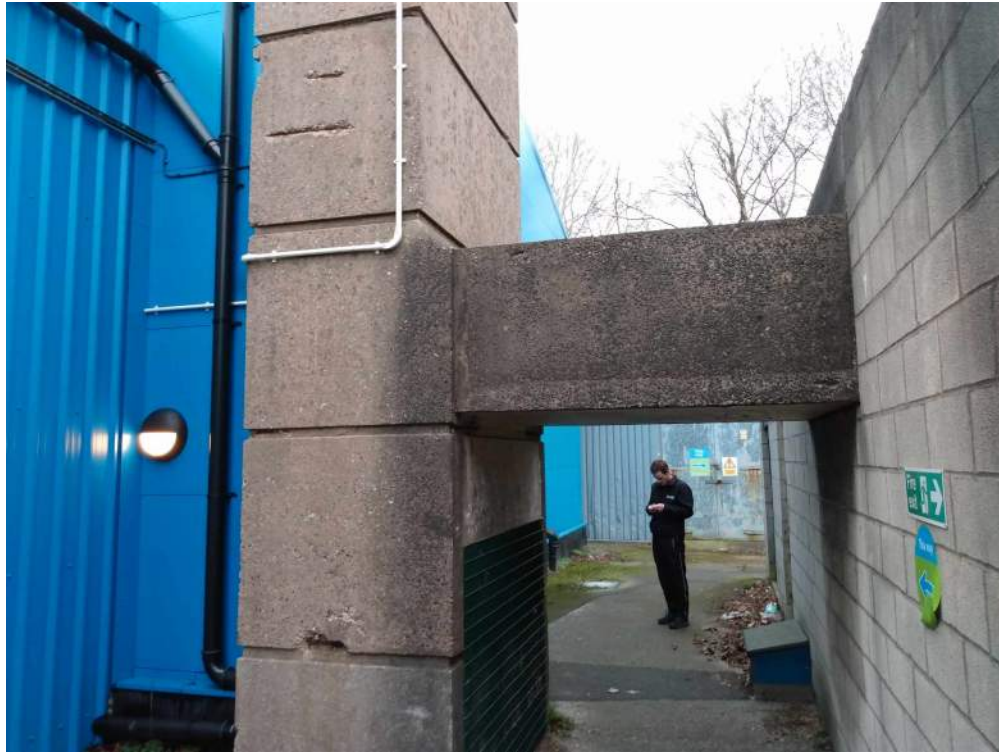
59) Boiler house to south (right) of chimney
