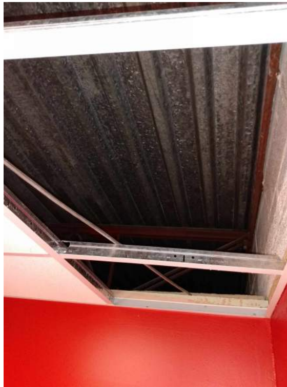
7) Asbestos cement ceiling tiles
