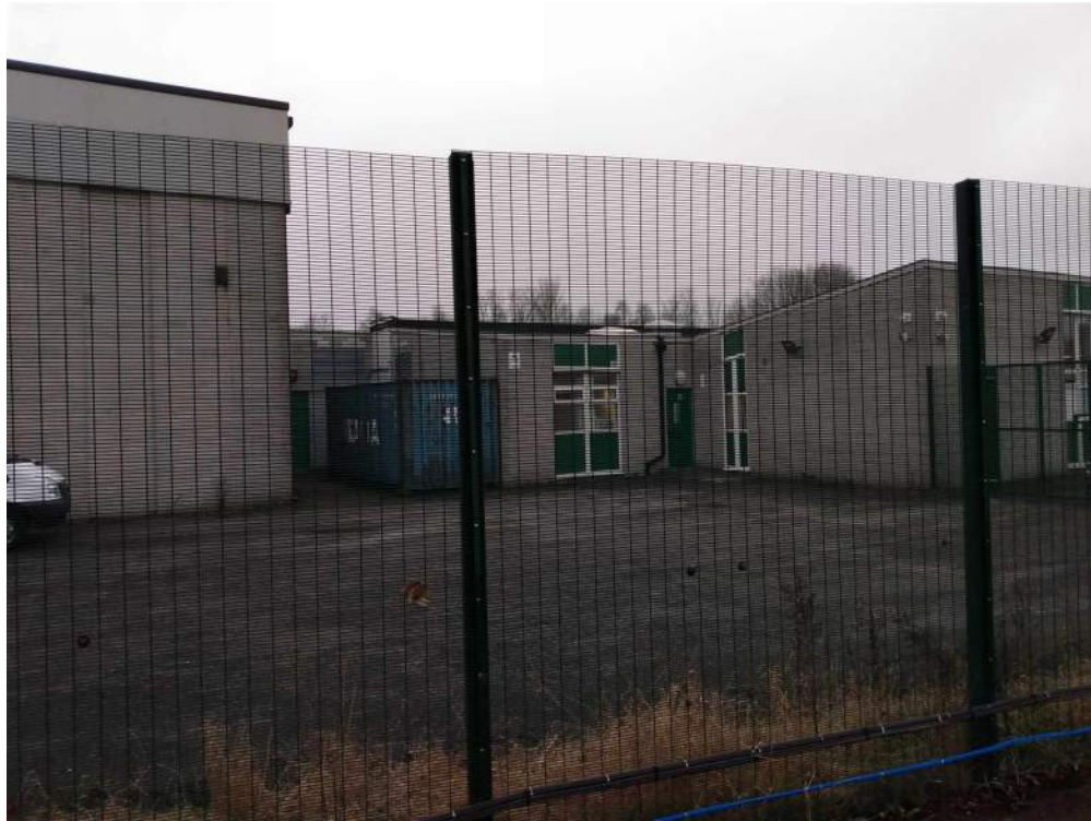
47) Looking south towards Plant Room between Sports Hall and blue shipping container
