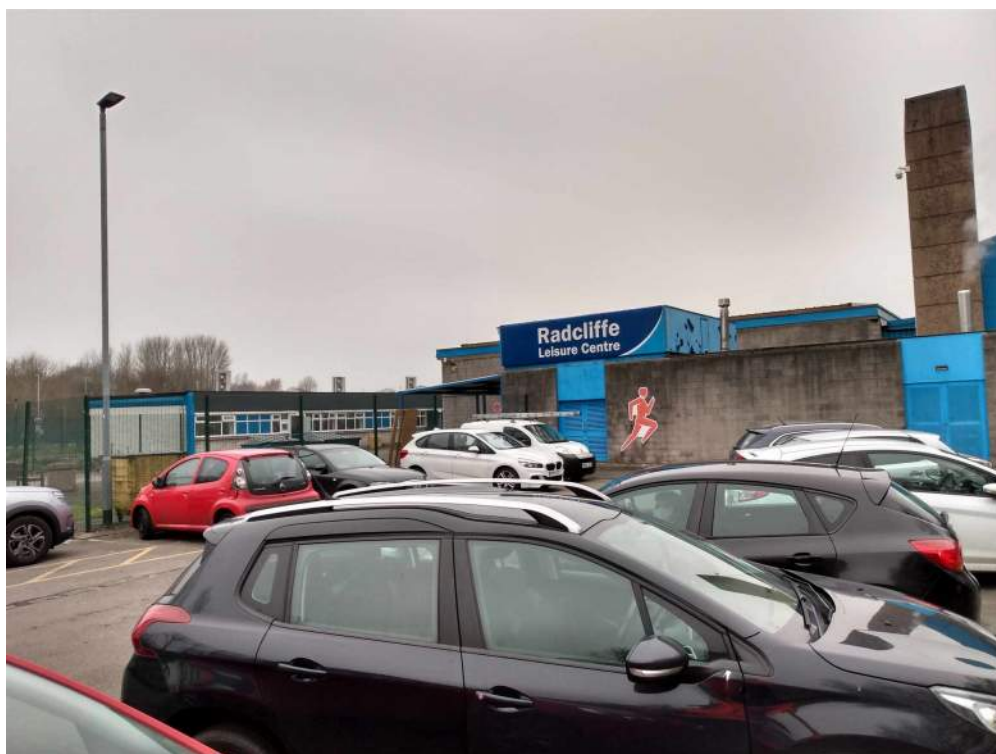
10) Radcliffe Leisure Centre with boiler house and chimney to the east (right) side
