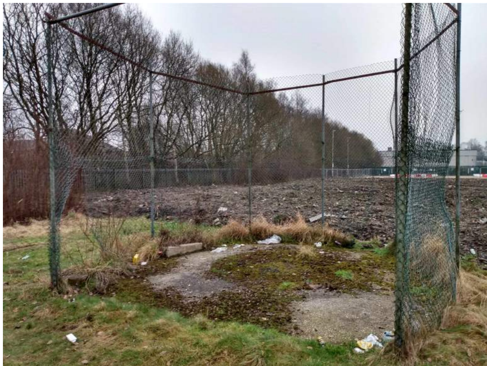
30) 5m diameter concrete base to former hammer and discus throwing area
