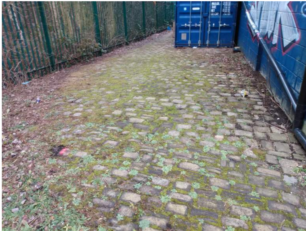
75) Looking south towards filtration unit on old cobbled roadway at rear of Sports Hall
