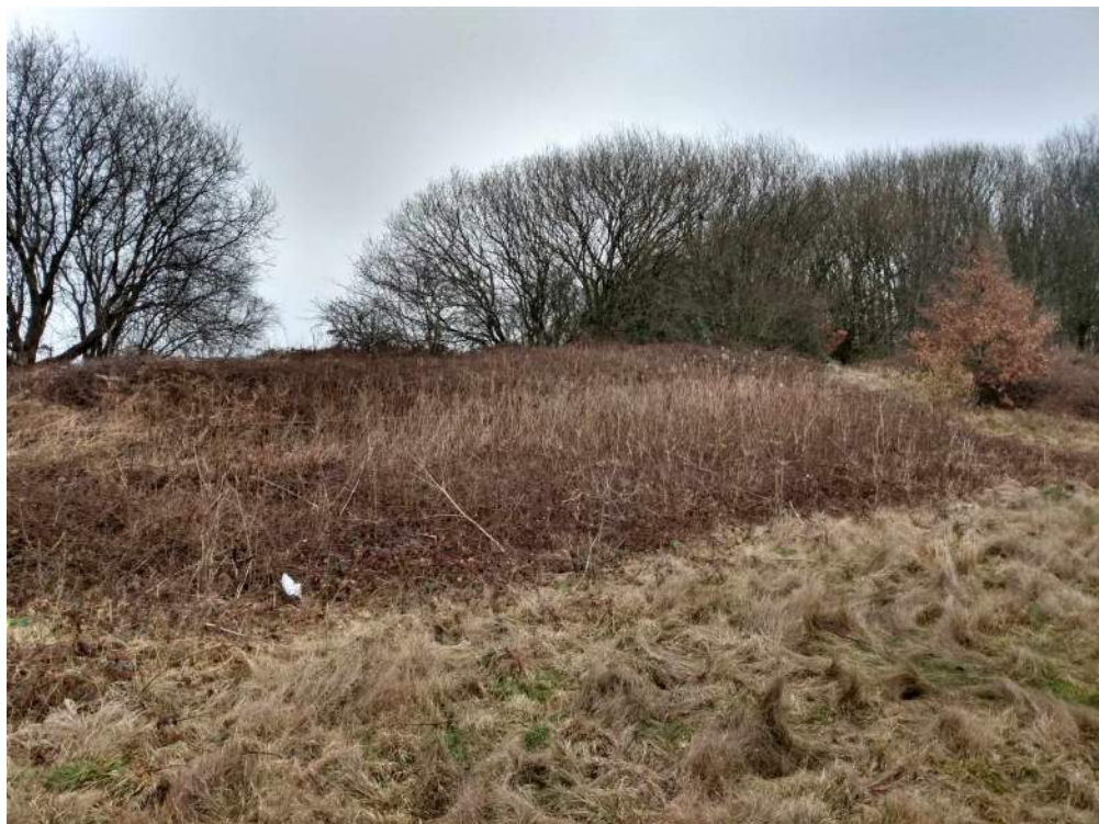
24) Embankment to the former L. & Y. R. Radcliffe West Fork
