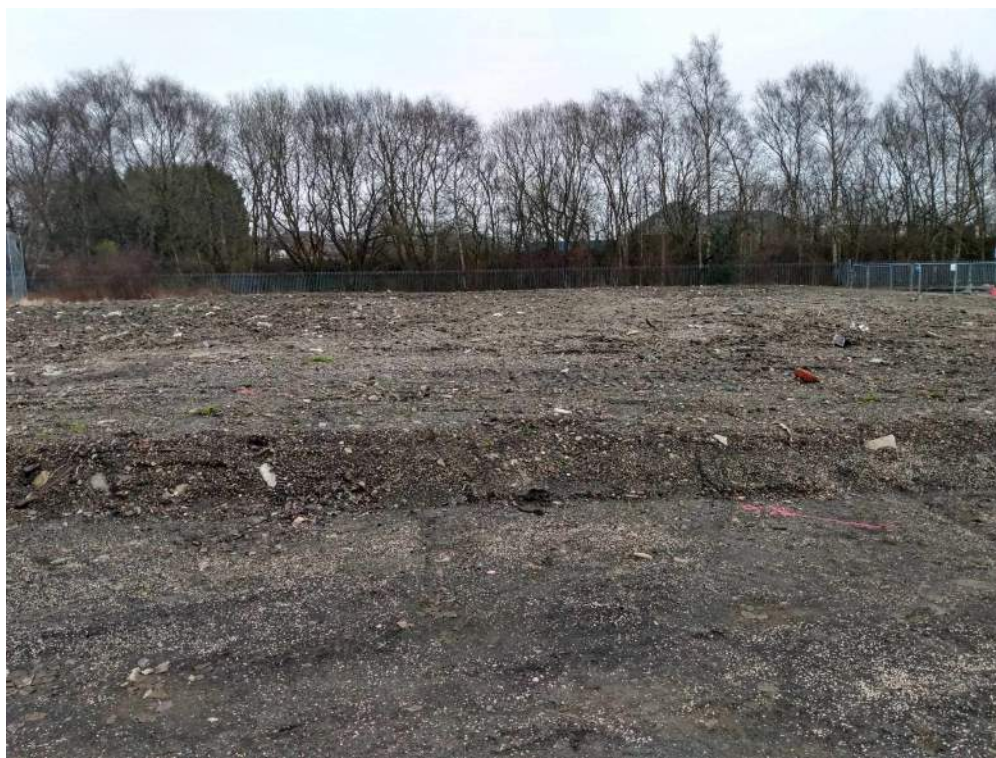
31) Construction rubble placed over former running track and athletics ground
