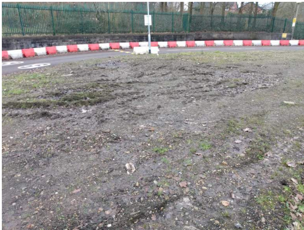
17) Rough ground, access road and stone retaining wall with Banana Path beyond
