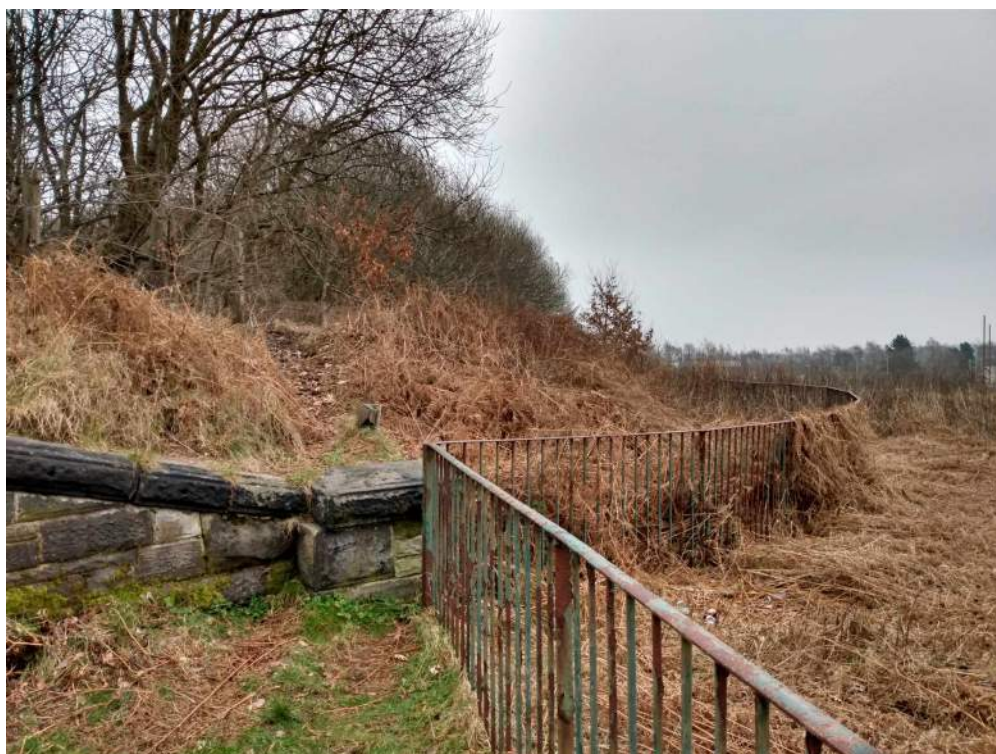
22) Wing wall of former bridge carrying L. & Y. R. Radcliffe West Fork over canal
