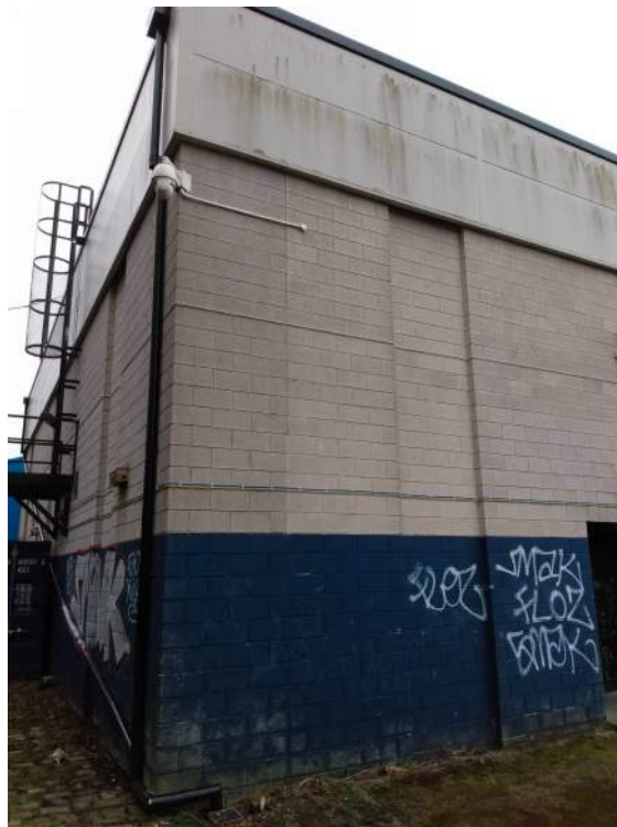
76) Northeast corner of Sports Hall
