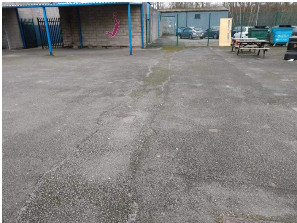
12) Looking east towards grey disused Radcliffe Sub Station
