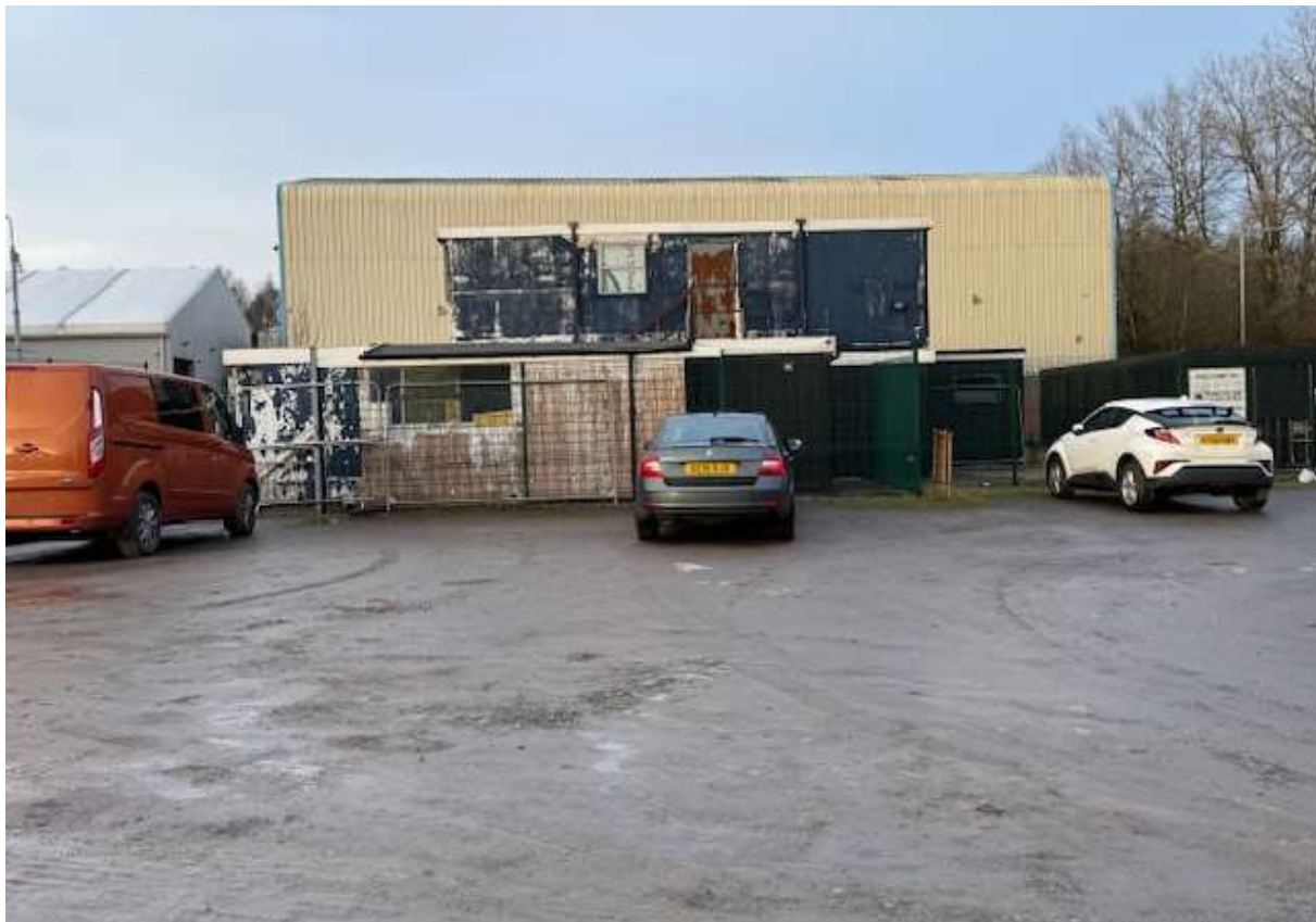
Photograph No 5 – Car Park and Training Centre to the North
