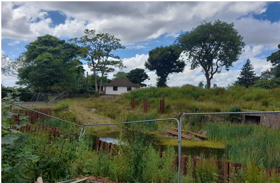
View of site to west prior to backfilling of basement excavation.
