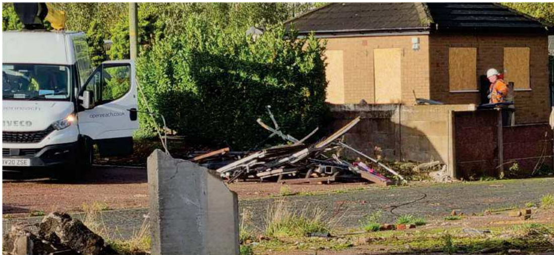
Figure 6: 26/10/22 – Openreach engineers on site disconnecting remaining services
