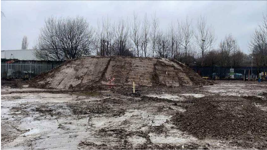
Figure 47: 3/02/23 – Western stockpile of clean certified subsoil (Stockpile 5)
