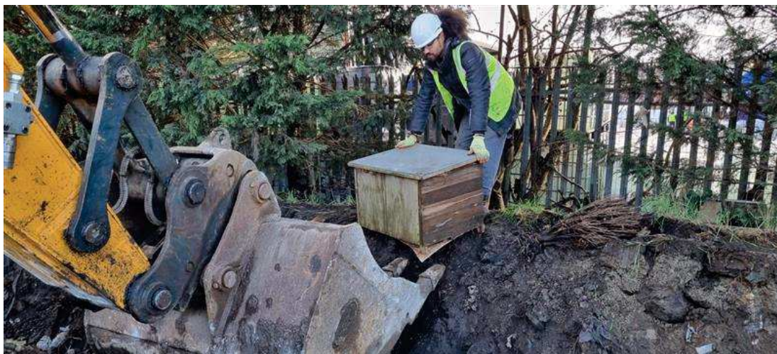
Figure 21 : 17/11/22 – Clearing existing general waste from treeline
