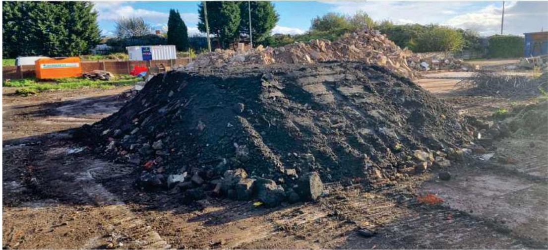
Figure 9: 4/11/22 – TP503 stockpiled on hardstanding ahead of removal from site to a licensed landfill facility
