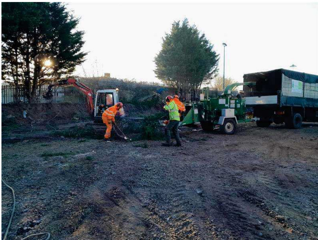
Figure 28 7/12/22 – Chipping felled trees from eastern boundary
