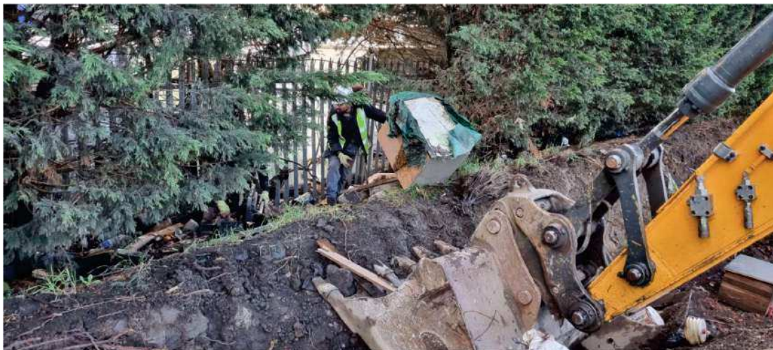
Figure 20: 16/11/22 – Waste from perimtere of site being hand-loaded into excavator bucket for transfer to waste skips
