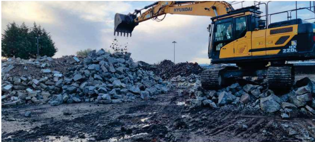
Figure 19: 16/11/22 – Oversize stockpile management
