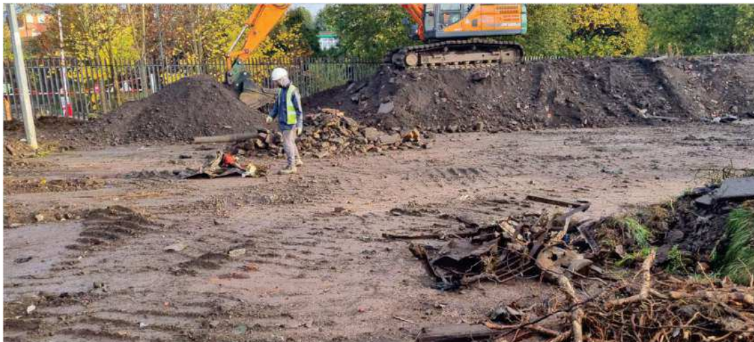
Figure 12 : 9/11/22 – Riddling perimeter bund material and separating waste into individual streams
