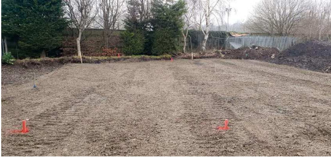
Figure 43 : 24/01/23 – Completed plot in SW of site
