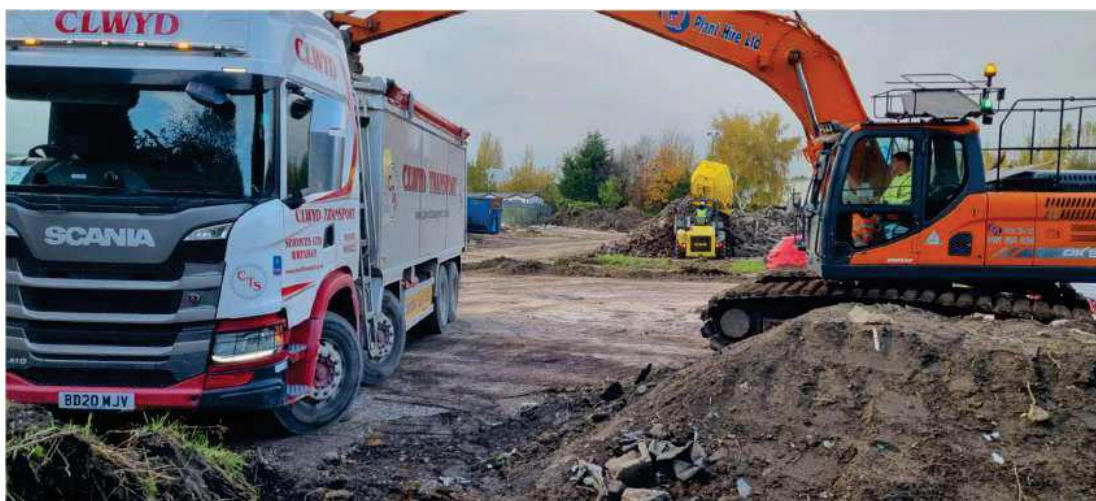
Figure 18: 15/11/22 – Loading contaminated (hazardous) soils into 8WT for disposal at Provectus in Crewe
