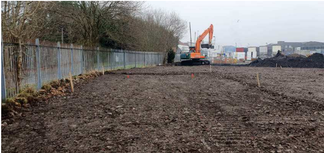
Figure 44 : 24/01/23 – Completed plot in NW of site
