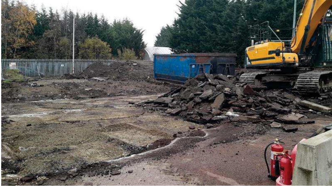
Figure 25 : 1/12/22 – Lifting and stripping areas of tarmac surfacing
