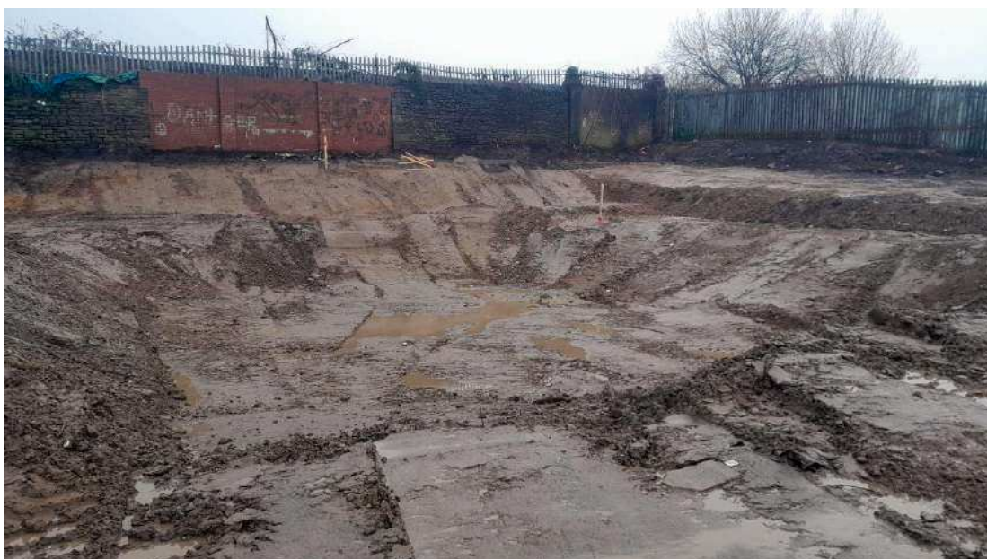
Figure 34 : 23/12/22 – Completed excavation for subsoils
