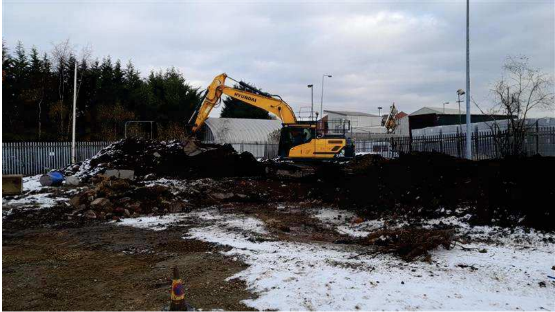
Figure 31 : 12/12/22 – Processing perimeter bund in north-east corner
