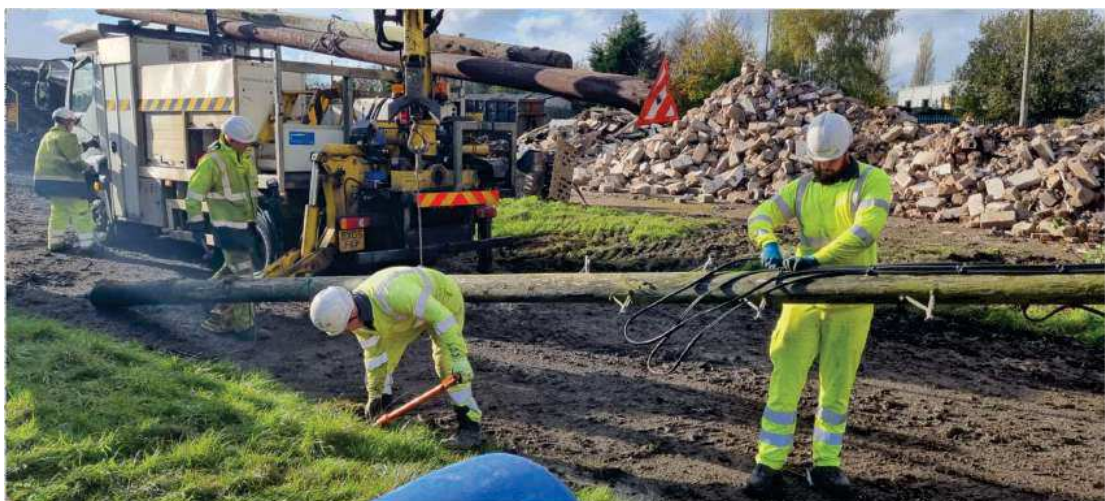
Figure 14 : 9/11/22 – Openreach engineers return to site to remove redundant telephone poles
