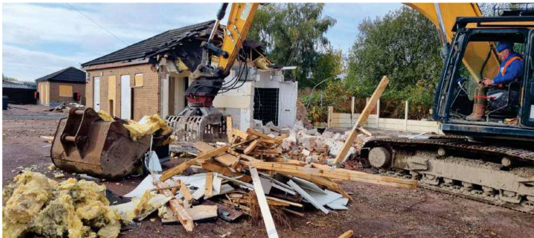
Figure 2 : 24/10/22 – Excavator with selector grab segregating demolition material into separate waste streams
