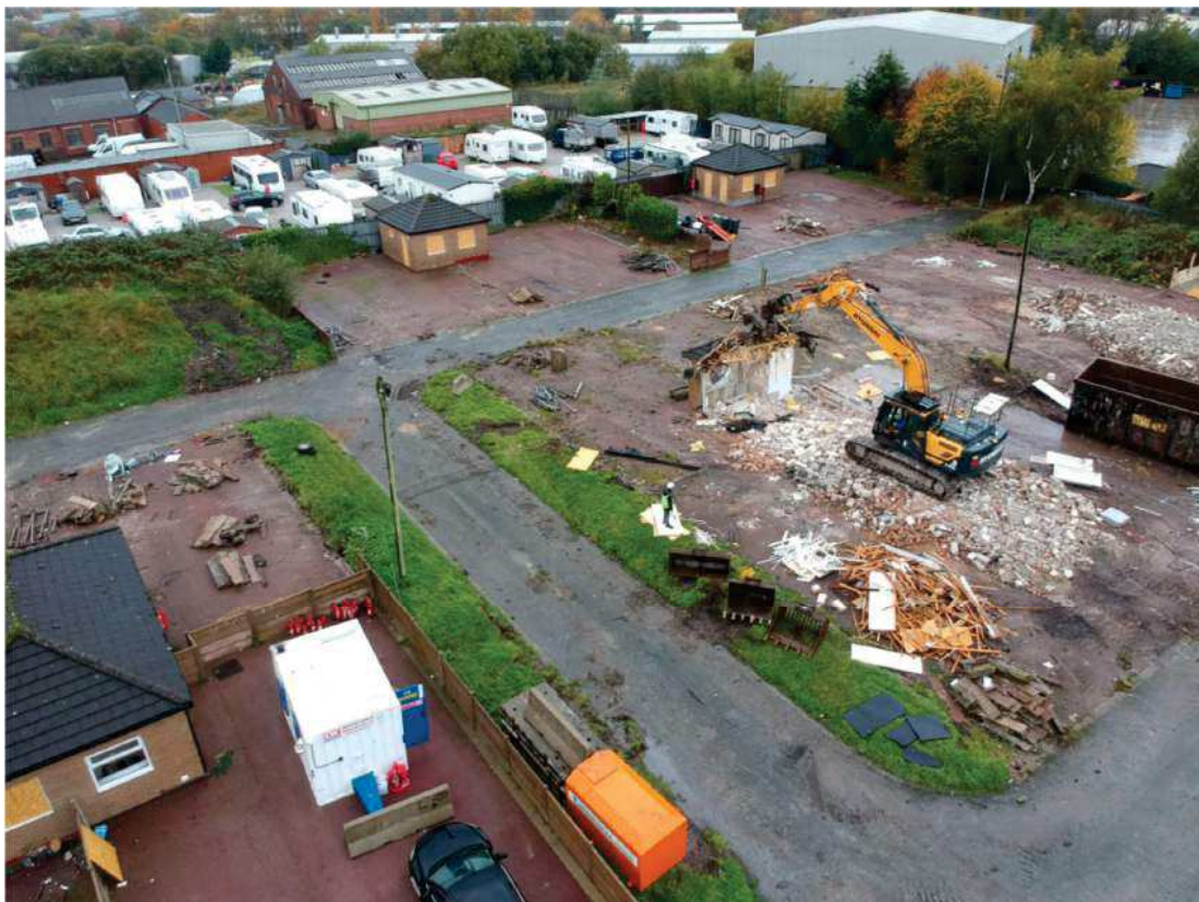
Figure 4 : 27/10/22 - Excavator demolishing/segregating materials from central building
