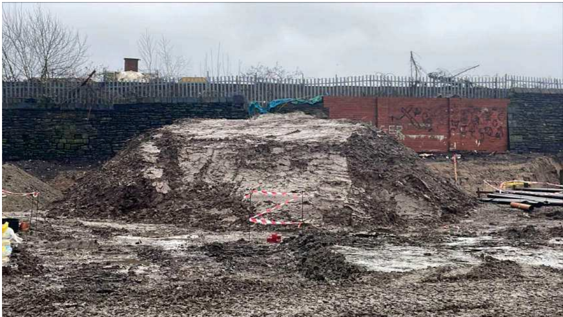
Figure 48 : 3/02/23 – Eastern stockpile of clean certified subsoil (Stockpile 6)
