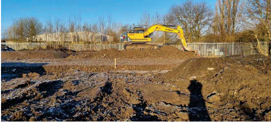
Figure 41 : 23/01/23 – Placement of granular fill to plots
