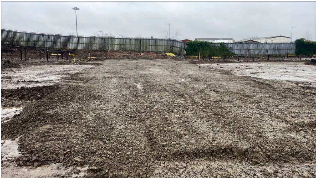
Figure 46 : 3/02/23 – Stoned-up access and pad for concrete pump (eastern pad)
