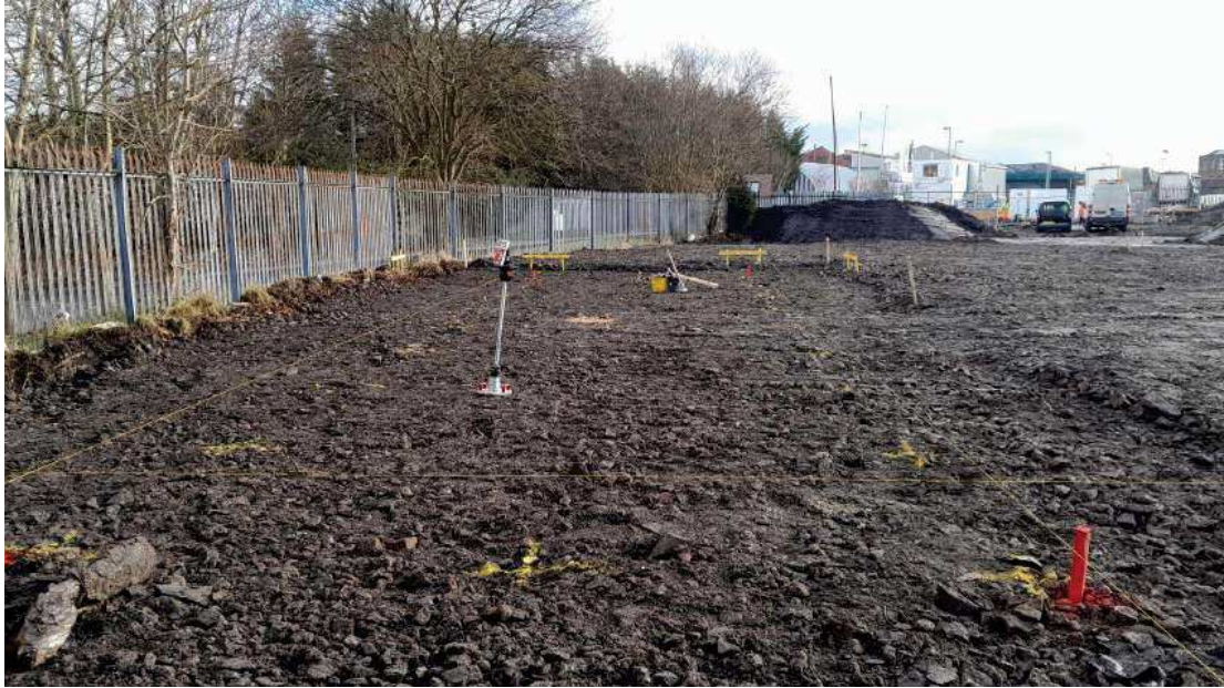
Figure 45 : 27/01/23 – Lightweight Deflectometer testing on completed pile mat
