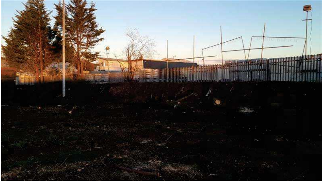
Figure 29 : 7/12/22 – Treefelling works almost complete
