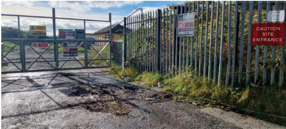
Figure 3 : 25/10/22 – Reinforced access gates displaying appropriate site safety signage
