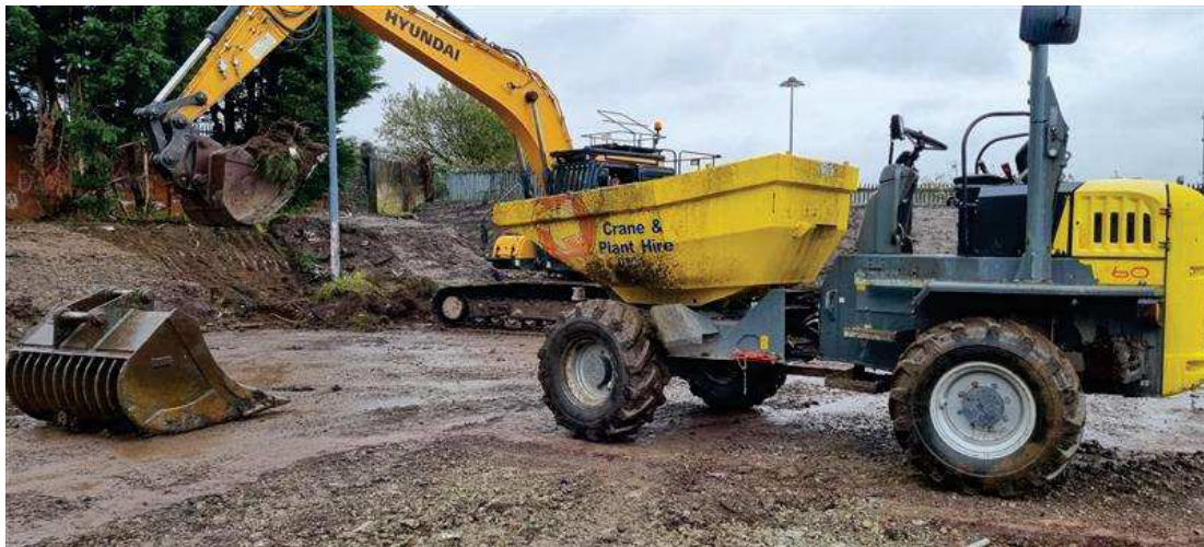
Figure 23 : 18/11/22 – Separating vegetation from remaining edge bunds
