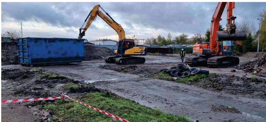
Figure 22 : 17/11/22 – Relocating scrap metal skip during operations
