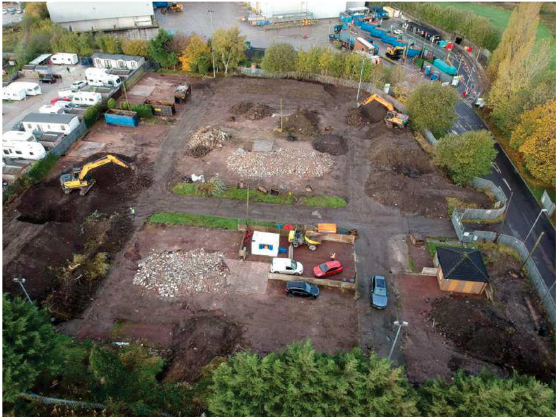
Figure 13 : 9/11/22 – Stockpile management; riddling of bunds to remove oversize material for processing
