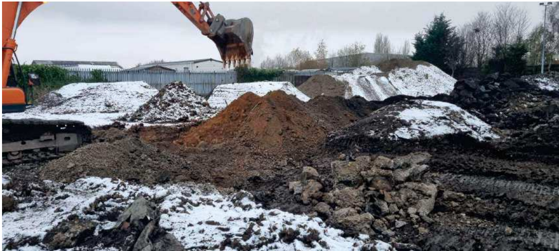
Figure 32 : 13/12/22 – Segregation of materials into stockpiles
