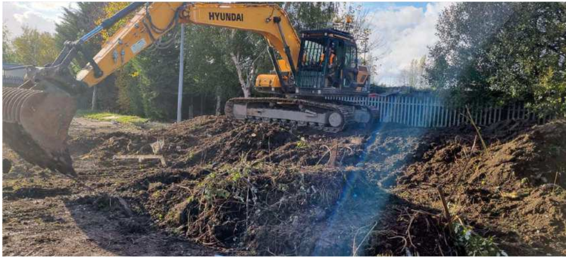
Figure 7: 3/11/22 – Vegetation scrape and segregation of green waste
