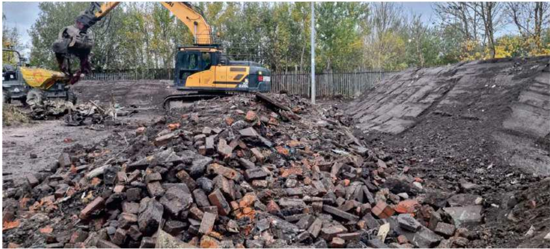
Figure 15 : 10/11/22 – Separating waste from oversize
