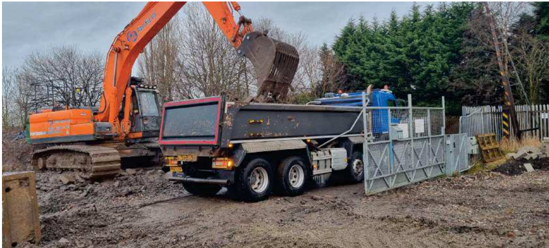
Figure 37: 12/01/23 – Disposal of last remaining oversized material
