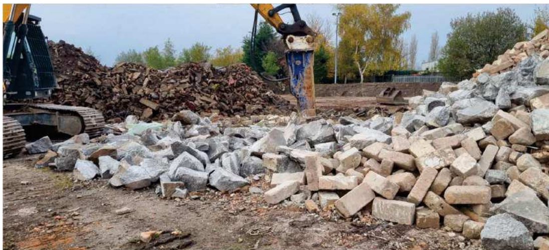
Figure 17: 15/11/22 – Utilising hydraulic breaker to process larger pieces of oversize ahead of crushing
