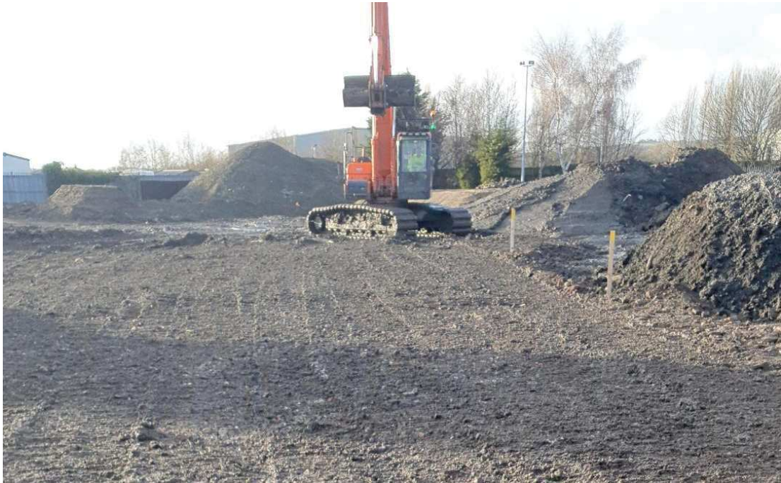
Figure 35 : 29/12/22 – PLacement of crush to access road
