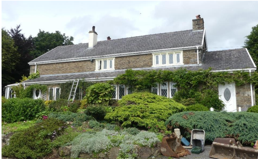
Figure 2.7: The principle, south-western, elevation of the farmhouse
