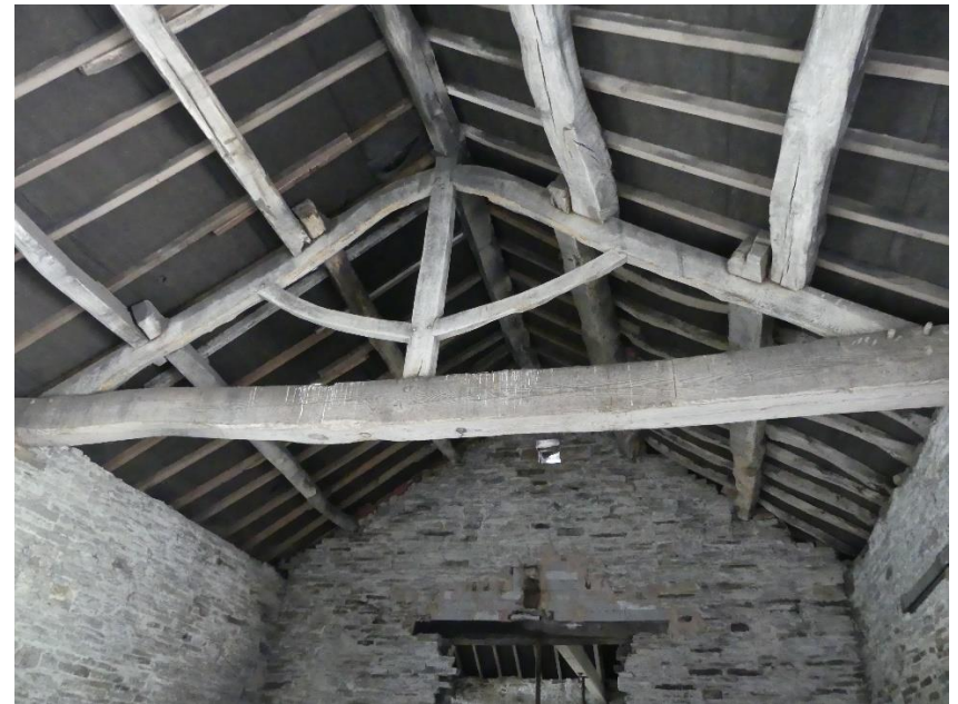
Figure 2.17: The western truss in the original phase of the barn
