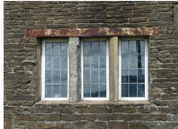
Figure 2.14: The mullioned window to the south-western elevation
