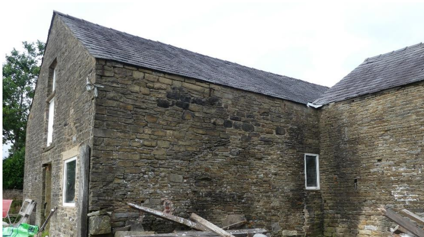
Figure 2.13: The scare of a previous roof form on the side elevation
