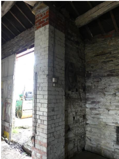
Figure 2.16: The brick support to the eastern truss
