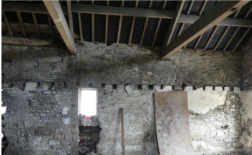
Figure 2.18: The vertical joint and quoins to the left of the partly blocked doorway illustrate the south-western corner of the original barn inside the western range. The former first floor level of the western range is evident below the trusses and the right-hand part of the wall appears to incorporate a previous roofline.
