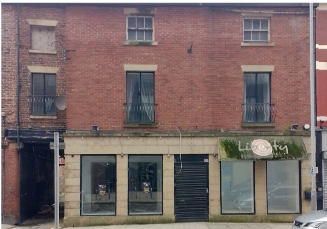
Photograph 1 - Front elevation of the property from The Rock.
