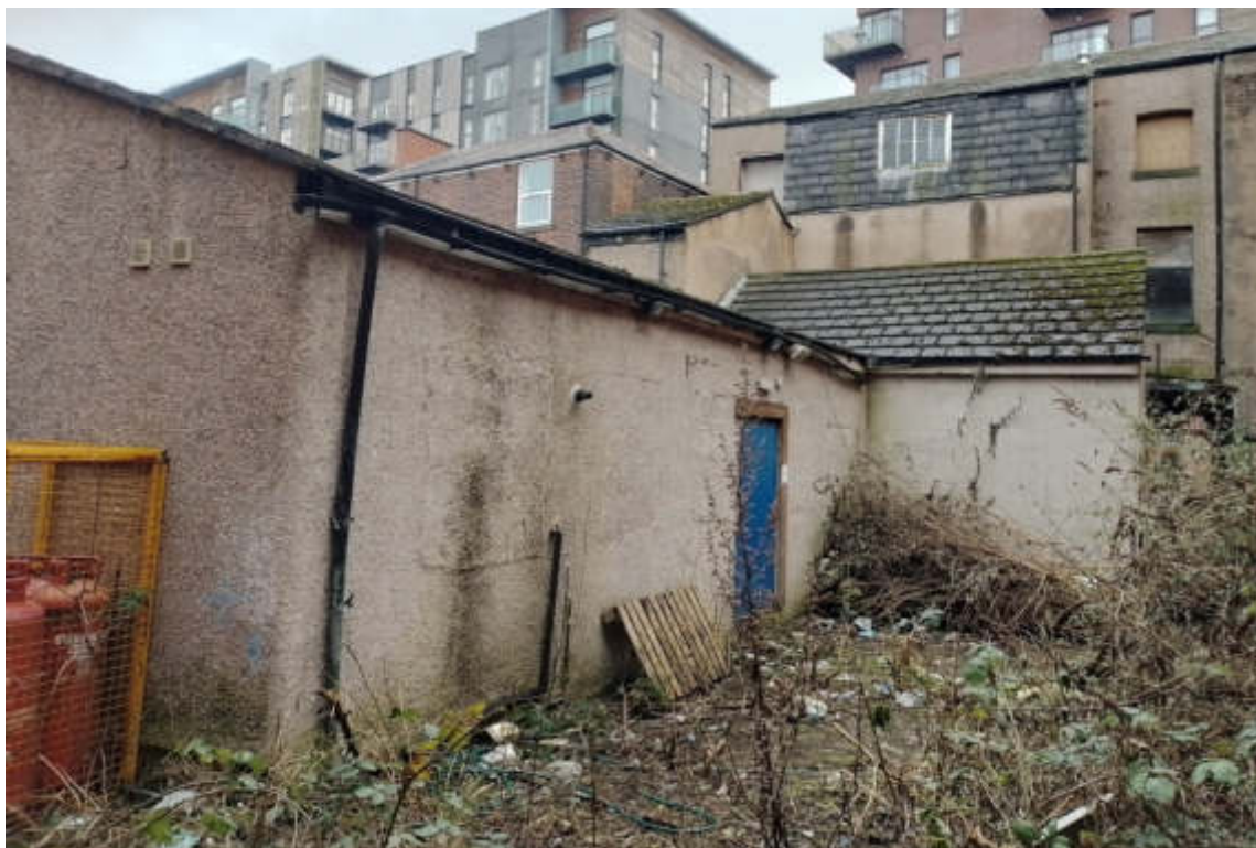
Photograph 3 - Rear buildings and central western courtyard.
