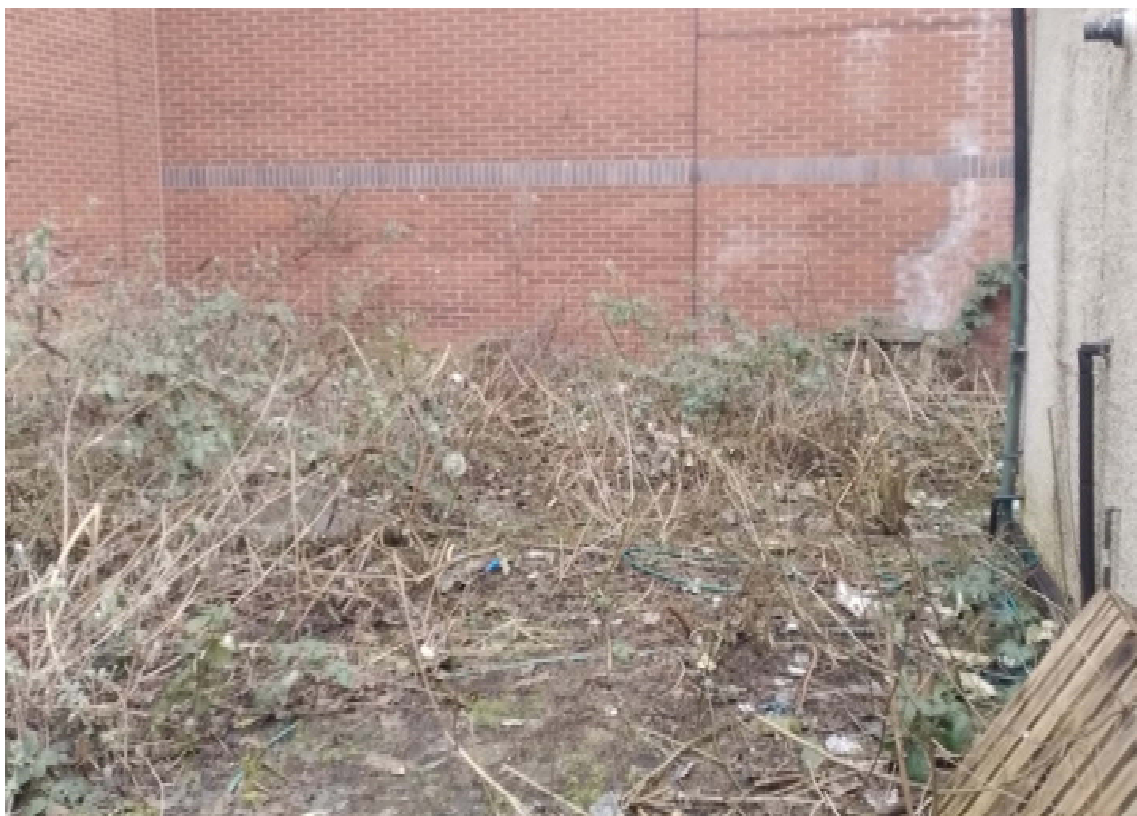
Photograph 5 - North boundary wall and central western courtyard.
