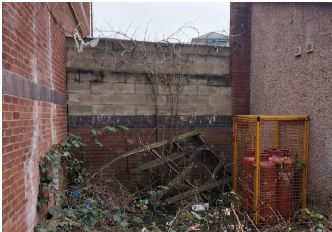
Photograph 4 – North east boundary wall and container storage.
