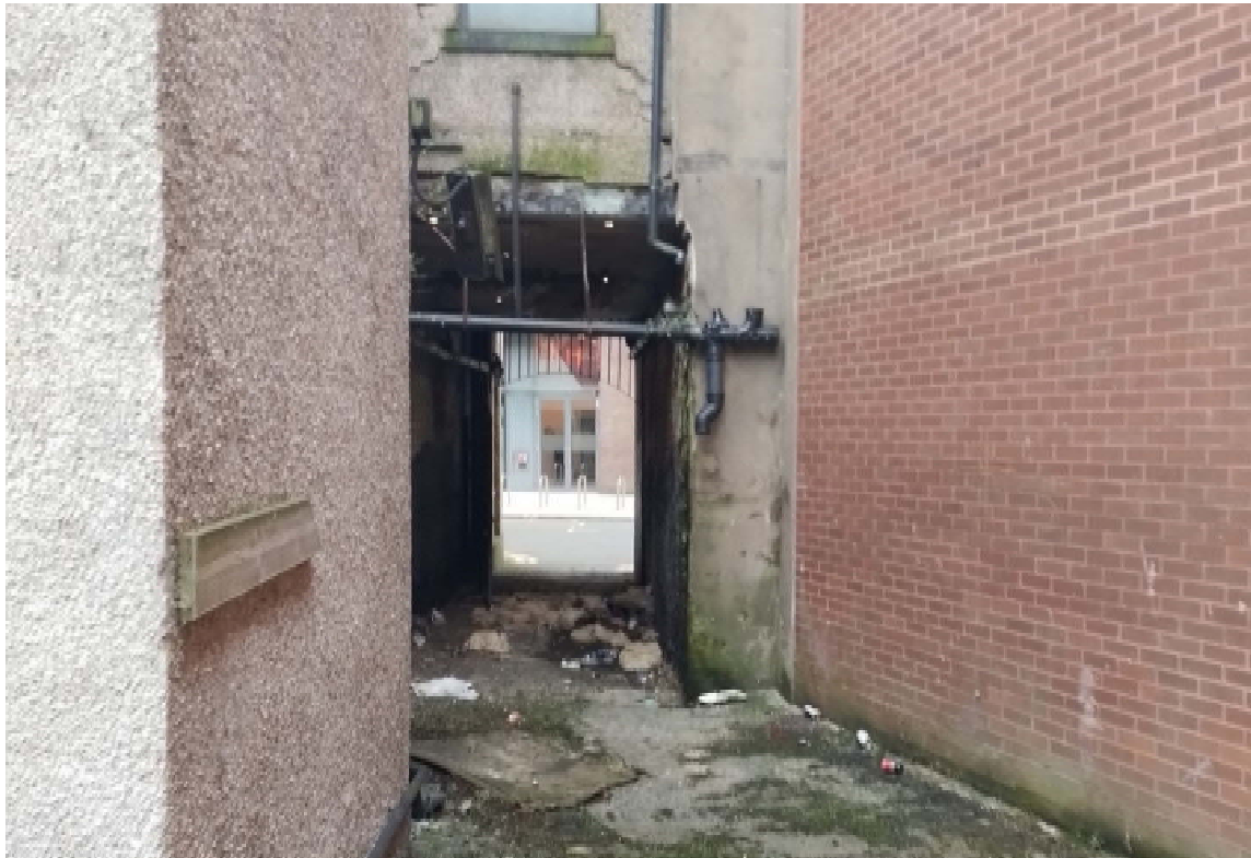
Photograph 7 - West boundary wall, central western courtyard and alley on the west side of the property.
