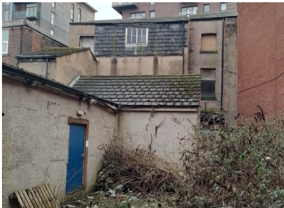
Photograph 2 - Rear elevation of the property.
