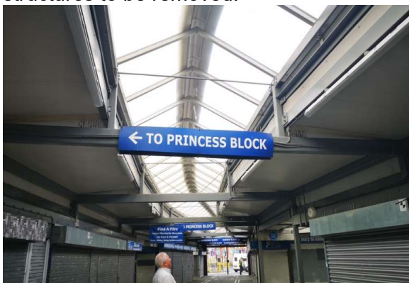
Typical Existing Canopy
