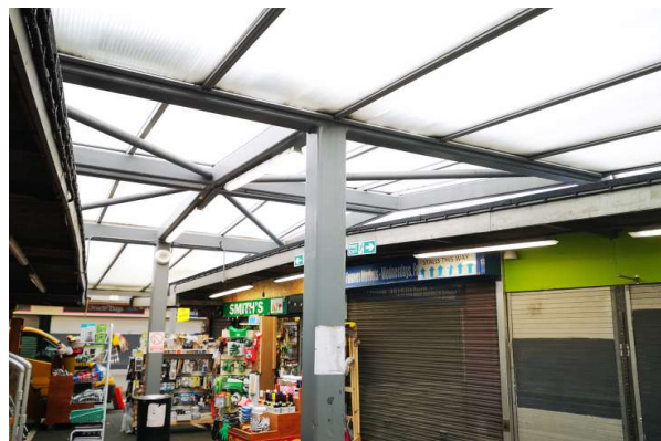
Typical Existing Canopy
