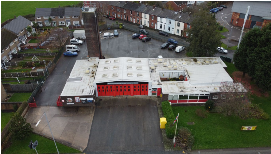
Existing Whitefield Fire Station
