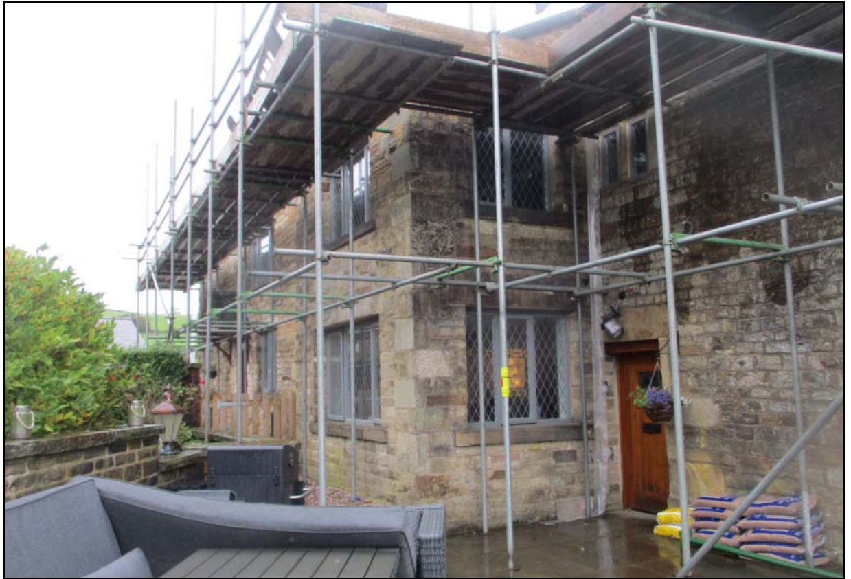
The rear wing has been greatly altered during conversion to domestic use
