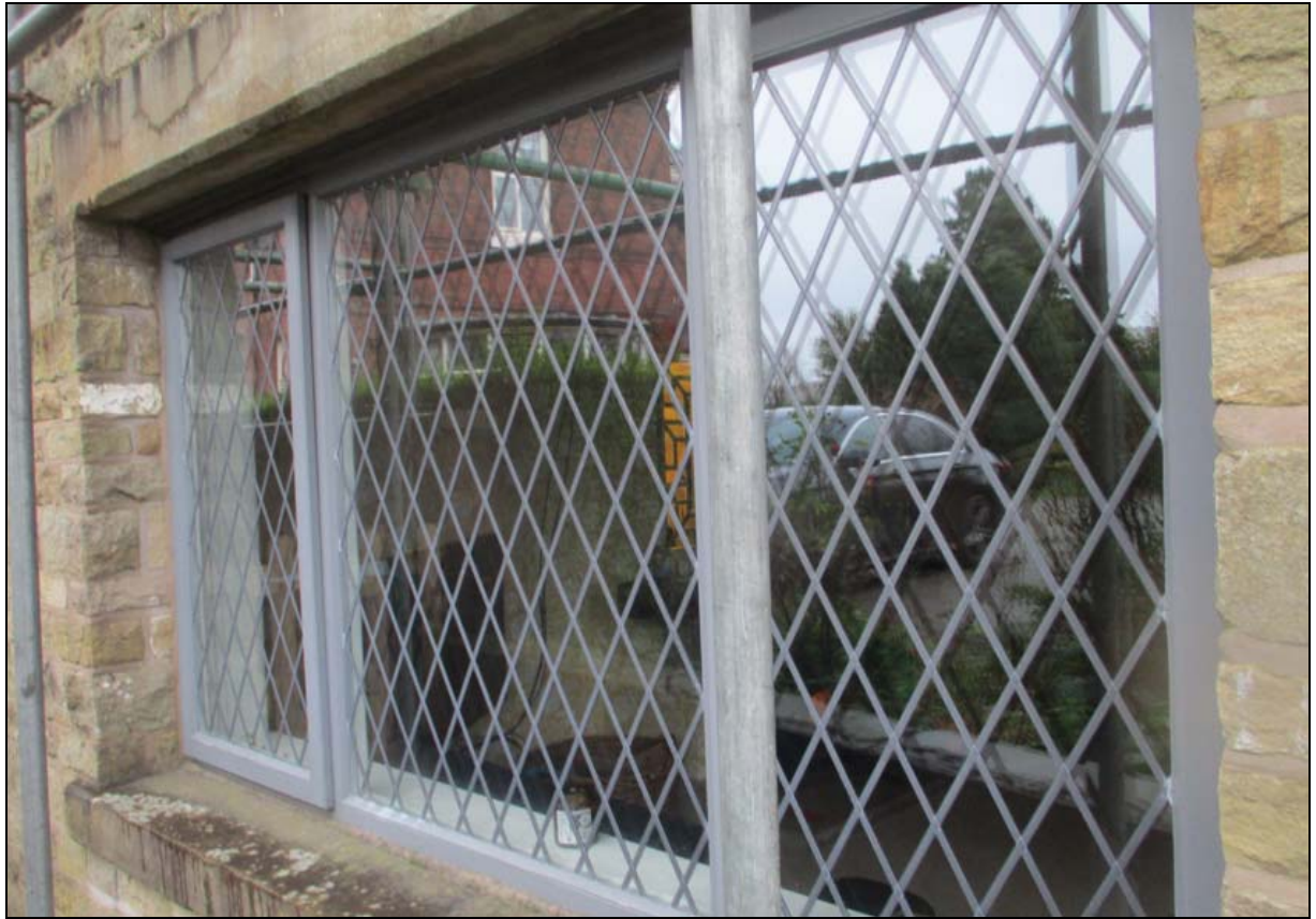
All windows in the wing are modern
