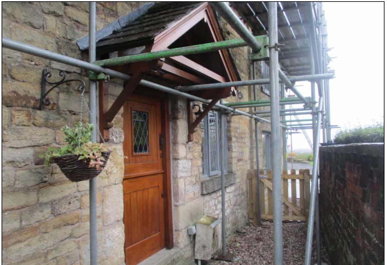
Modern door and canopy on west elevation of the wing
