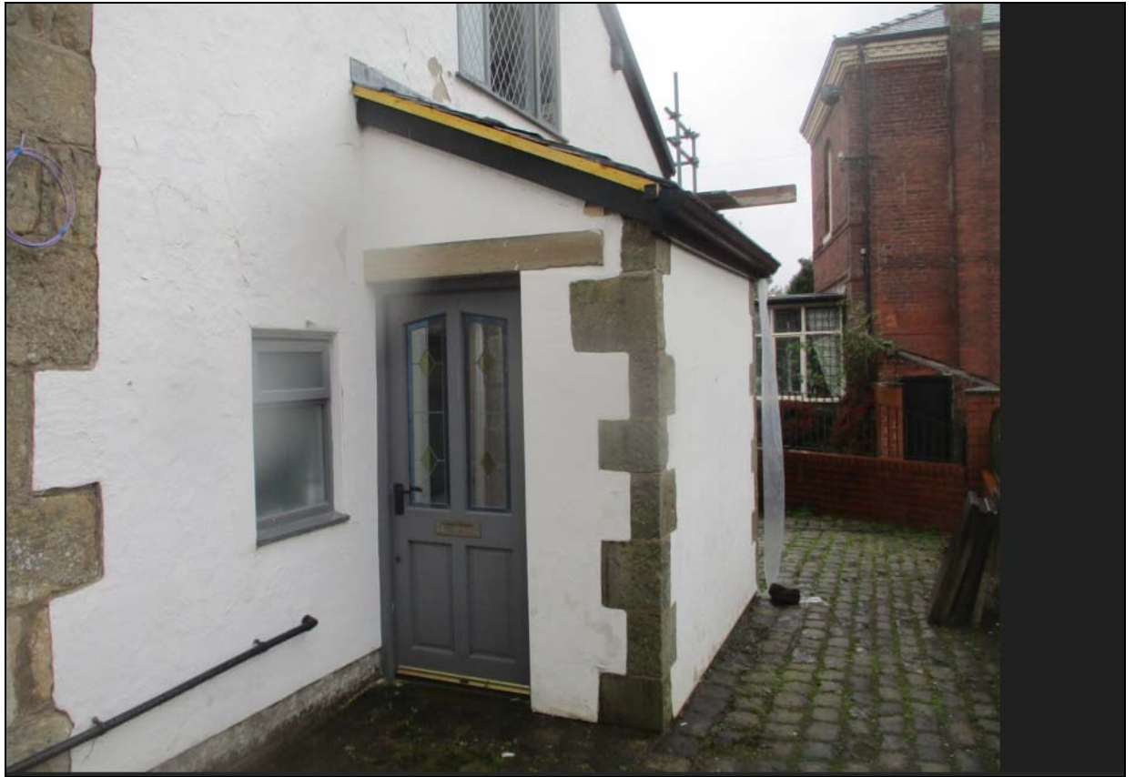
Modern porch on rear elevation of the wing
