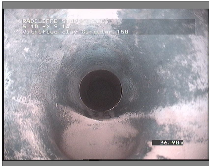
Photo: 8_8_39_A.JPG 36.9m, Finish node type, manhole reference number: S 14
