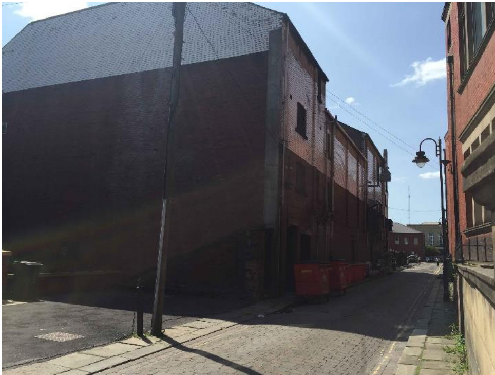
The back of The Art Picture House, from the corner of Moss Street and Back Knowsley Street.
