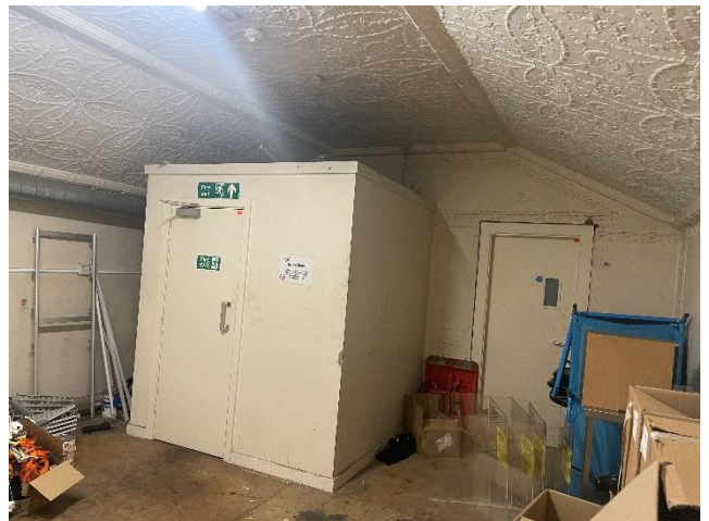
The undeveloped space which will become the staff WC and changing area.
