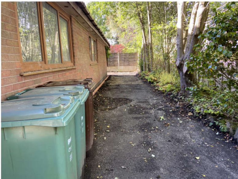
Looking Northwest along Northeast Boundary
