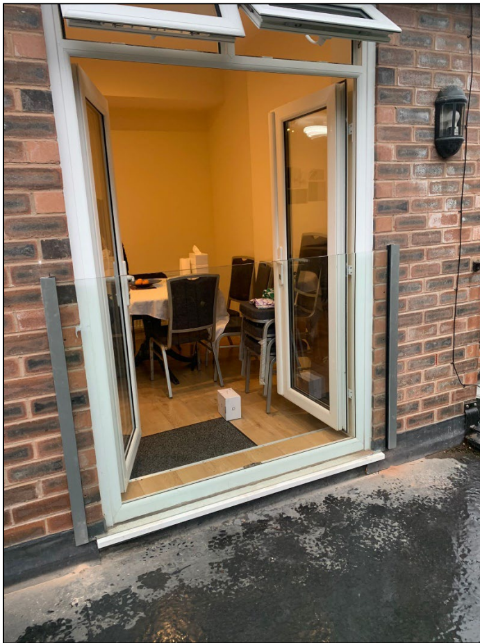
Photograph showing recently installed glass balustrade Juliet Balcony
