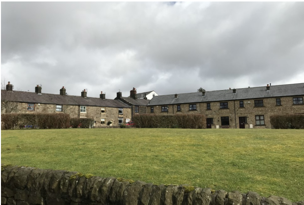
Figure 33: View across the former reservoir to the listed 13-28 Mount Pleasant and the 1980s residential infill.
