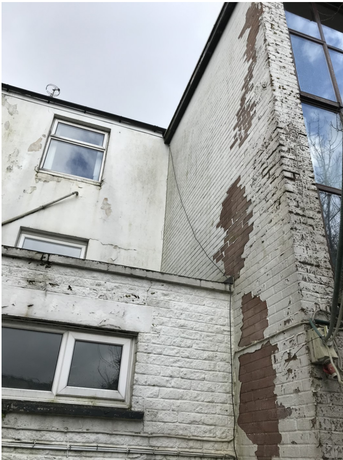
Figure 20: Rear staircase extension to Lord Raglan Public House
