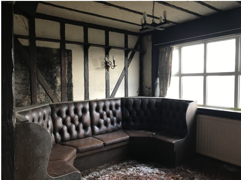
Figure 21: Ground floor of Lord Raglan Public House
