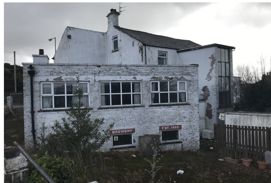
Figure 2: Western (rear) elevation of Lord Raglan Public House
