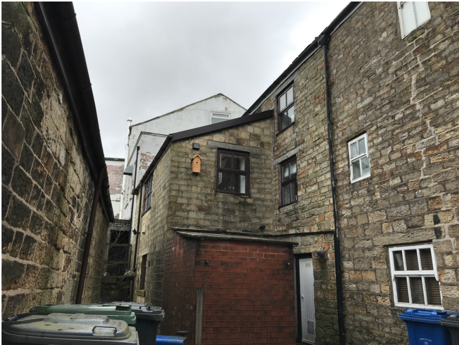
Figure 22: Rear of numbers 11 and 12 Mount Pleasant with southern elevation of Lord Raglan Public House in the background.
