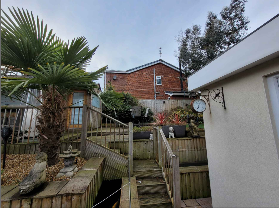
Gable wall number 25 Hackford Close
