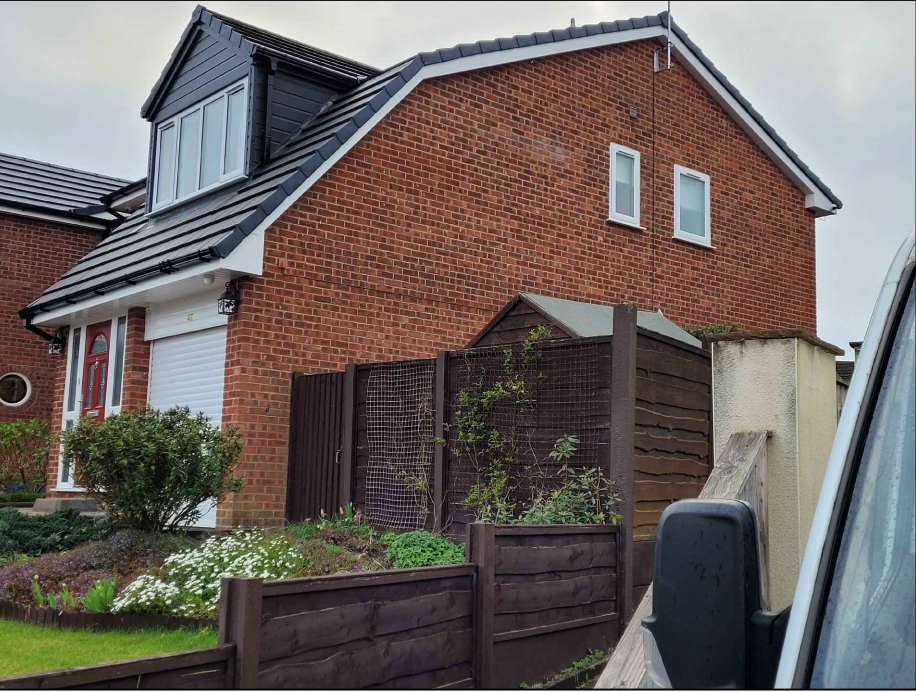
Gable wall number 47 Grantham Drive
