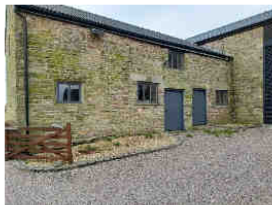
Photograph 2: View of building in centre of site.
