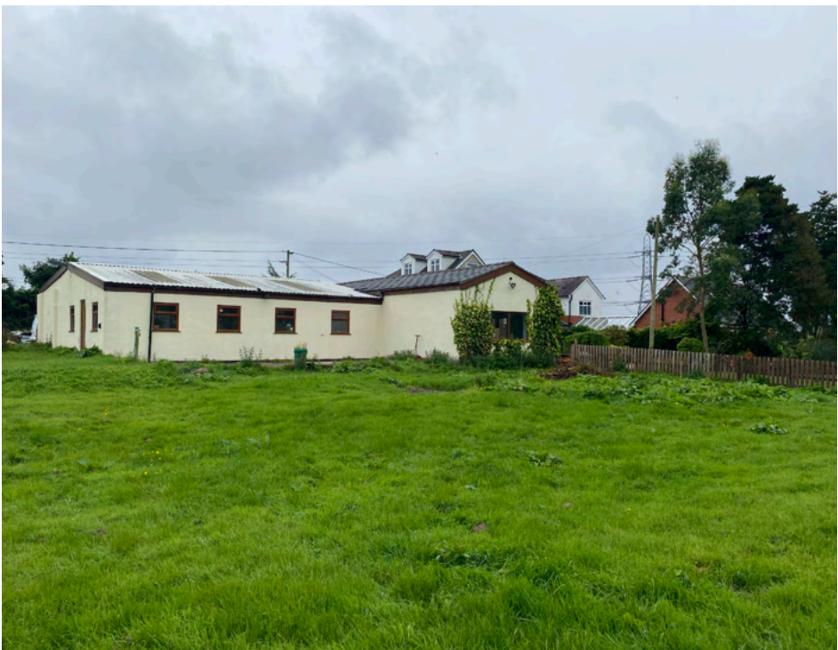
North elevation of existing building
