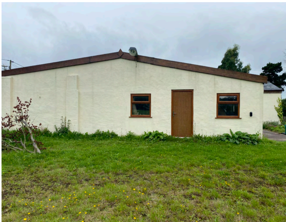
East elevation of existing building
