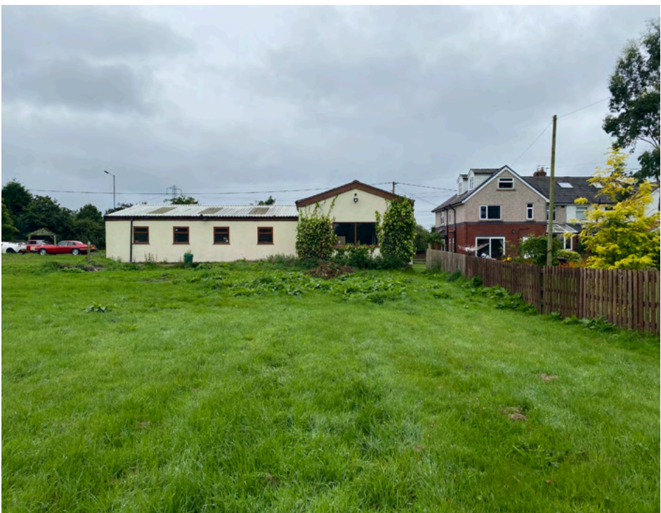
North elevation of existing building adjacent to No.41 Bury Old Road
