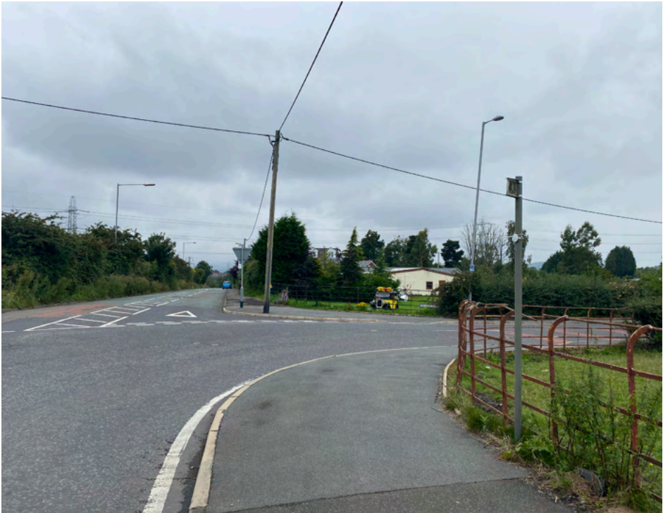
Junction off Bury Old Road leading to Arthur Lane looking East
