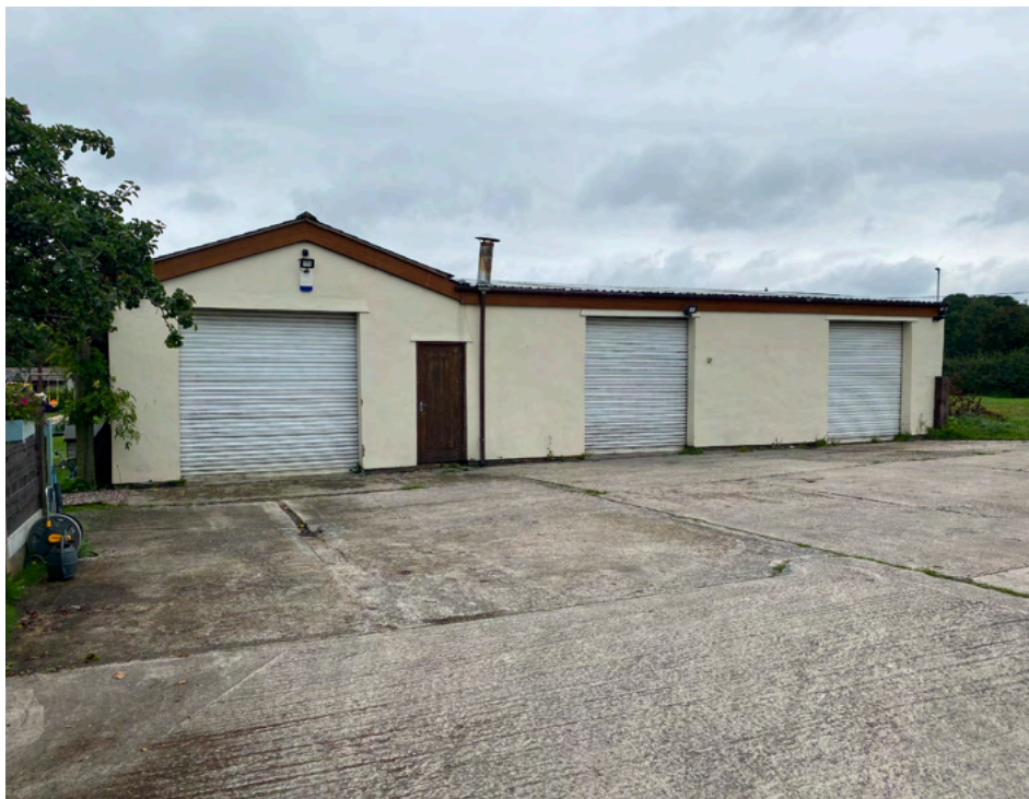
Front elevation of existing building
