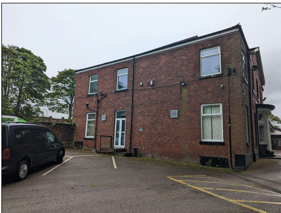
Plate 10: West elevation of Hall
