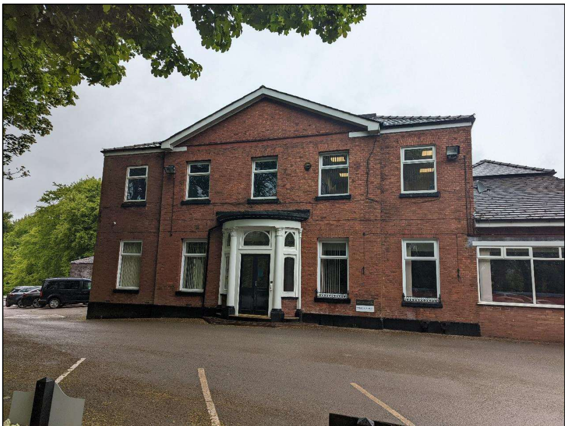
Plate 6: South elevation of Unsworth Hall
