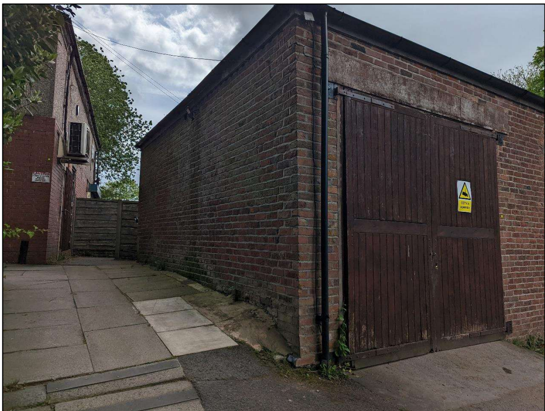
Plate 16: As above from the east
