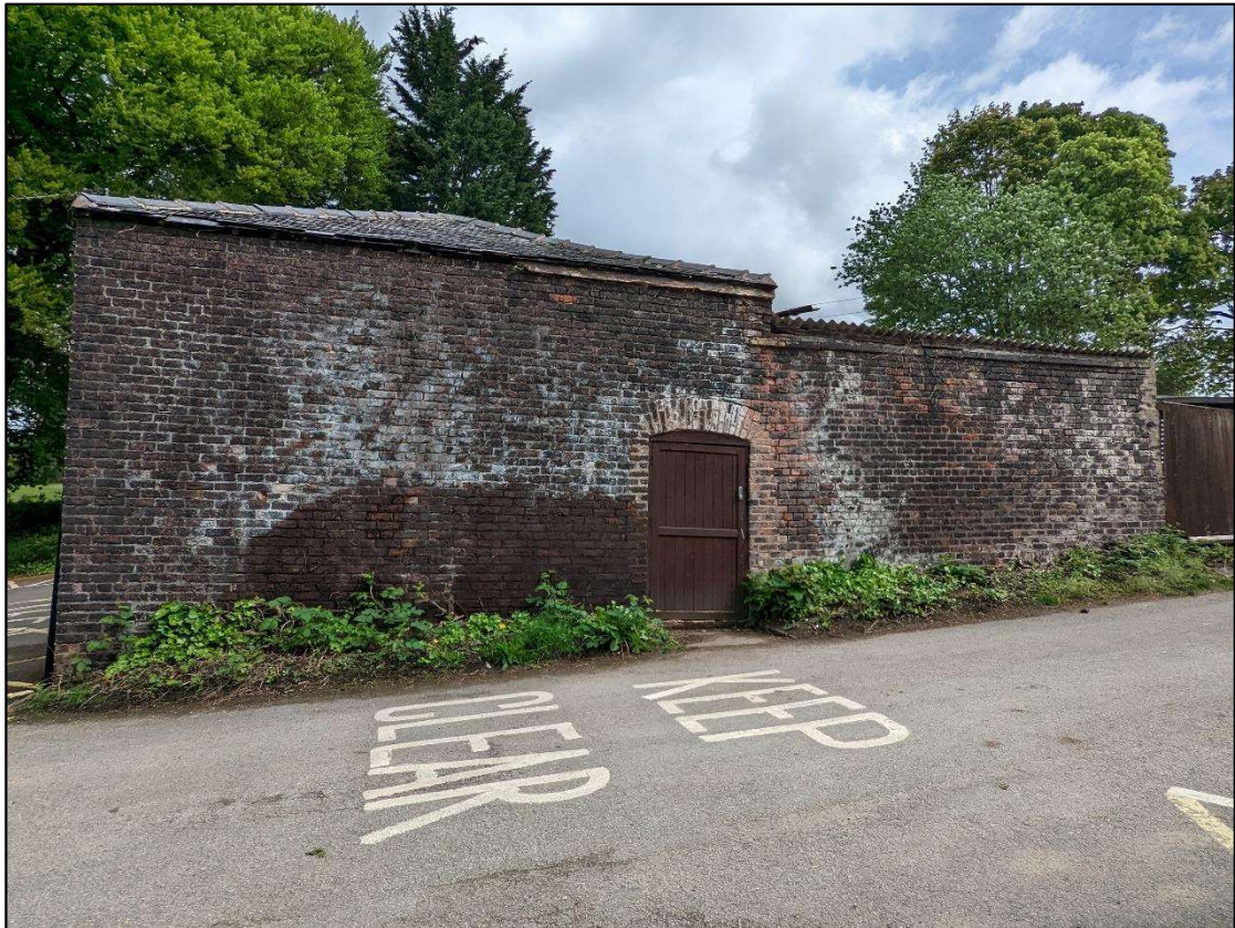
Plate 13: South elevation of attached carriage house and attached garage proposed to be removed
