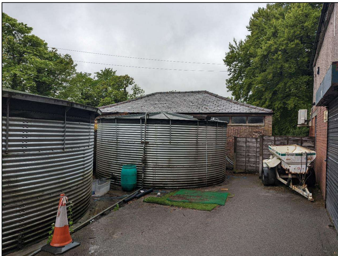
Plate 3: Site showing large water tanks
