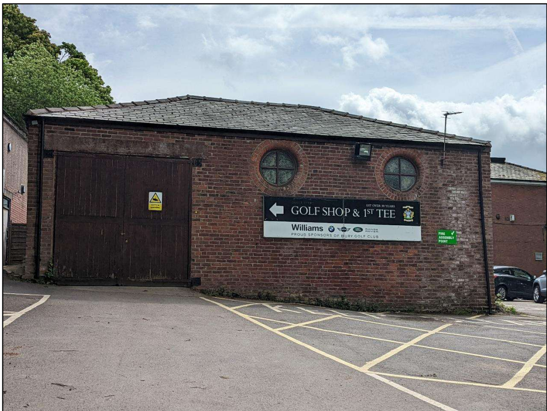
Plate 12: East elevation of carriage house
