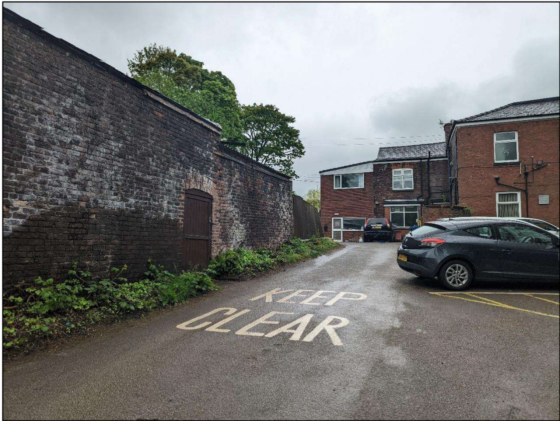
Plate 5: Southern side of site showing carriage house and attached garage
