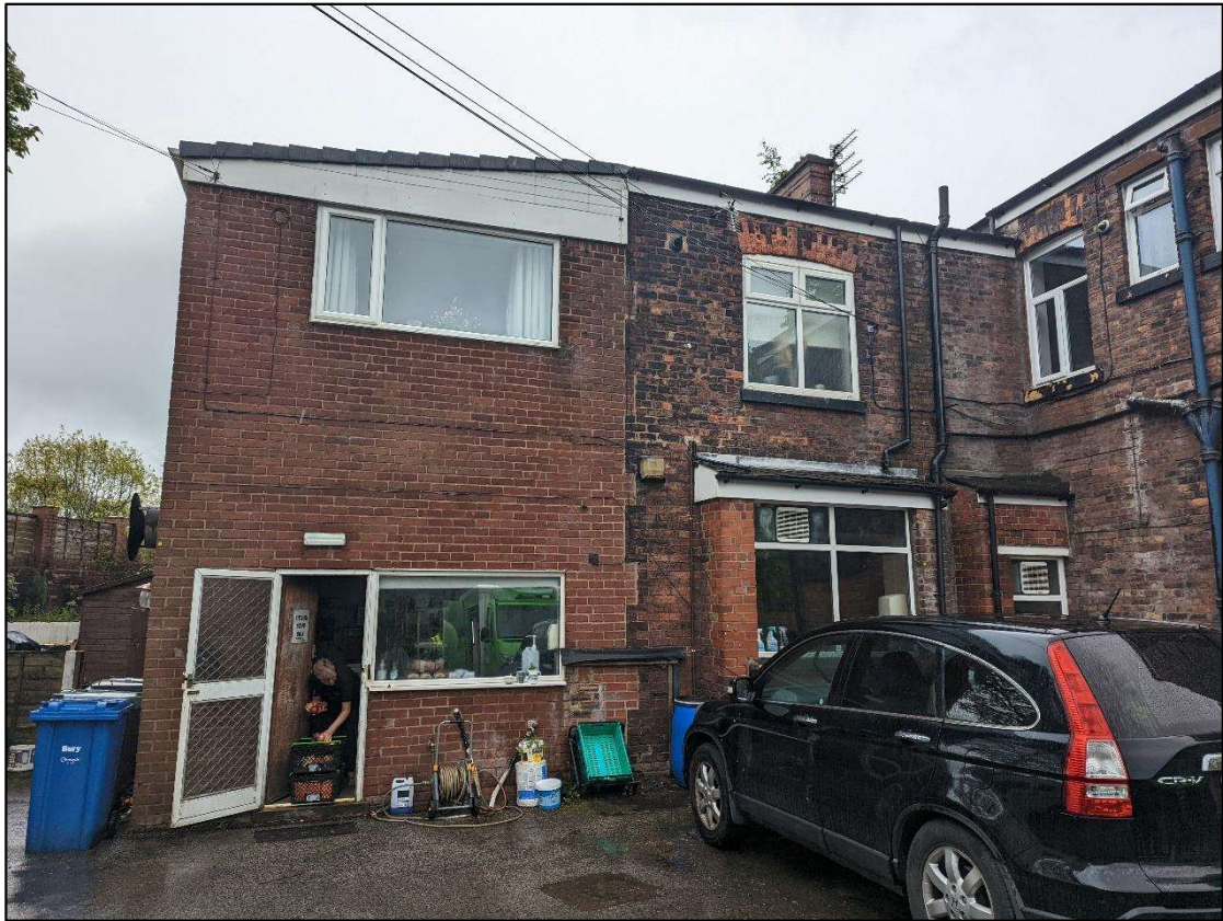
Plate 11: Northern extensions showing early 19 th century extension (right), with modern unsympathetic extension attached (left)
