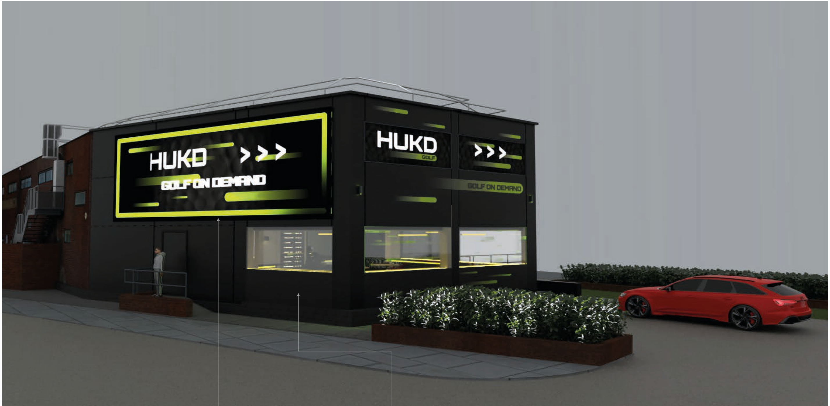
Facade of building clad in new matt Black Dibond panels with crushed edge construction
