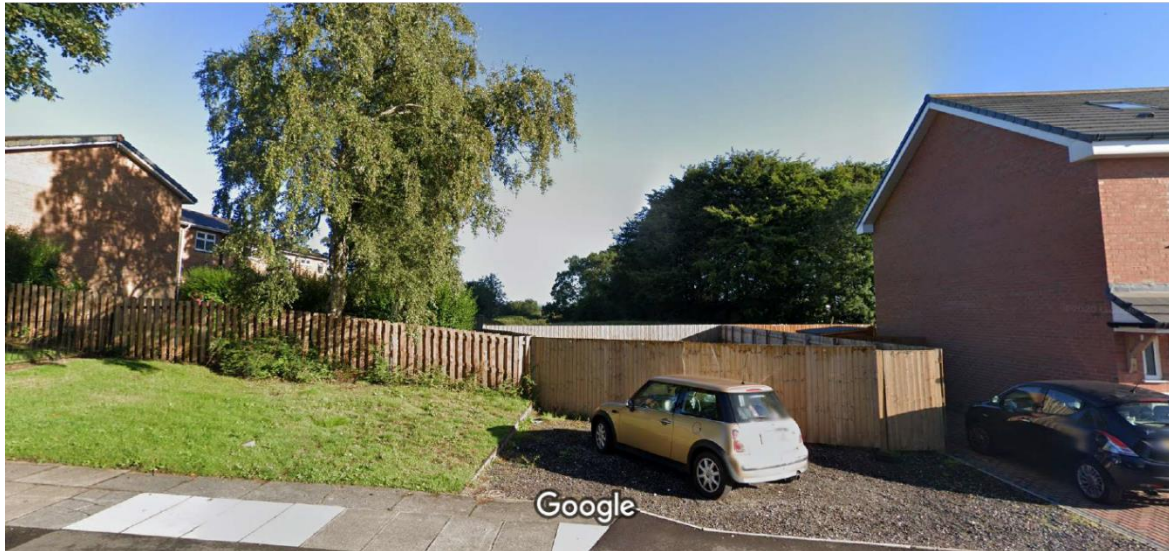
Fig 3 Existing Site Photo (extracted from google street view)
