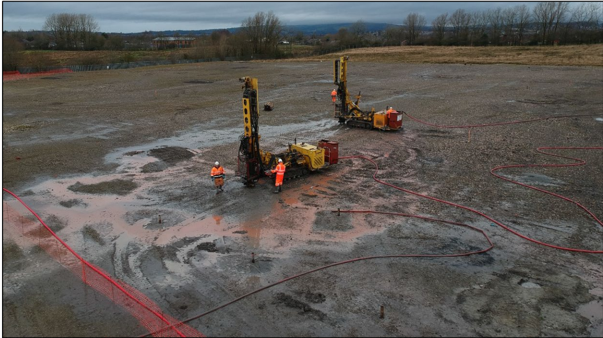
Rotary drilling rigs undertaking drilling in the northern site section in February 2025.
