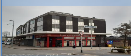
The three-storey building viewed from the south-west
