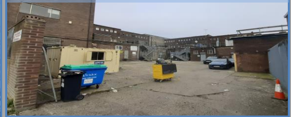
The open, service yard at the rear of the three-storey building
