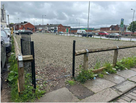
Photograph of the new pedestrian access for the car park
