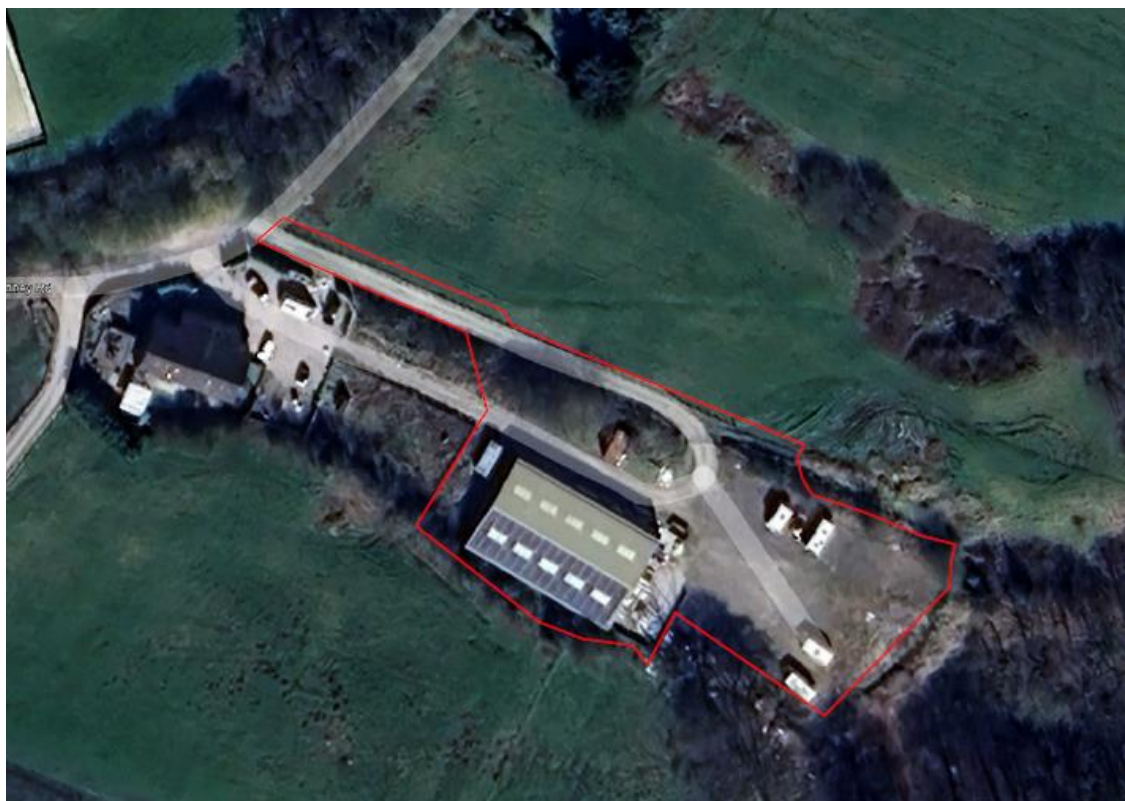
Figure 1.1: Abbots Hall, Woodhey Road, Holcombe Brook.
