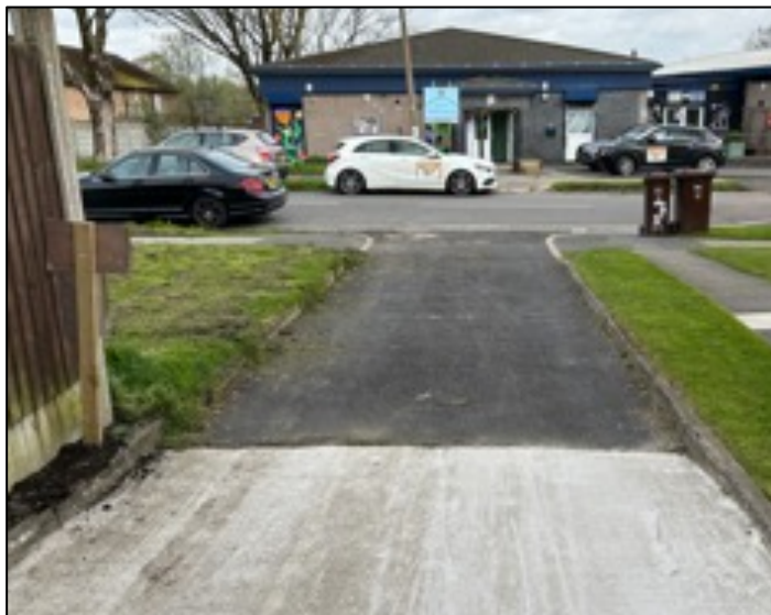
Tarmac surfaced access to garage site with concrete edgings
