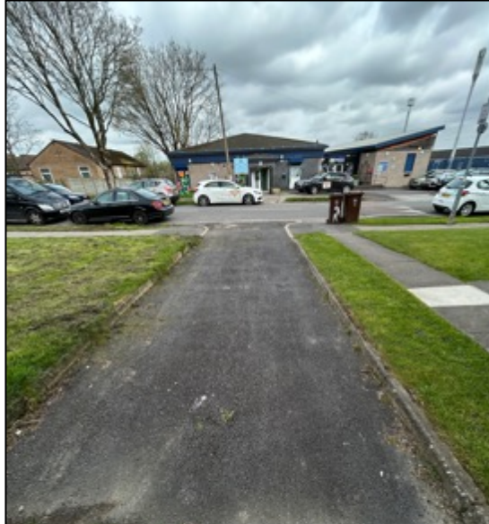
Tarmac surfaced access to garage site with concrete edgings
