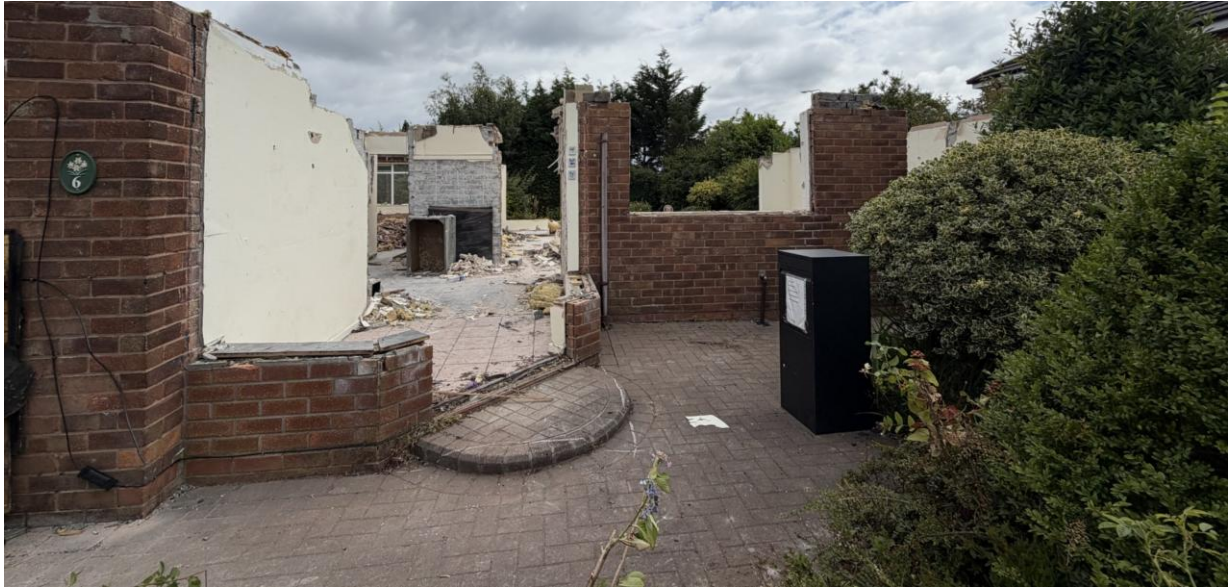
Figure 4: Partially demolished dwelling photograph
