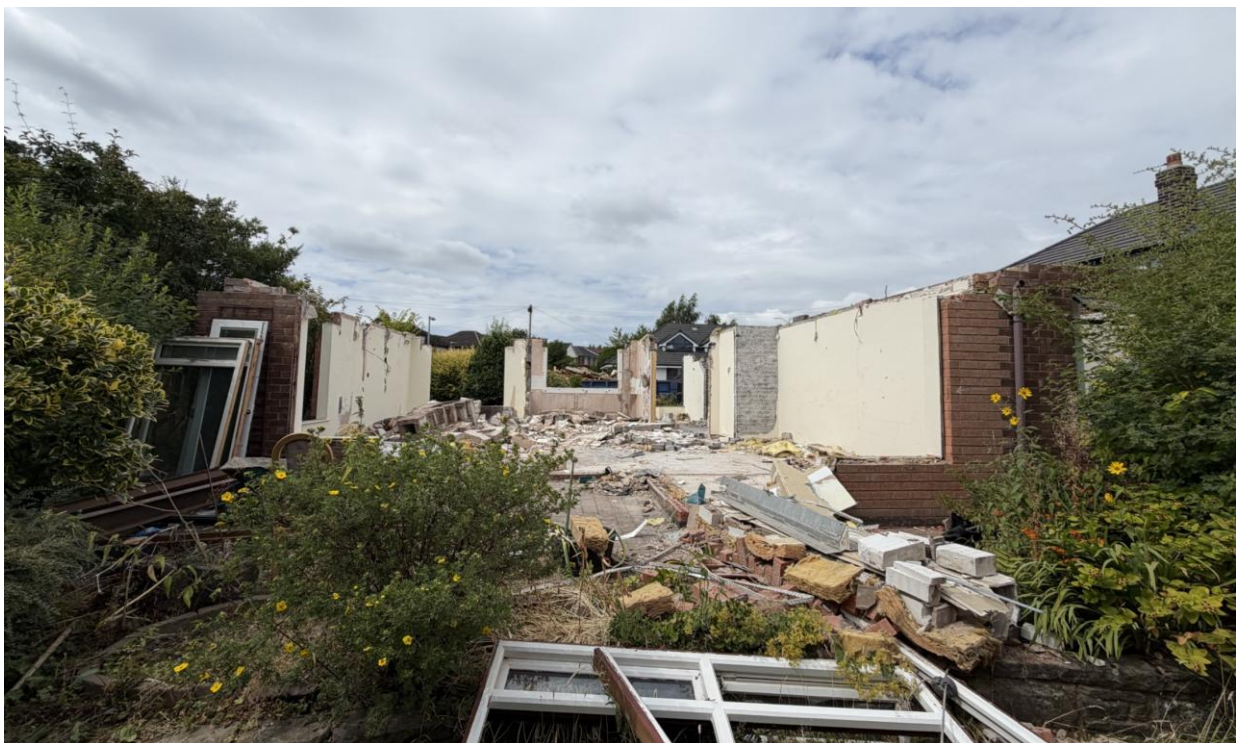
Figure 5: Partially demolished dwelling photograph
