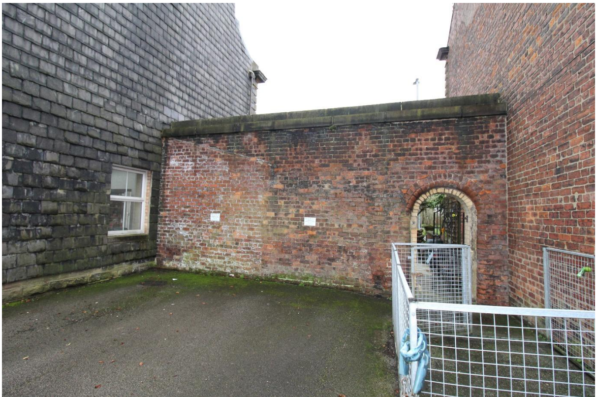
Plate 8 – Side Wall, Rear Elevation
