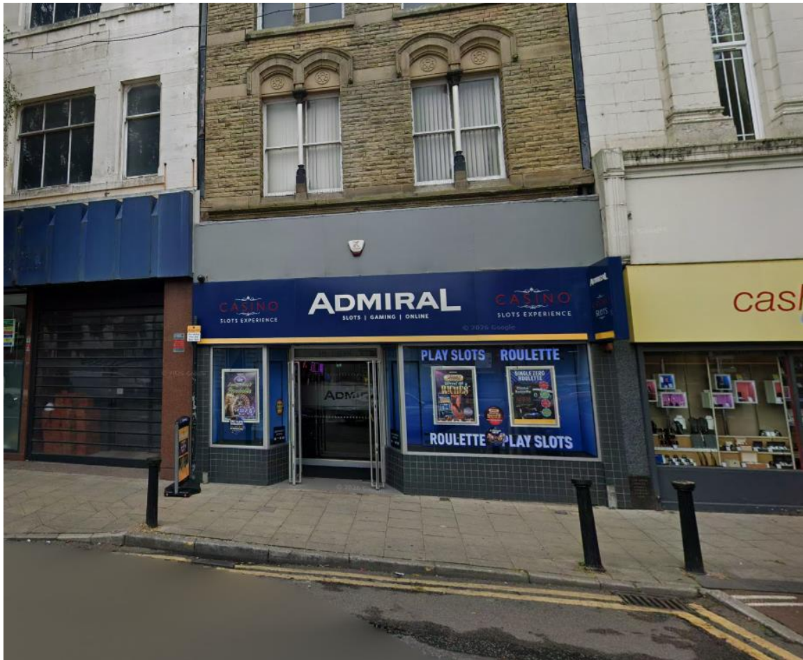
Existing Satin Anodised Aluminium Shopfront
