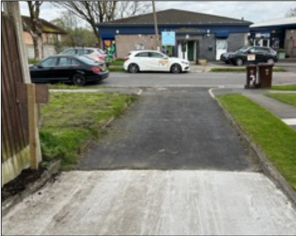
Tarmac surfaced access to garage site with concrete edgings
