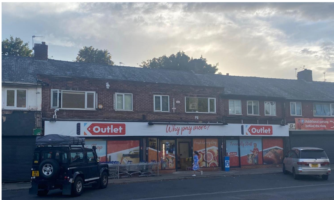
Image 1: The site as viewed from Bury Old Road currently trading as K-Outlet
