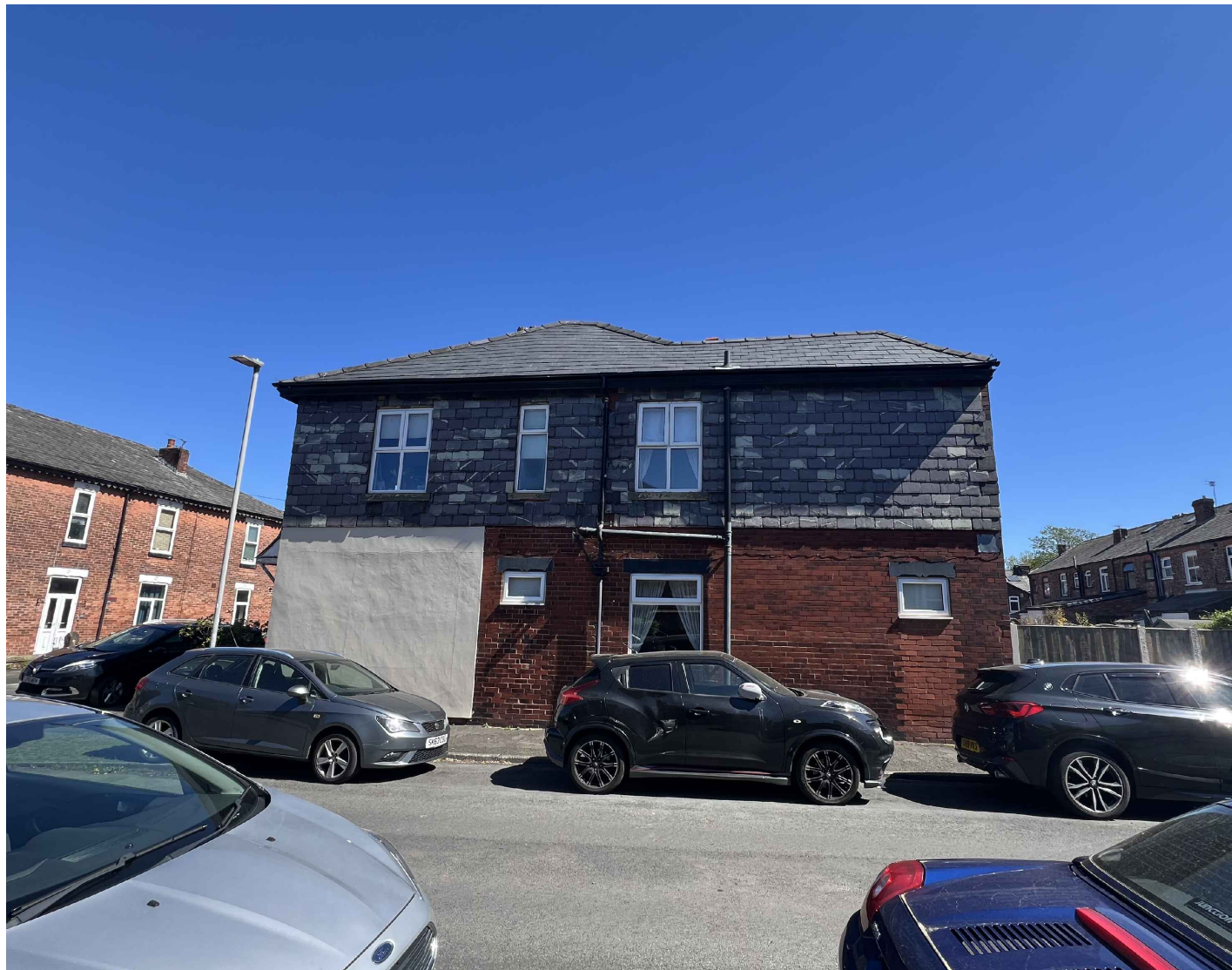
Side Elevation of Site
