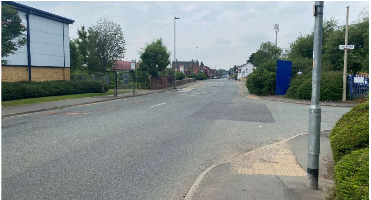
Photograph 2.3 : Access Road / Dumers Lane Junction (westbound)
