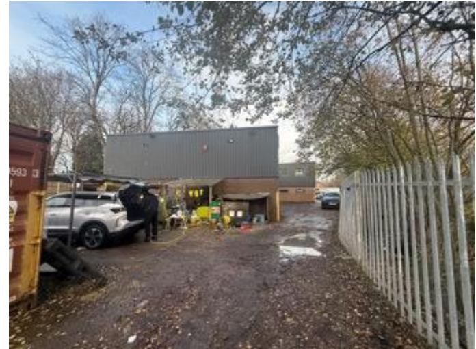
Southern elevation of B1
