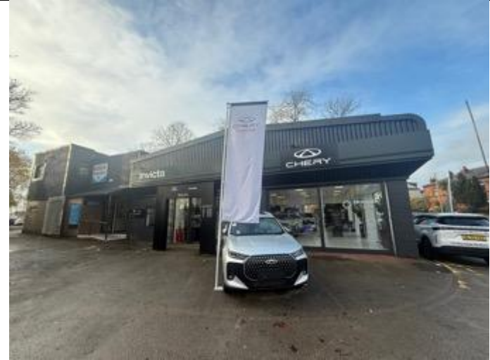
Western elevation of B1
