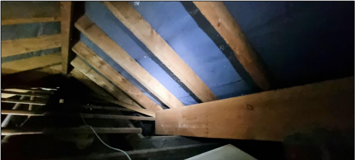
Plate 14: The membrane was generally intact with no gaps apparent. No evidence of bats were present behind them.
