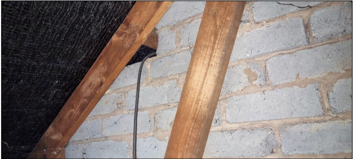
Plate 17: Locations such as the top of the gable walls offered roosting potential but no signs of bats were present.
