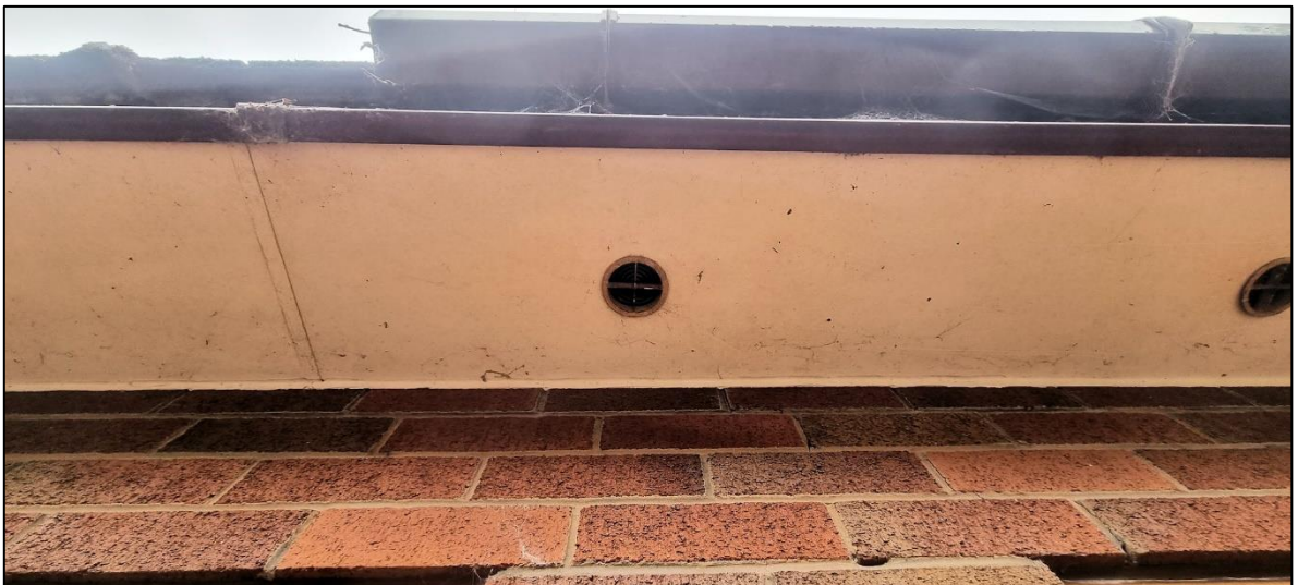
Plate 8: The soffits were generally tightly sealed with no gaps.
