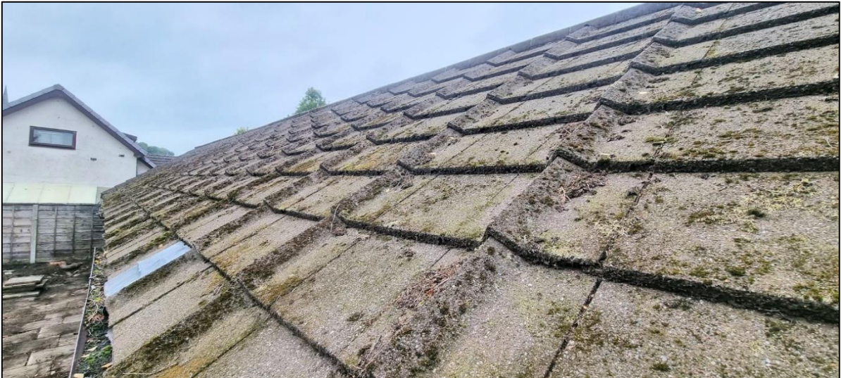
Plate 4: The roof pitches were intact with no slipped or missing tiles and offered roosting opportunities.
