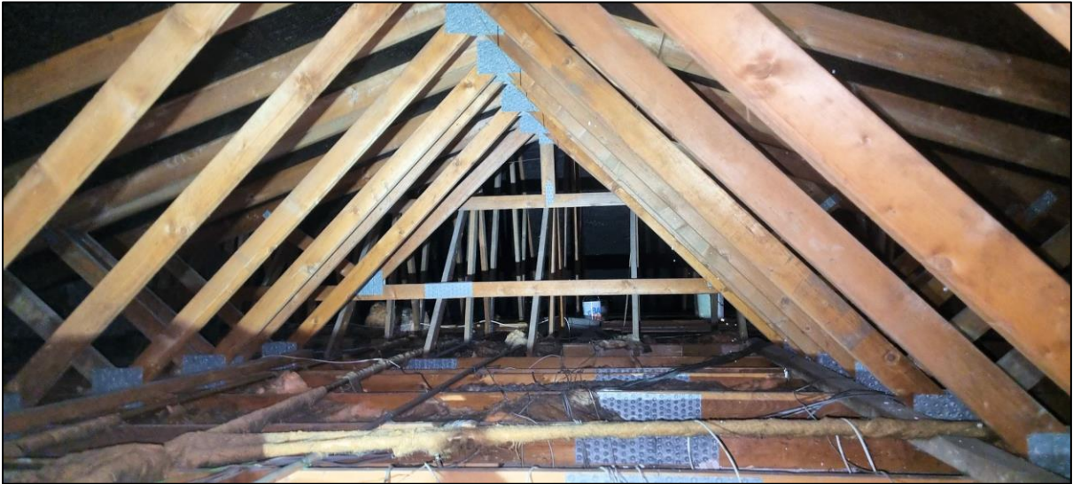
Plate 13: The loft void was open to the roof roofing timbers and the roofing membranes.
