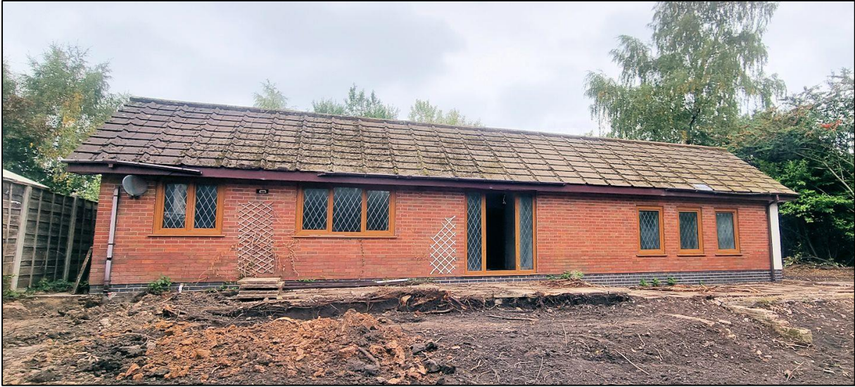
Plate 1: General view of the residential property from the south.
