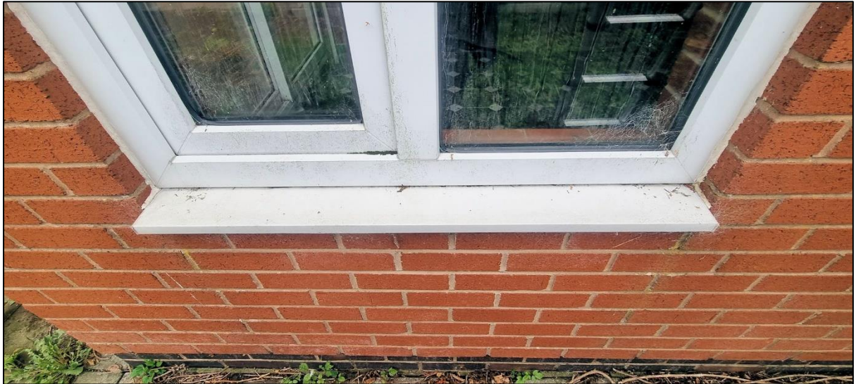
Plate 12: There was no evidence of bat activity on the walls or flat surfaces around the building.
