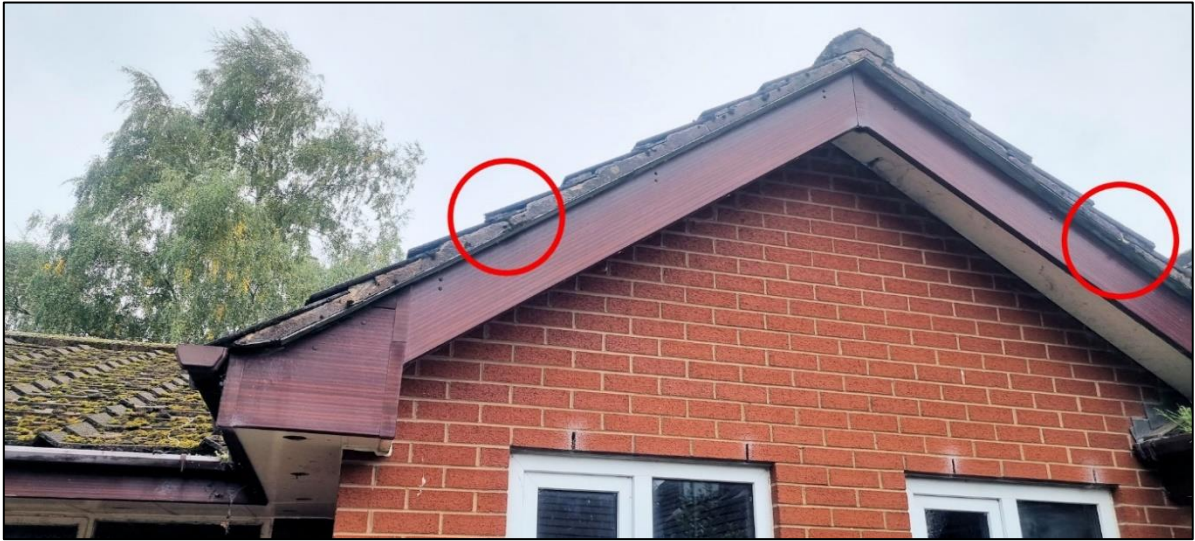
Plate 5: Gaps were noted in the mortar of the verges which were inspected more closely to see if they offered opportunities.
