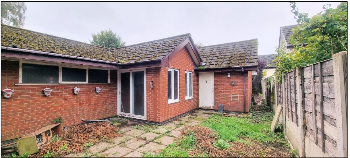
Plate 2: General view of the detached residential bungalow from the rear.
