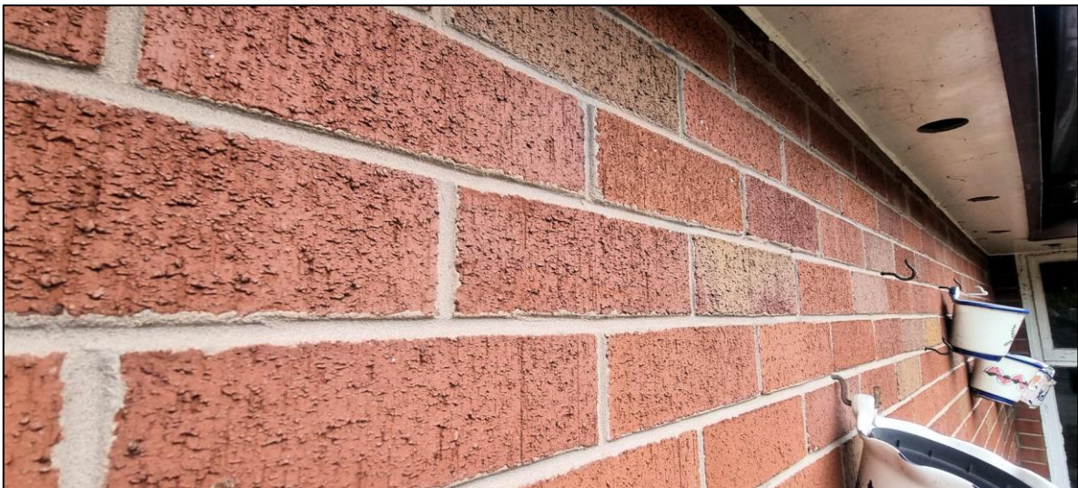
Plate 10: The external walls were in good condition with no gaps in the brickwork or the render.
