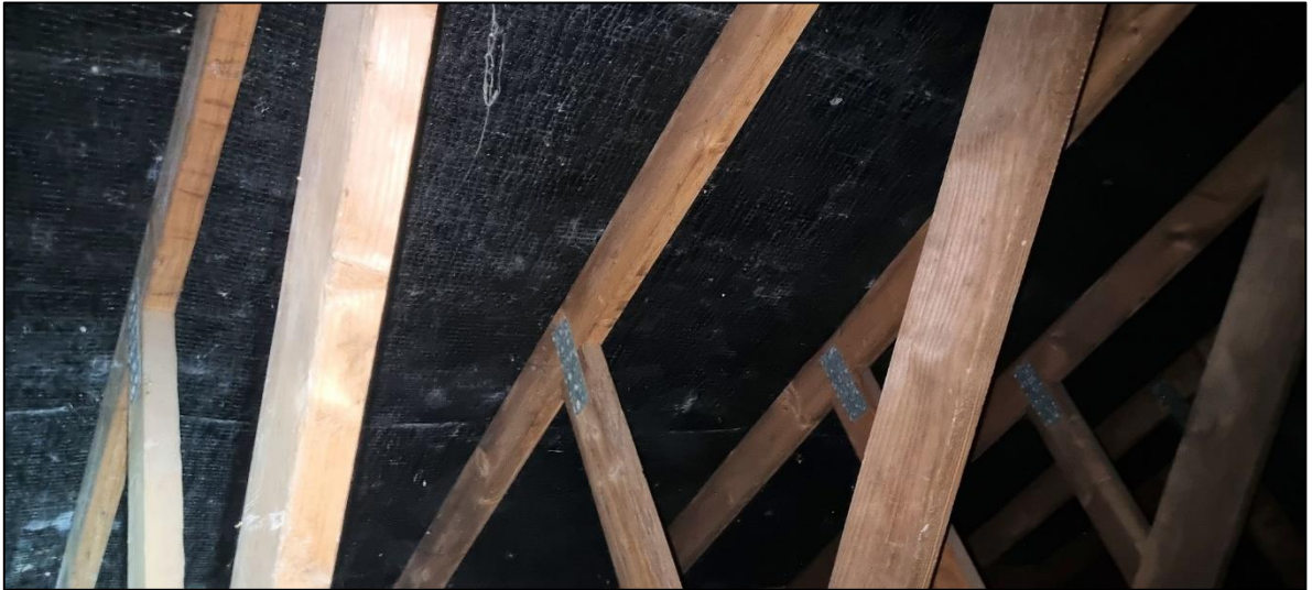
Plate 15: The older felt membrane were also generally intact.
