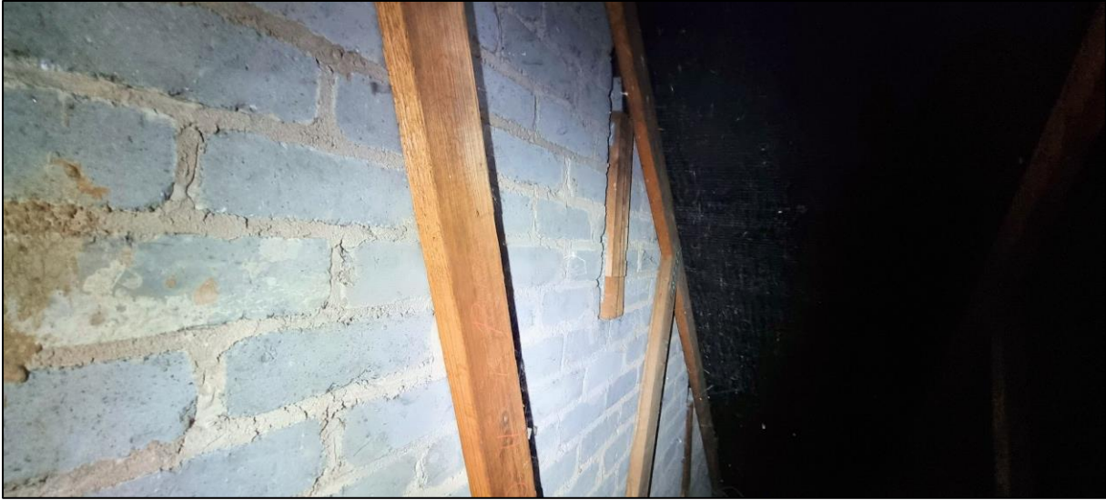
Plate 19: There was no evidence of bat activity on the internal gable walls.
