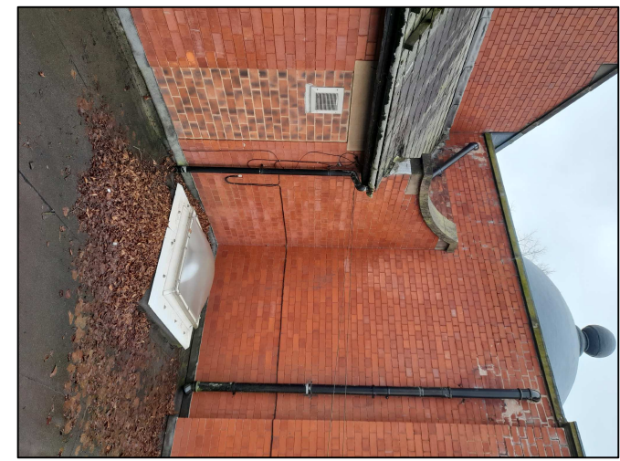
PHOTO 4 Showing wall to dome
