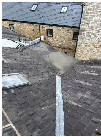
photos showing two existing flat roofs
