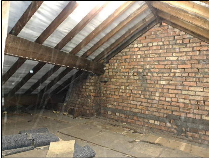
Photograph 5 showing the first roof void
