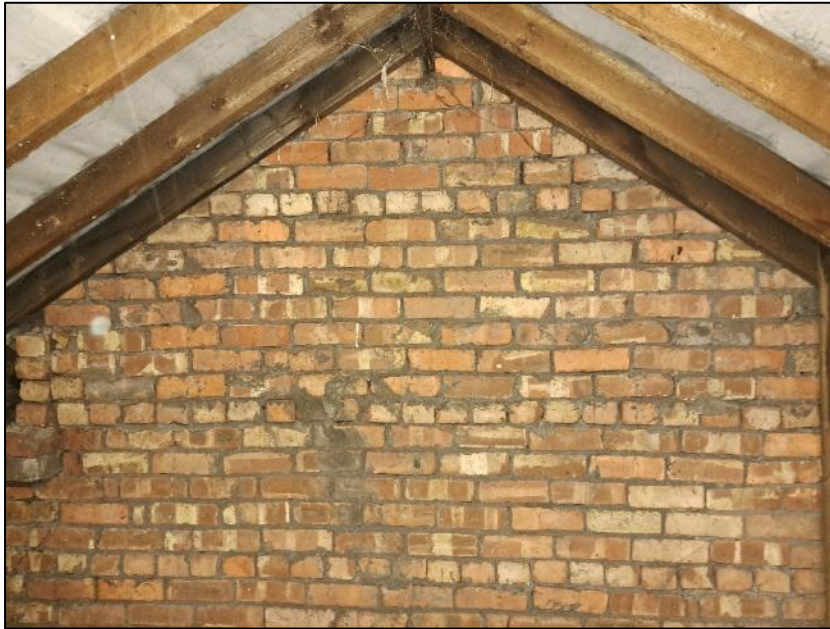
Photograph 7 showing the internal brickwork
