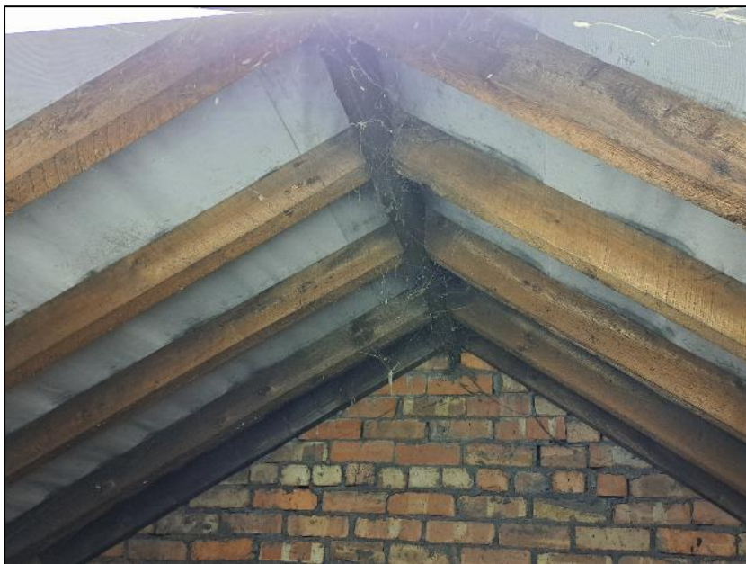
Photograph 6 showing the roof timbers and lining
