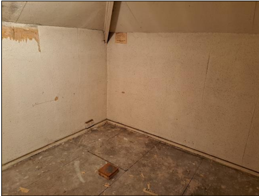
Photograph 9 showing the room within the second roof void
