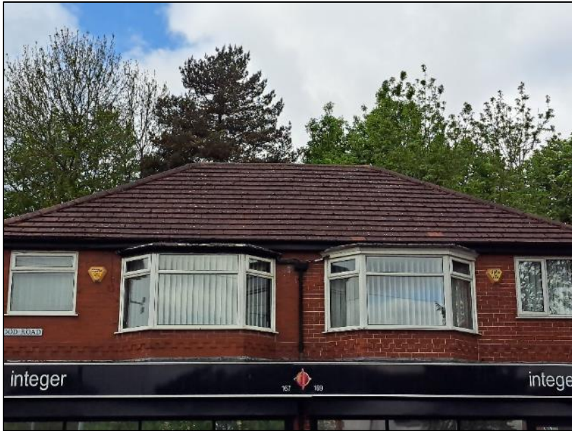
Photograph 3 showing the hipped roof
