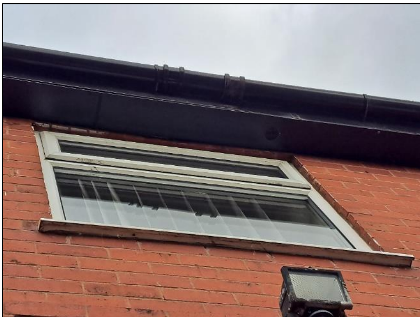
Photograph 4 showing the soffit boxes
