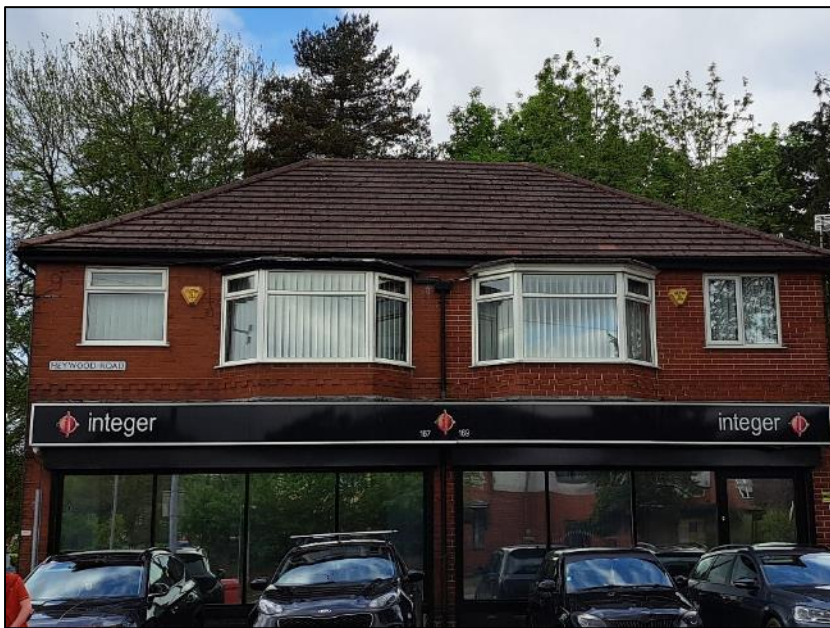
Photograph 2 showing the front elevation
