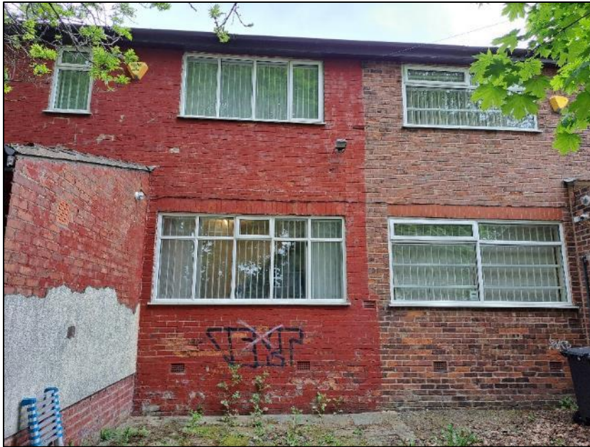
Photograph 1 showing the rear elevation
