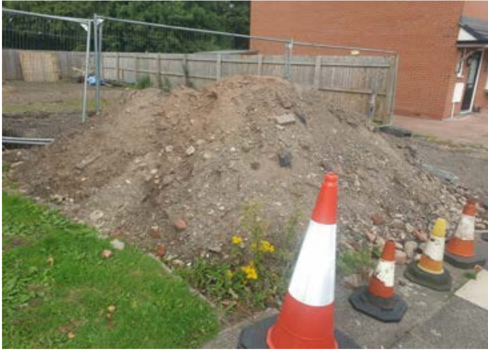
Photograph 5: Site conditions (north easterly facing)
