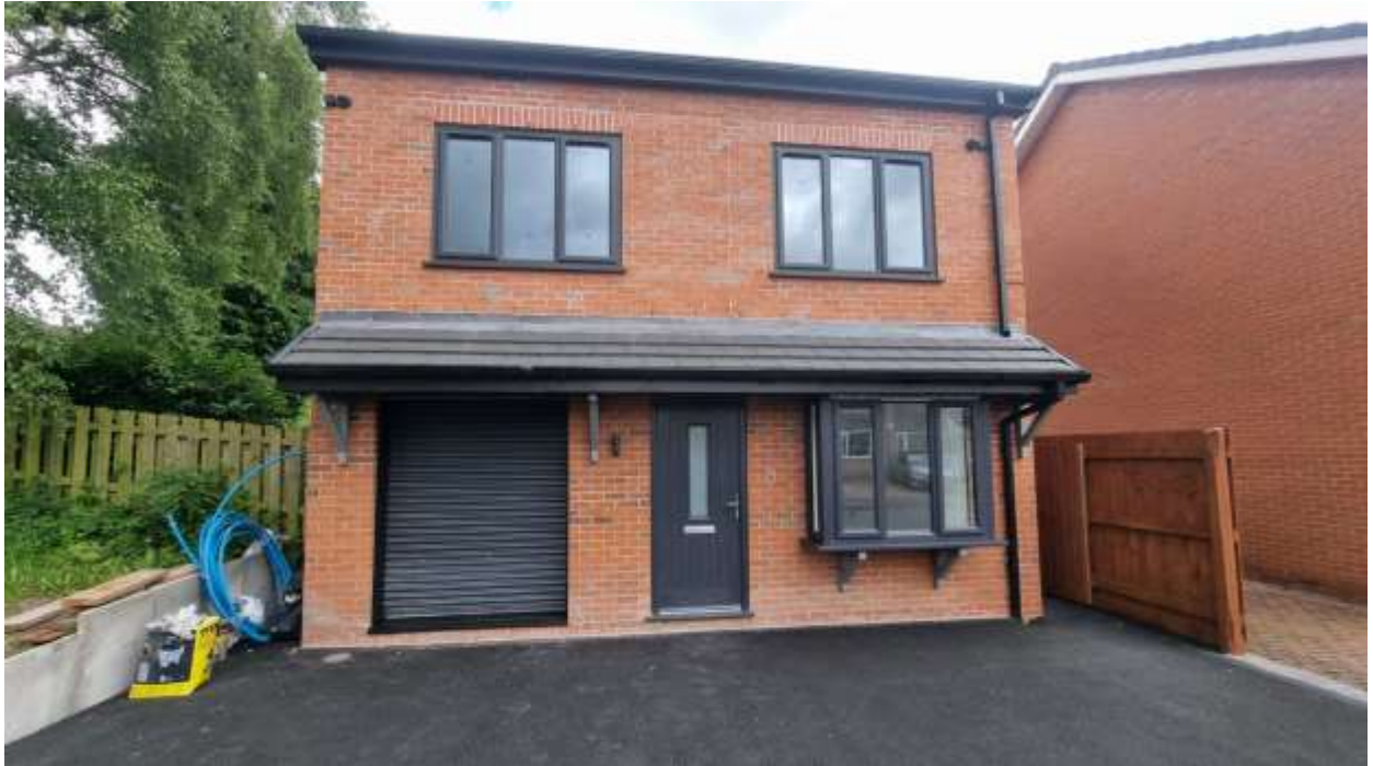
Figure 1, Roller shutter and Footway Crossing
