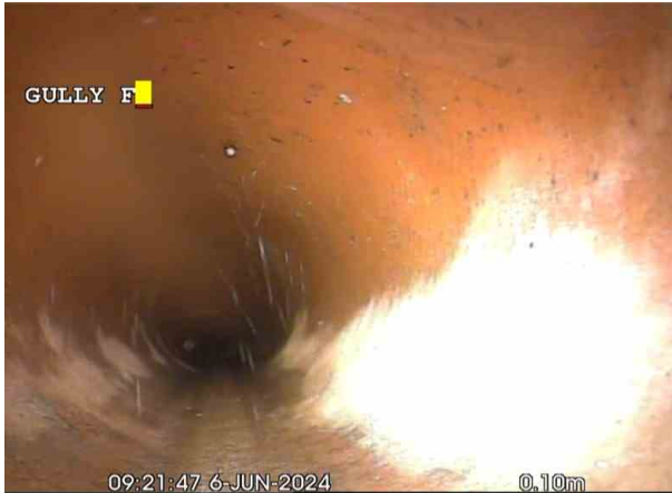
GULLY FX_a2c1a5ab-91a9-4f0b-a5cc-319c8cc1ae6b_20240606_131 009_109.jpg, 00:00:00, 0.00 m General photograph taken at this point
