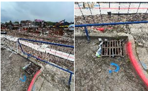
GULLY C AND ITS LOCATION
