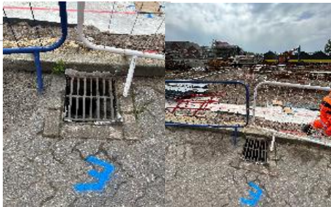
GULLY E AND ITS LOCATION
