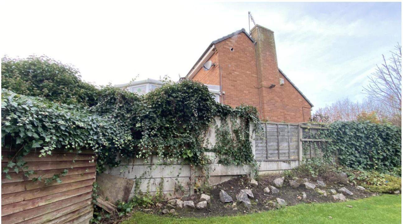
Image 2: View of the side elevation of No. 75 Sheepfoot Lane from the rear of the site facing west
