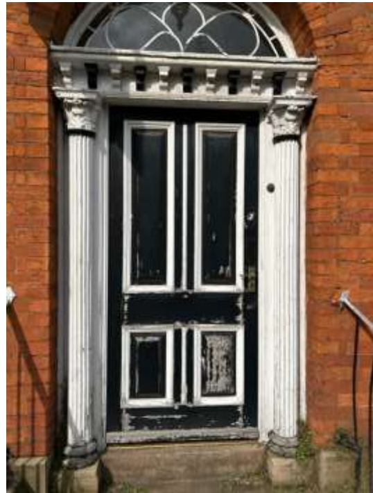
External view of redundant entrance door (D2)
