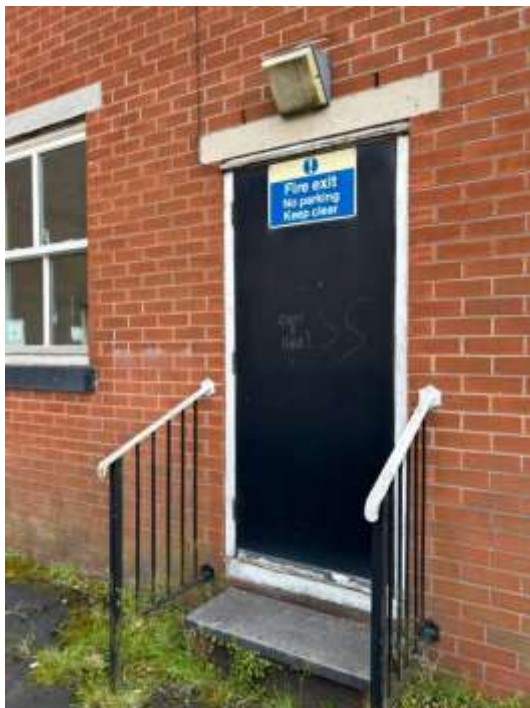
Timber door and frame (D5)
