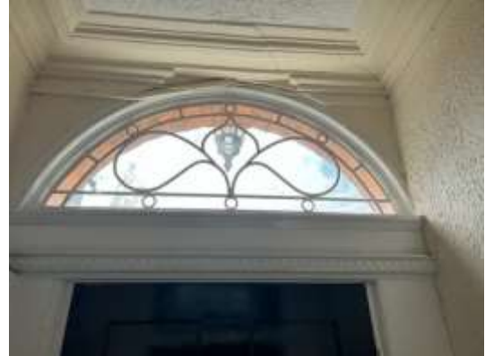
Internal view of fanlight – WT2
