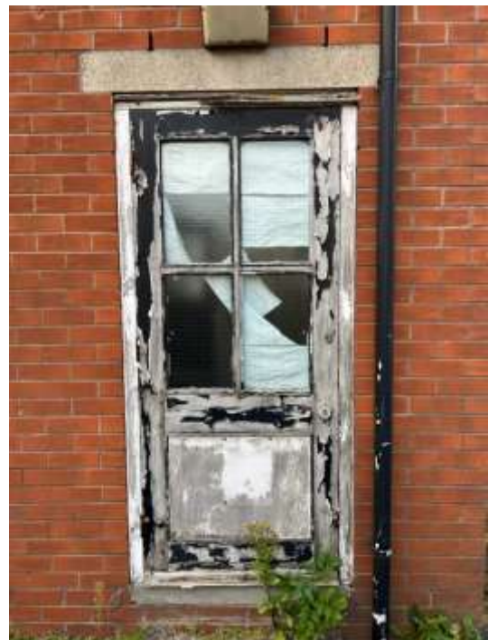
Timber door and frame (D6)
