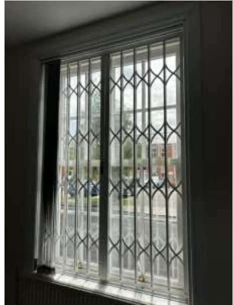
Internal view of Type 1 window – WT1
