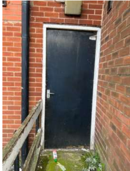
Timber door and frame (D3)
