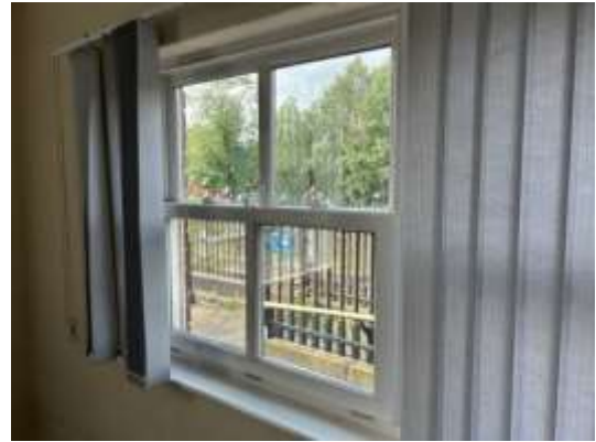
Internal view of Type 3 window – WT3
