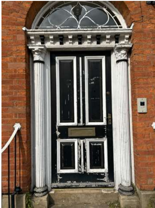
External view of communal entrance door (D1)
