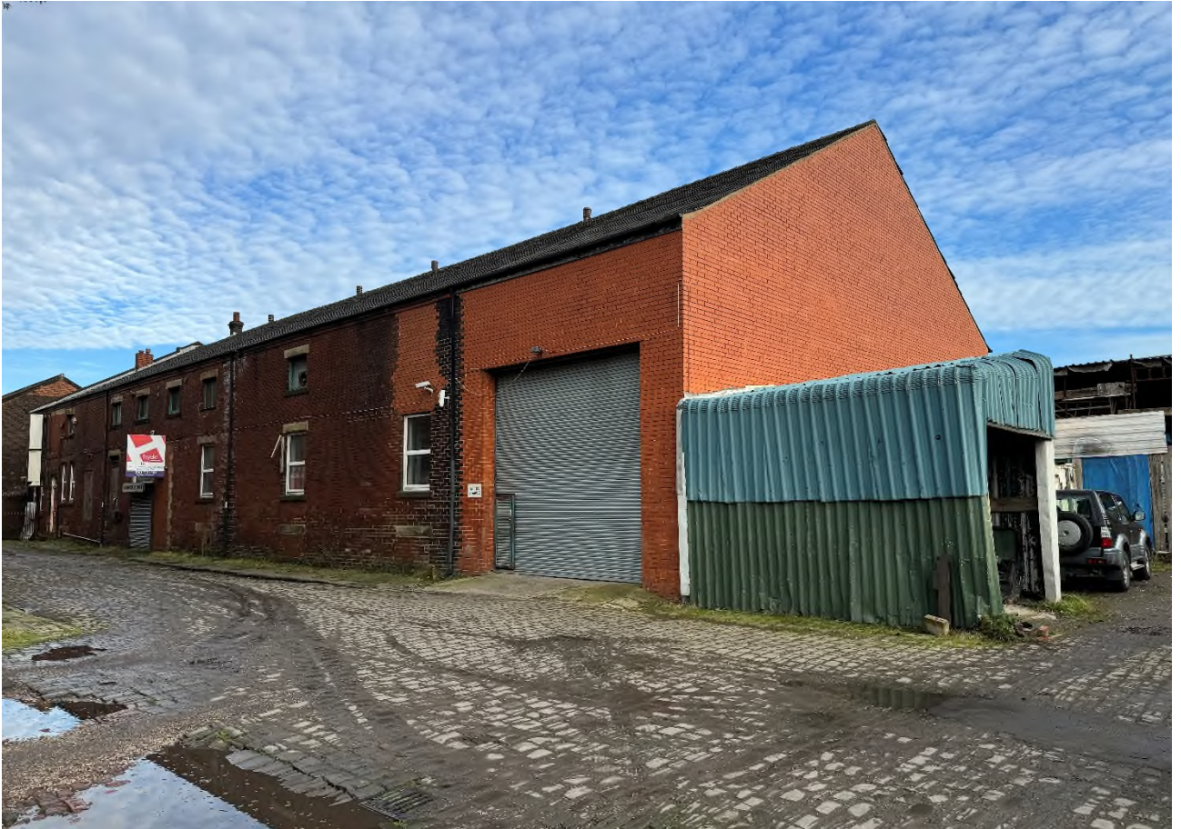
Photograph No 3 - General View of Albion House from the South
