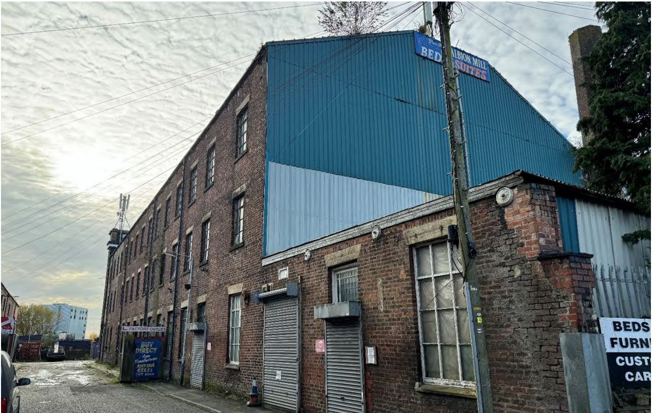
Photograph No 11 - View of Albion Mill from the North
