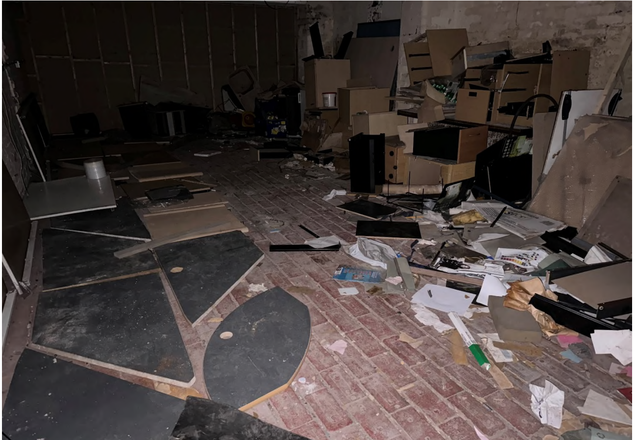
Photograph No 9 - Albion House Semi-Basement
