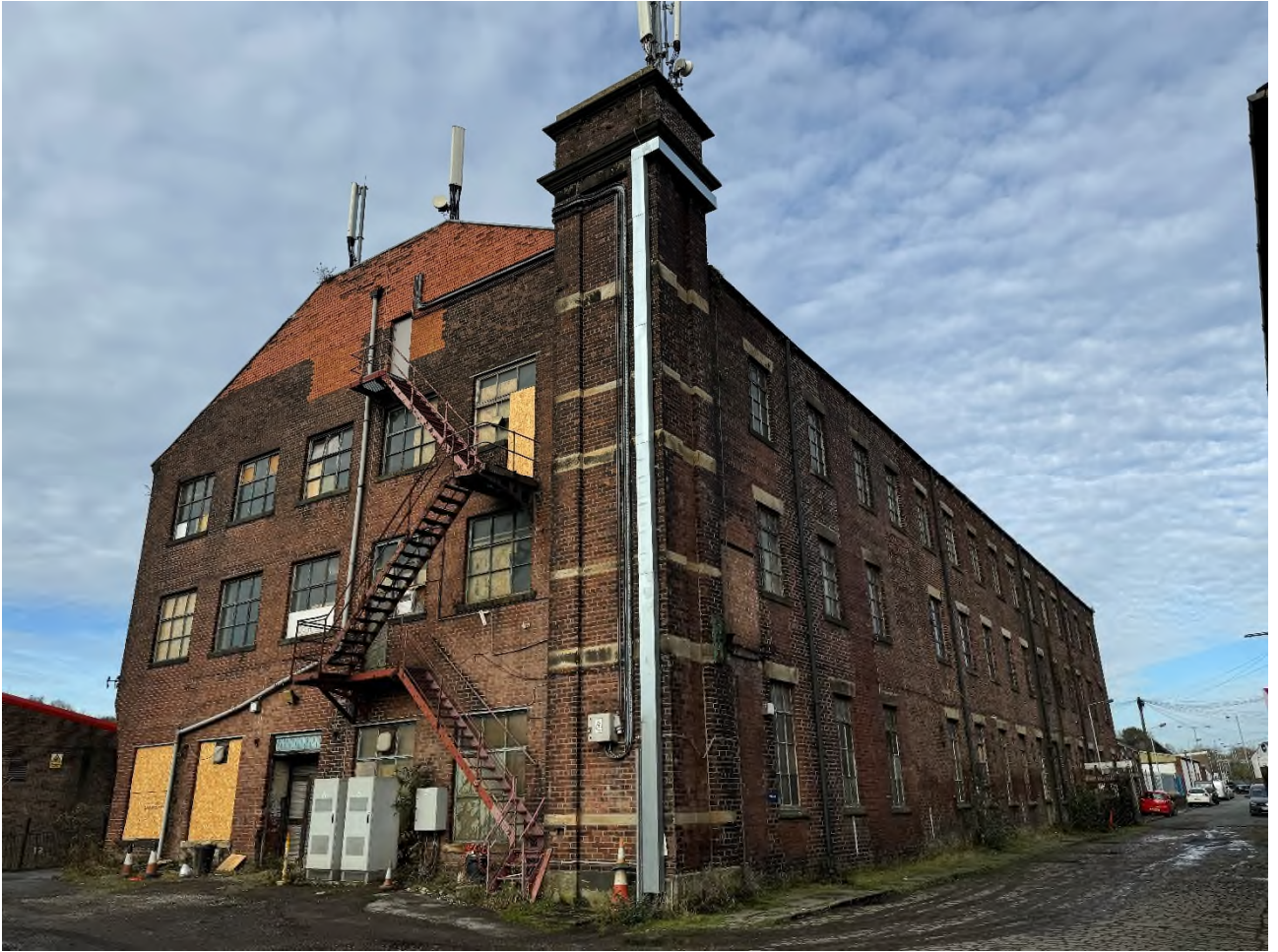
Photograph No 11 - View of Albion Mill from the South
