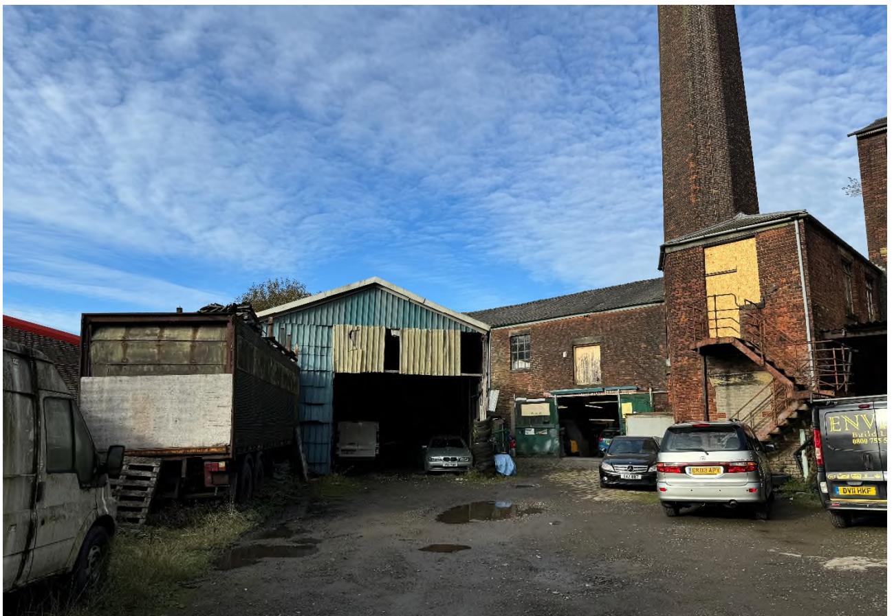
Photograph No 13 - View Towards the Garage
