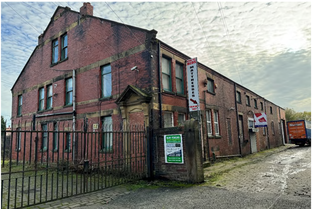
Photograph No 2 - General View of Albion House from the North
