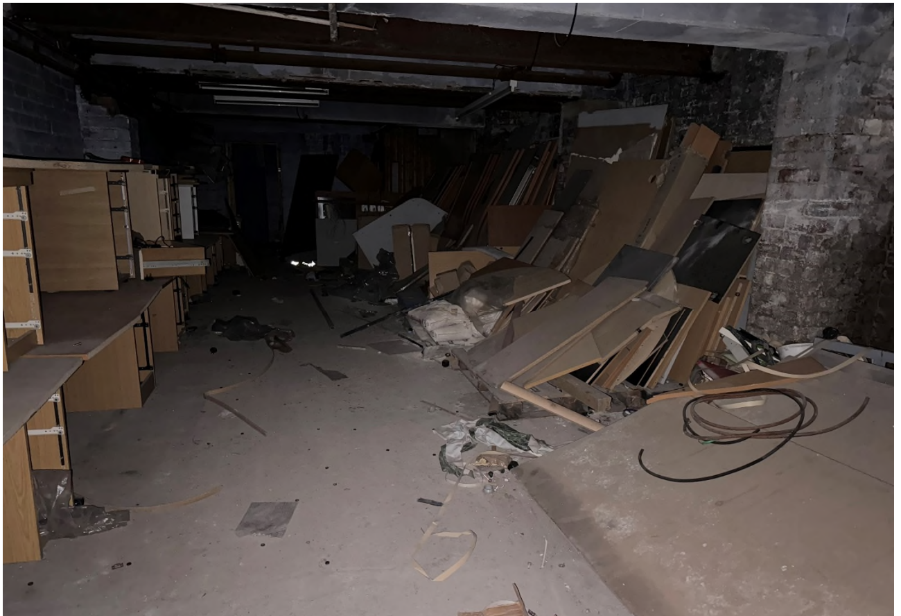
Photograph No 8 - Albion House Semi-Basement
