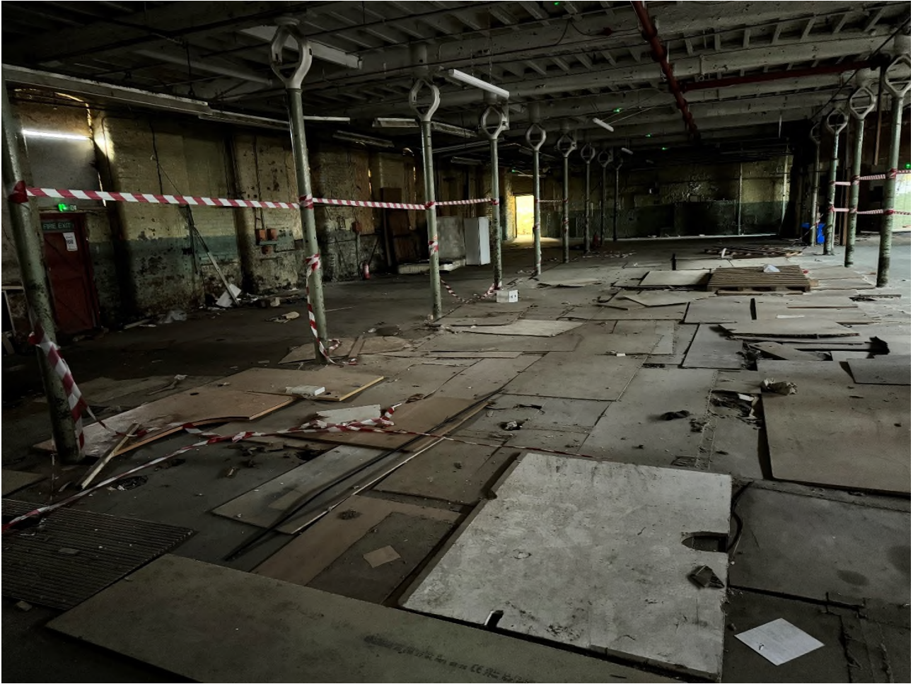
Photograph No 16 - Internal View of Albion Mill
