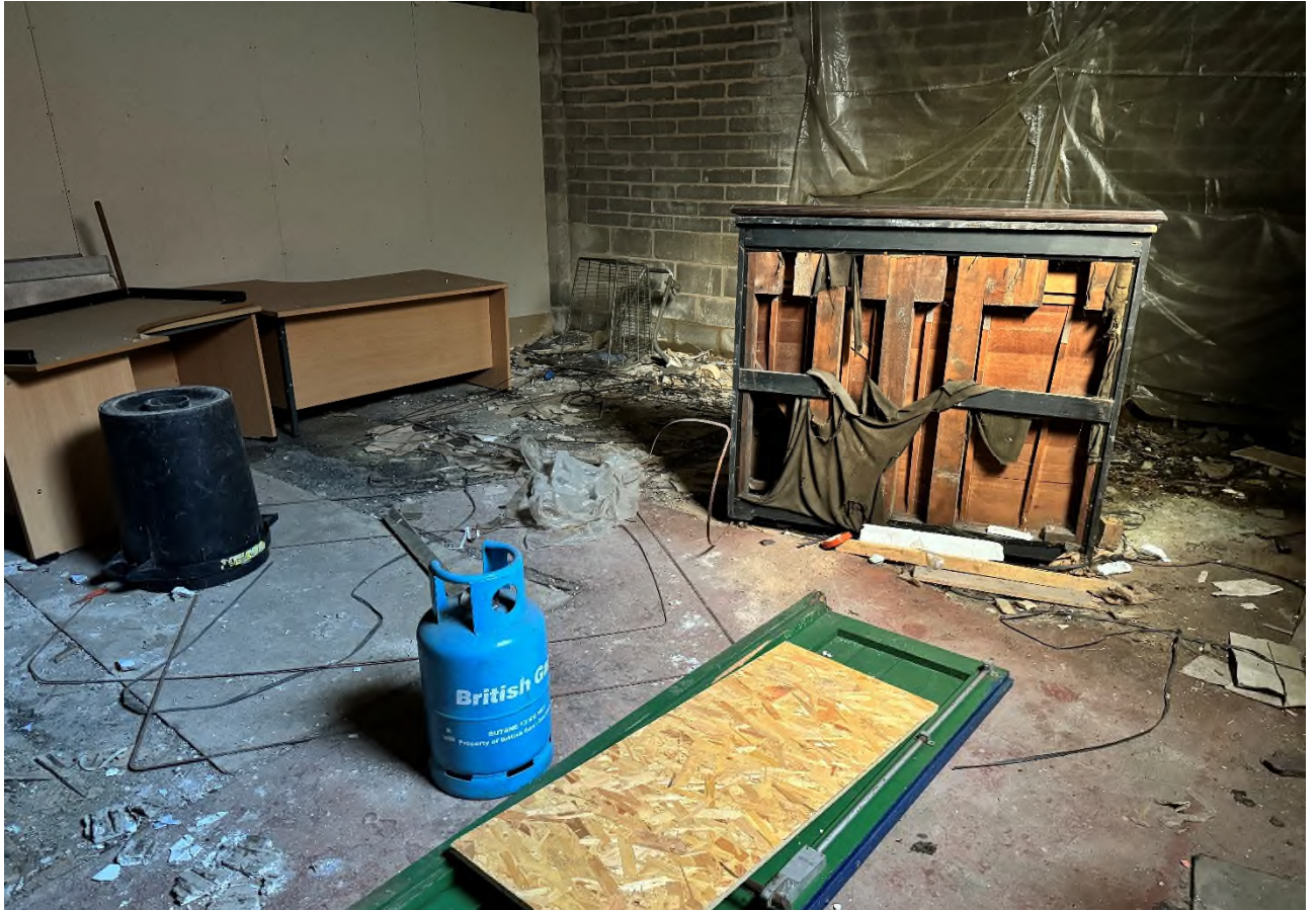
Photograph No 18 - Internal View of Albion Mill
