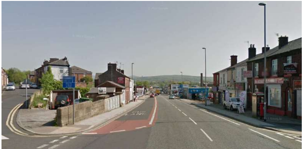
View along A58 (north-eastbound direction) west of Site
