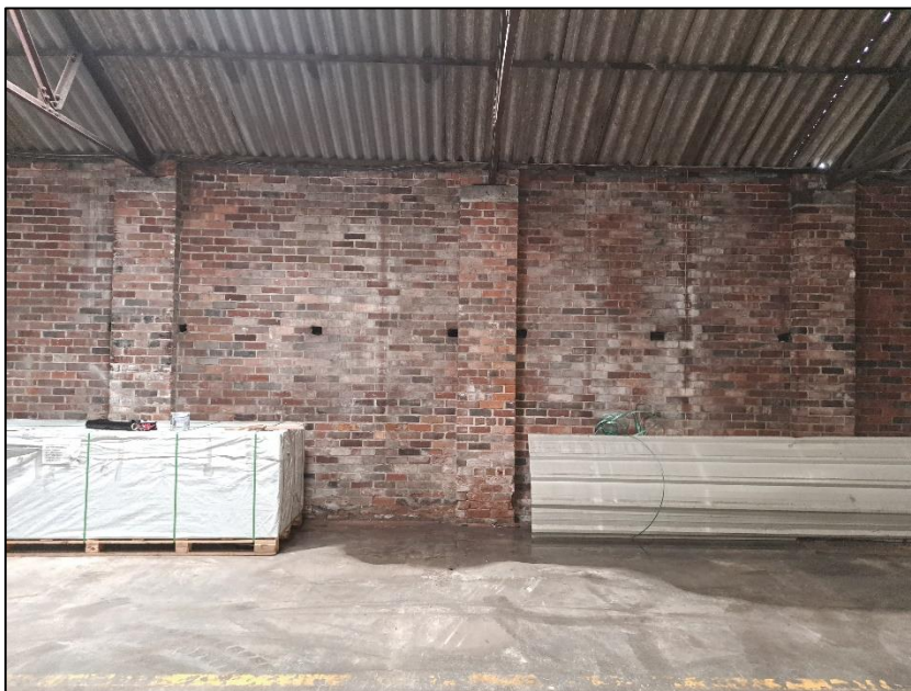
Photograph 7 showing holes that allow access to the wall cavity
