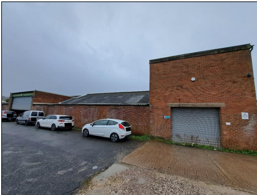
Photograph 1 showing exterior of building from Chelsea Street elevation
