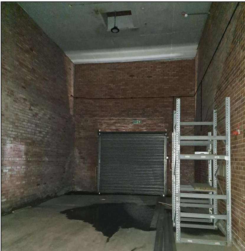
Photograph 9 showing rear flat roof section
