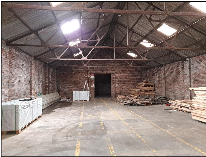
Photograph 6 showing section of internal space lit by skylights
