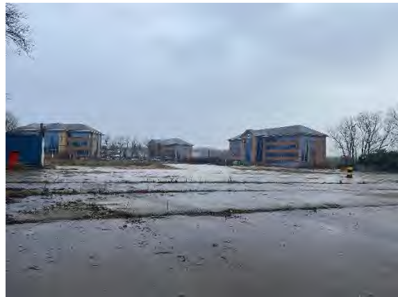
Photograph 2 – Area of hardstanding encompassing the centre and the south of the site
