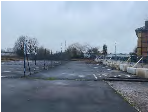
Photograph 1 – Area of hardstanding at the north-east of the site
