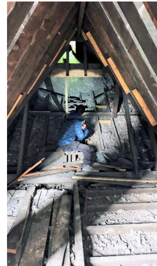
Left: roof space above nave in main worship space; Right; roof space above transept. Sufficient space for mineral wool insulation to be laid and ventilation to be maintained.
