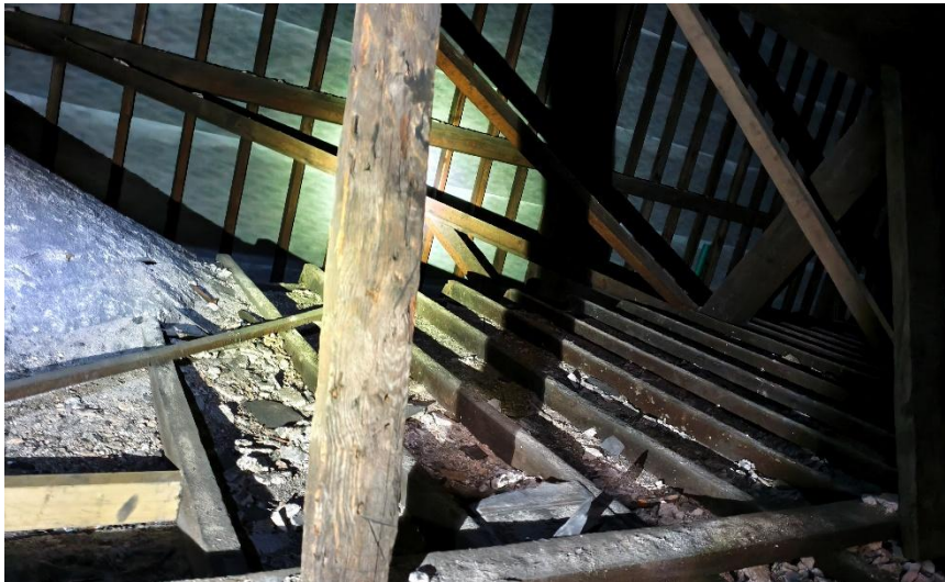
Left: roof space above nave in main worship space; Right; roof space above transept. Sufficient space for mineral wool insulation to be laid and ventilation to be maintained.
