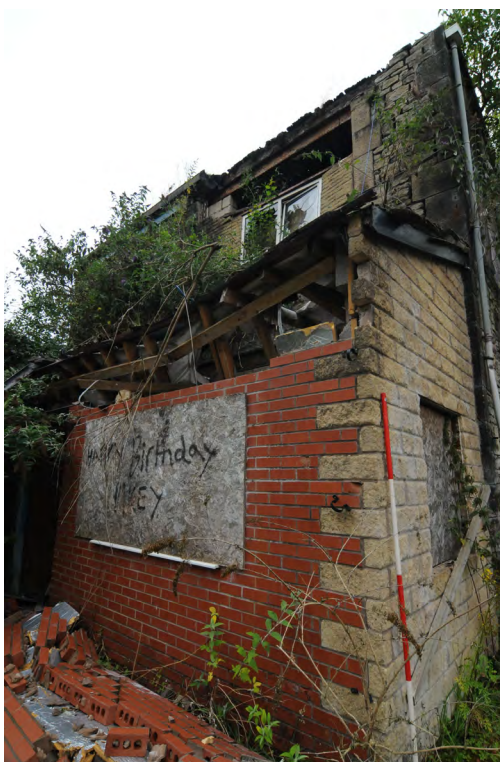
Photograph No : 46 Digital Ref: HOMI_HBR_0112 Direction: SW Description: Brick east elevation of single storey addition of Building B
