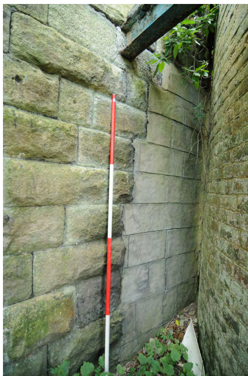
Photograph No : 73 Digital Ref: HOMI_HBR_0023 Direction: SW Description: Blocked opening at west extent of north elevation of Building C with chimney to north (right)
