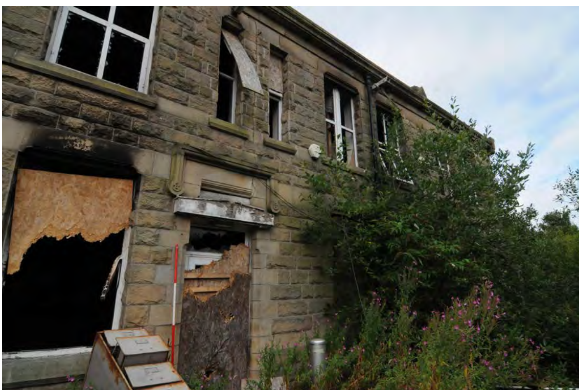
Photograph No : 8 Digital Ref: HOMI_HBR_0072 Direction: NW Description: East elevation of Building A
