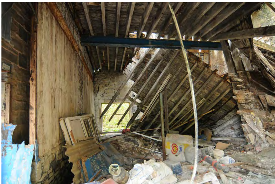
Photograph No : 52 Digital Ref: HOMI_HBR_0048 Direction: S Description: General southern view of internal area of Building B
