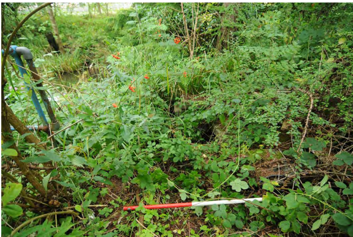
Photograph No : 5 Digital Ref: HOMI_HBR_0111 Direction: W Description: Sluice in goit
