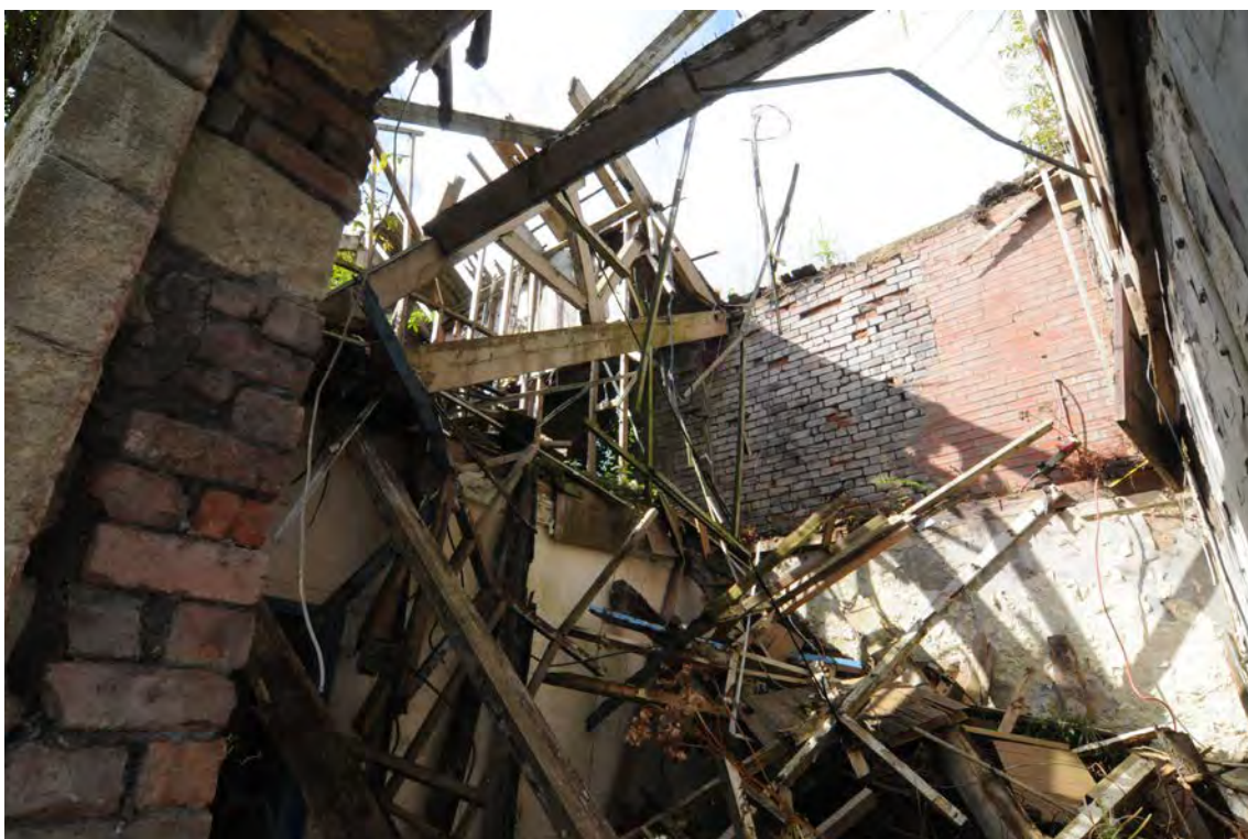
Photograph No : 82 Digital Ref: HOMI_HBR_0017 Direction: SW Description: SW view into ground and first floor of Building C
