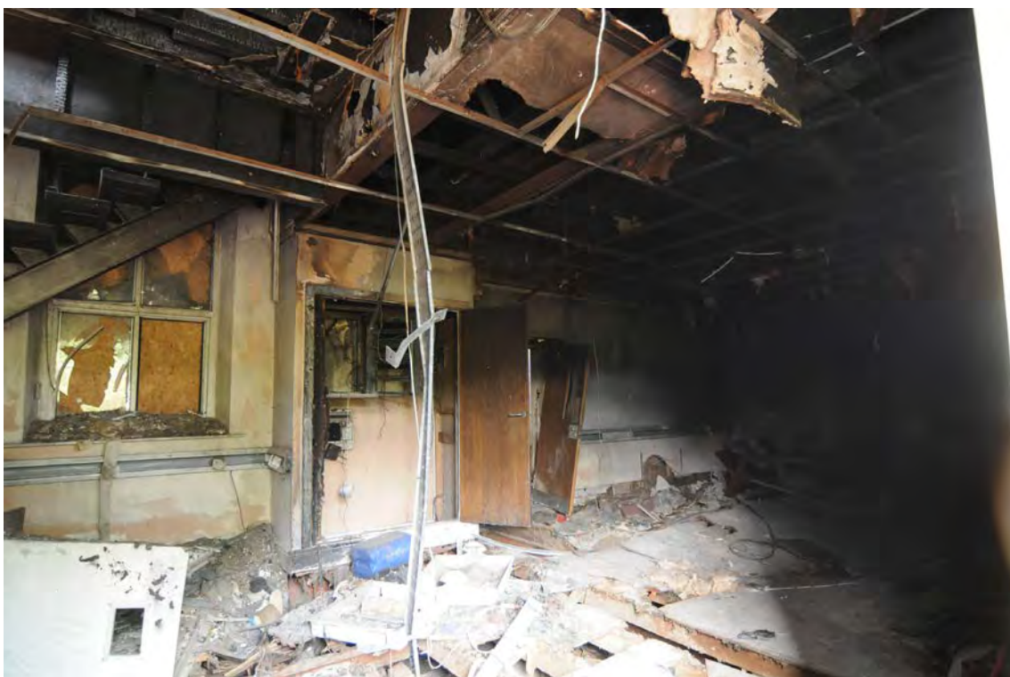
Photograph No : 20 Digital Ref: HOMI_HBR_0068 Direction: NW Description: General NW view of internal ground floor of Building A
