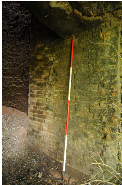
Photograph No : 90 Digital Ref: HOMI_HBR_0030 Direction: NE Description: East wall in opening in south side of chimney
