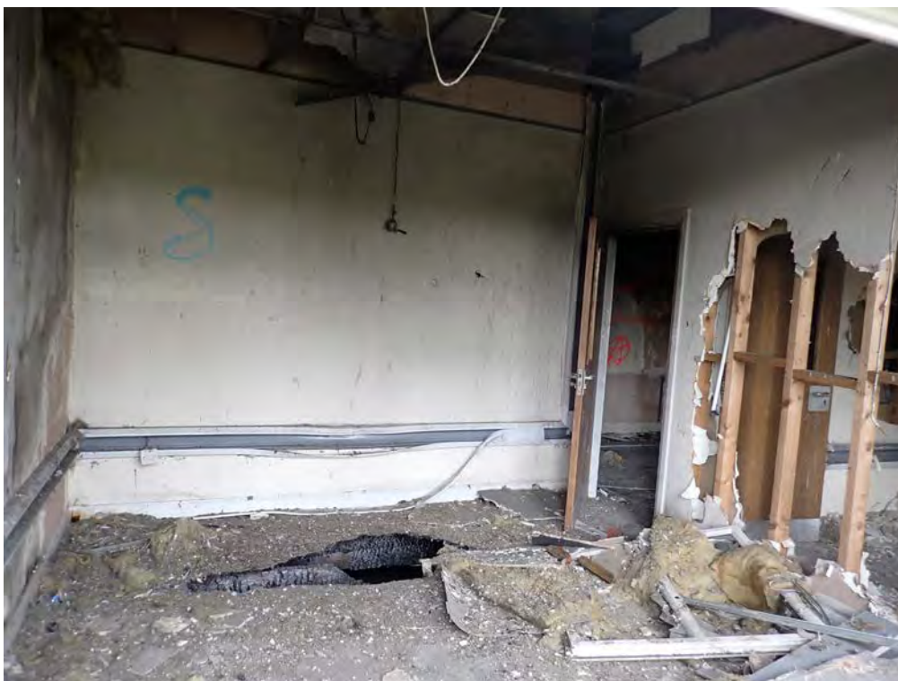
Photograph No : 23 Digital Ref: HOMI_HBR_0104 Direction: W Description: General view of first floor of Building A
