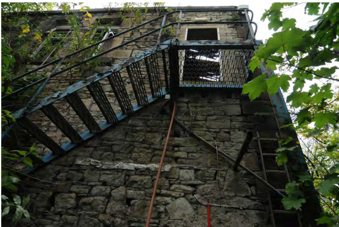
Photograph No : 43 Digital Ref: HOMI_HBR_0060 Direction: S Description: Ground and first floor of north elevation of Building B with fire escape
