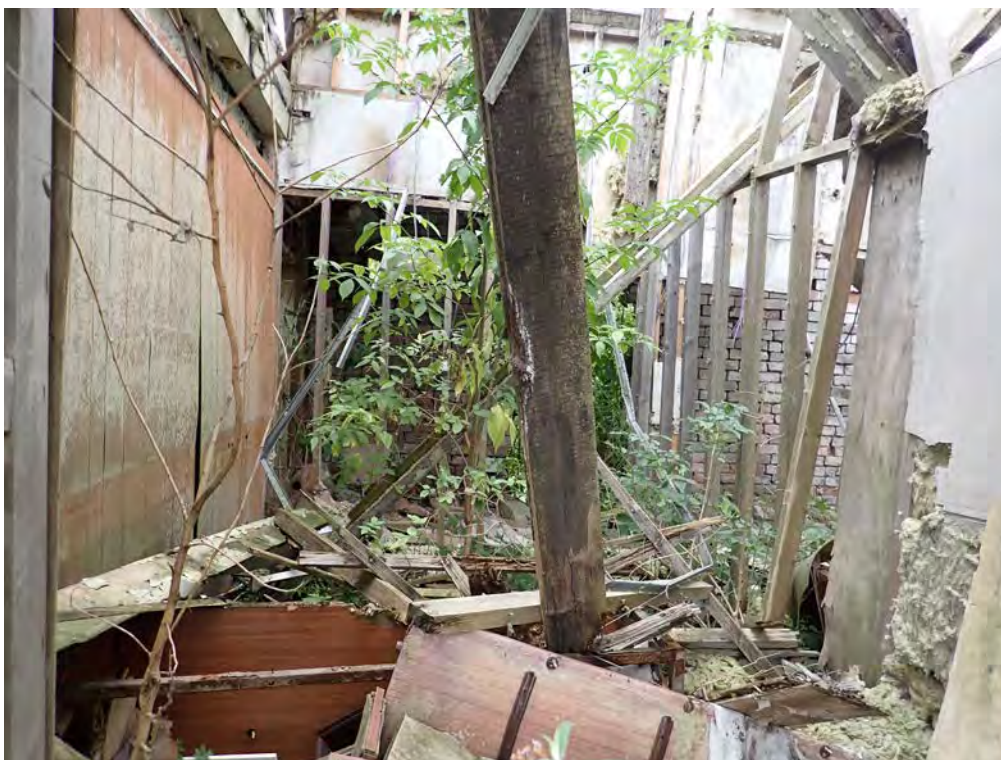
Photograph No : 79 Digital Ref: HOMI_HBR_0090 Direction: W Description: General view of first floor of Building C
