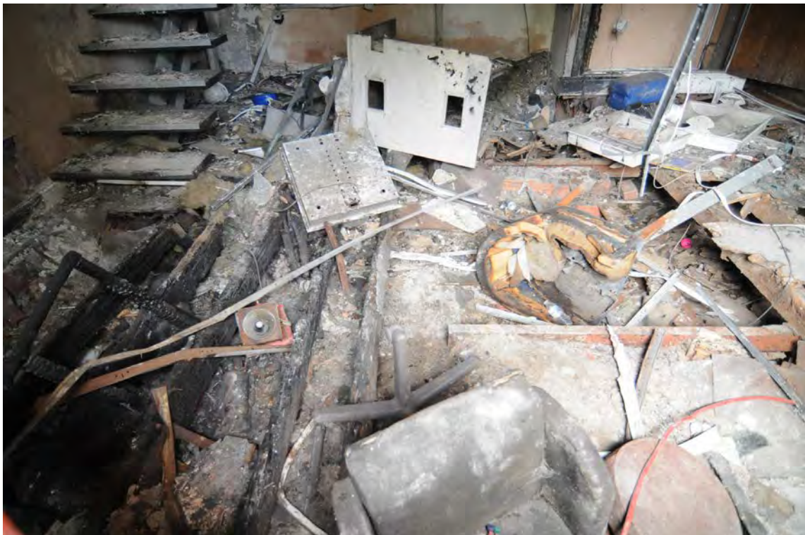
Photograph No : 22 Digital Ref: HOMI_HBR_0071 Direction: W Description: Ground in ground floor of Building A
