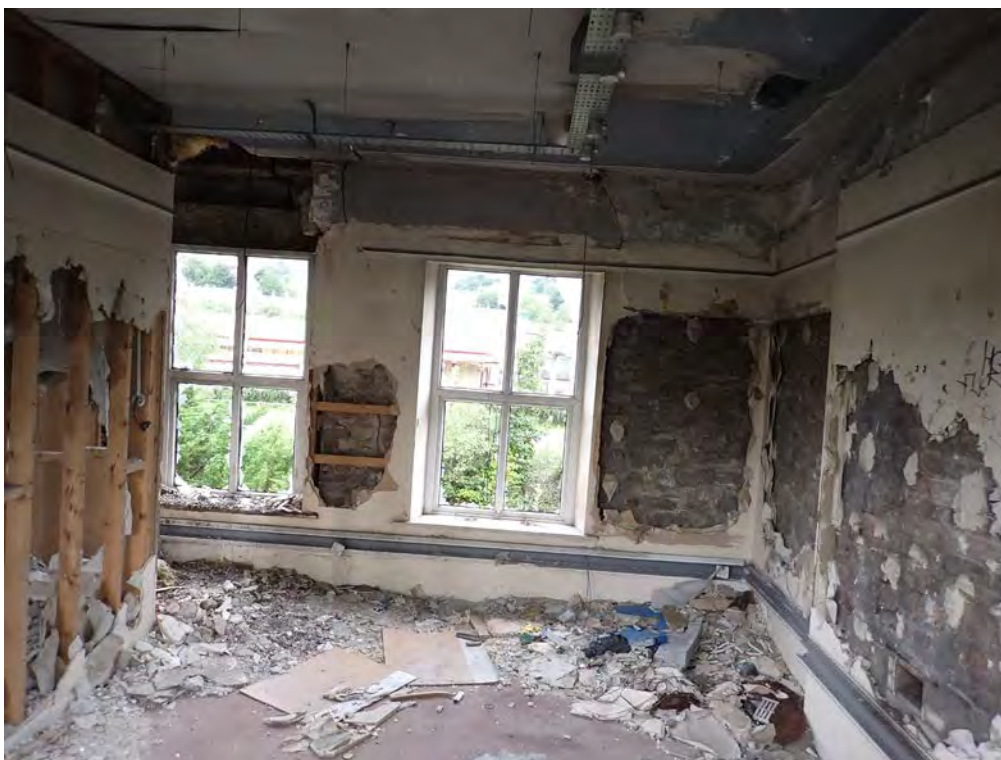
Photograph No : 25 Digital Ref: HOMI_HBR_0108 Direction: W Description: General view of first floor of Building A, blocked fireplace and chimney at the north (right)
