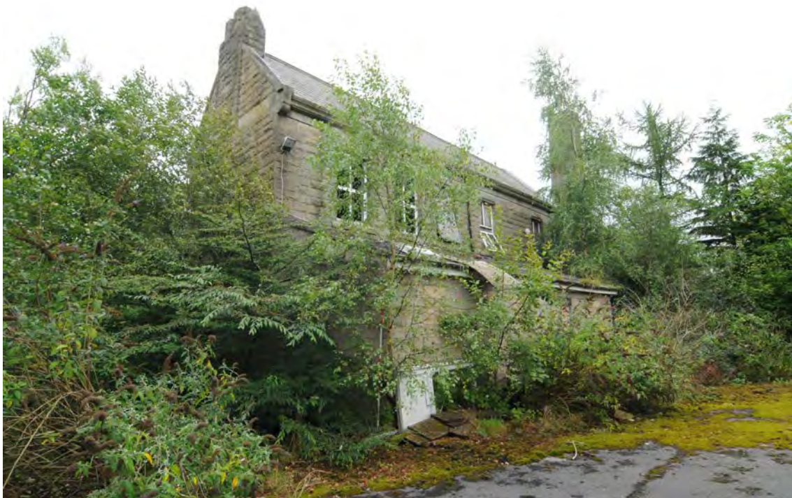
Photograph No : 9 Digital Ref: HOMI_HBR_0080 Direction: SE Description: West elevation and north gable of Building A with single storey addition
