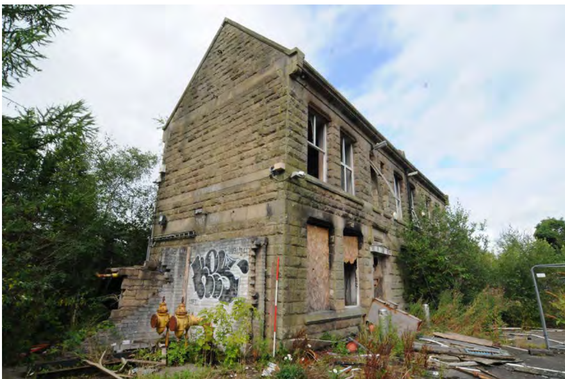
Photograph No : 6 Digital Ref: HOMI_HBR_0065 Direction: NW Description: South gable and east elevation of Building A
