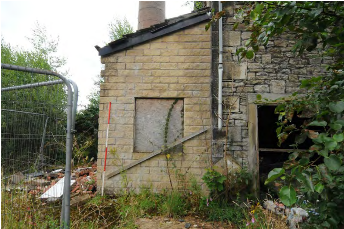
Photograph No : 47 Digital Ref: HOMI_HBR_0044 Direction: S Description: North elevation of addition of Building B with Chimney in background
