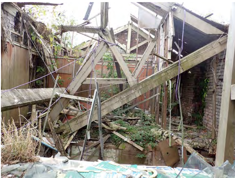
Photograph No : 84 Digital Ref: HOMI_HBR_0092 Direction: S Description: King post trusses and general view of first floor of Building C
