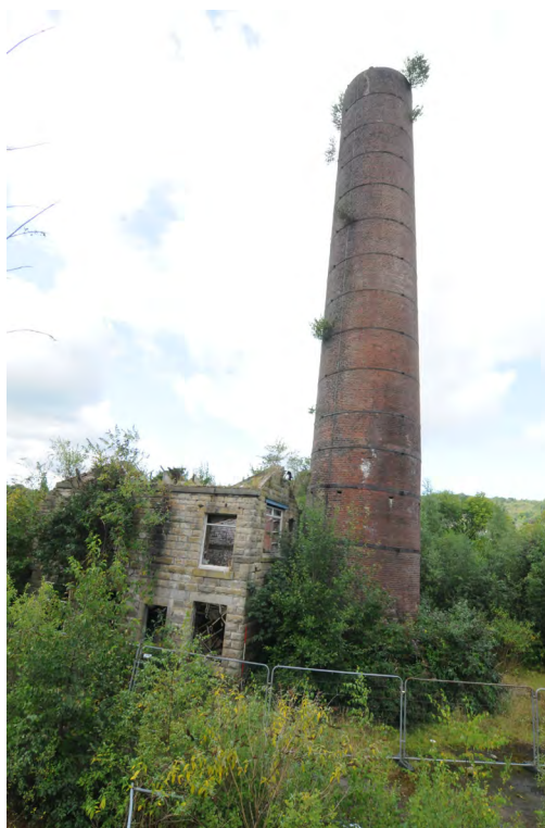
Photograph No : 60 Digital Ref: HOMI_HBR_0005 Direction: SW Description: East and north elevations of Building C and Chimney
