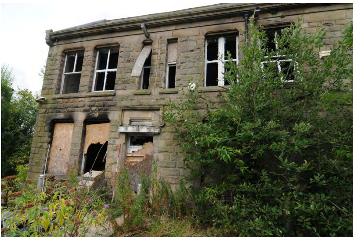
Photograph No : 15 Digital Ref: HOMI_HBR_0073 Direction: SW Description: Southern extent of east elevation of Building A
