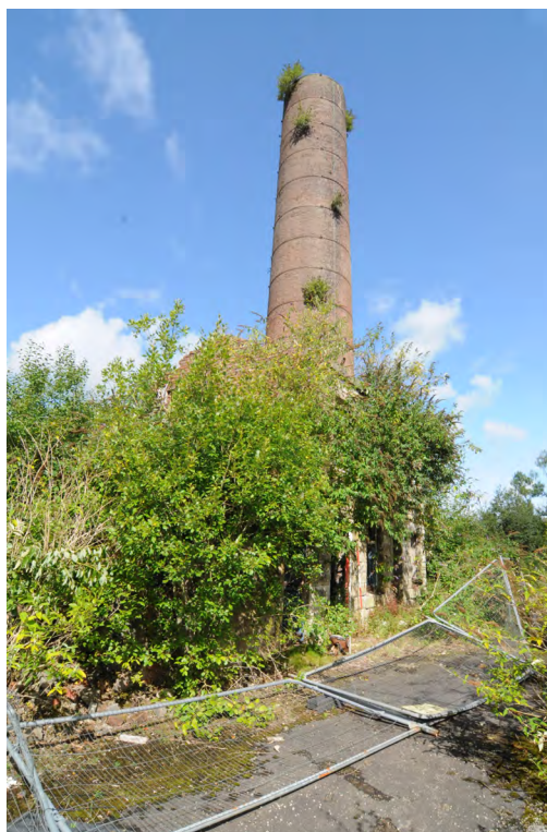
Photograph No : 59 Digital Ref: HOMI_HBR_0001 Direction: NW Description: East elevation of Building C and Chimney
