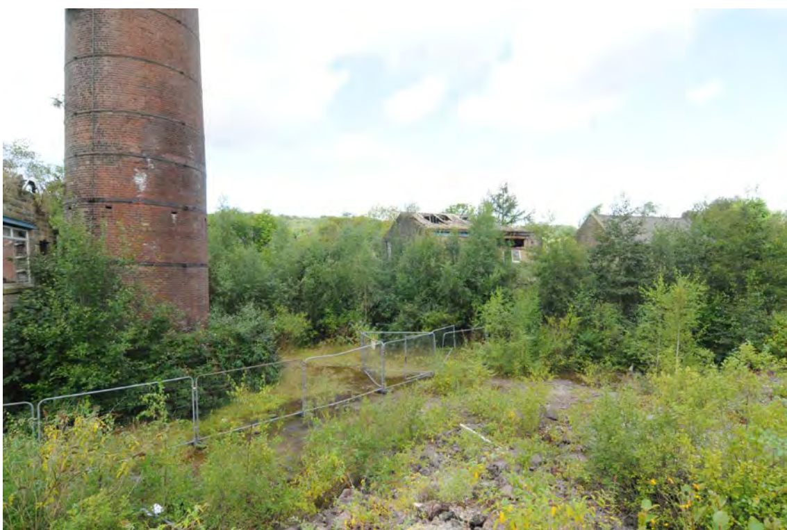
Photograph No : 2 Digital Ref: HOMI_HBR_0006 Direction: NW Description: NW view of site with Building A at north (right), Building B (centre), Building C and Chimney at south (left)
