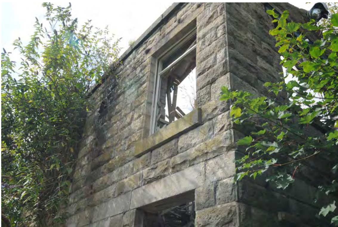
Photograph No : 67 Digital Ref: HOMI_HBR_0026 Direction: SW Description: First floor east elevation of Building C with window exposing internal brick
