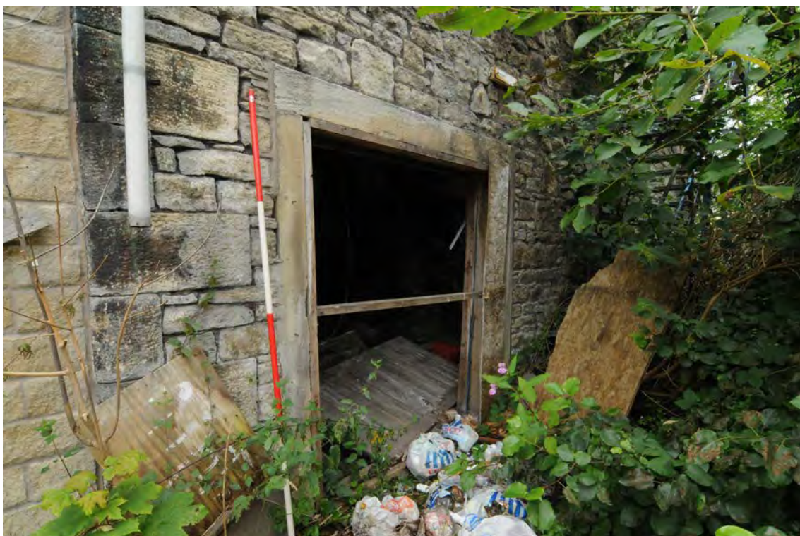
Photograph No : 41 Digital Ref: HOMI_HBR_0046 Direction: SW Description: Detail of ground floor fenestration in north elevation of Building B
