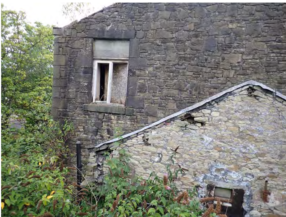
Photograph No : 34 Digital Ref: HOMI_HBR_0102 Direction: NW Description: South gable of Building B with blocked fenestration at the first floor, gable scar of former building, bearing box
