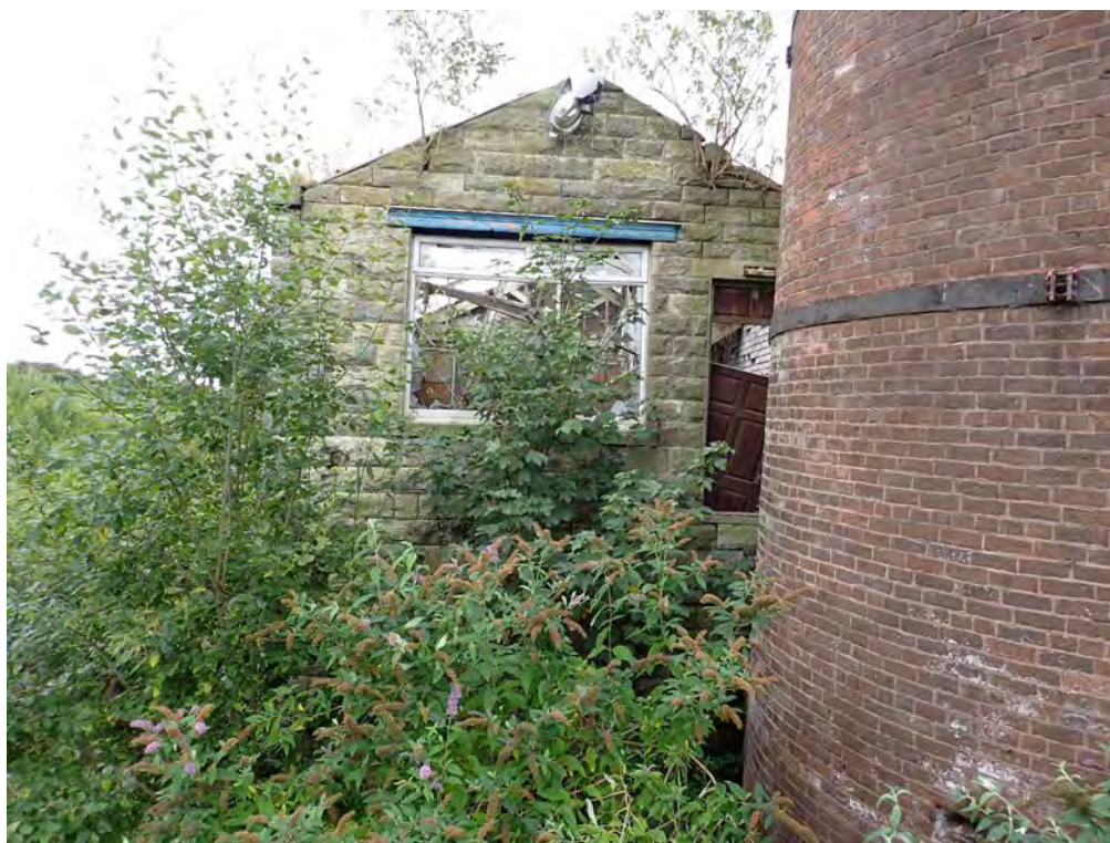
Photograph No : 68 Digital Ref: HOMI_HBR_0096 Direction: S Description: North gable of Building C with Chimney at NW (right)
