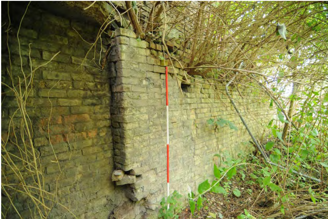
Photograph No : 85 Digital Ref: HOMI_HBR_0034 Direction: SE Description: West elevation of Building C
