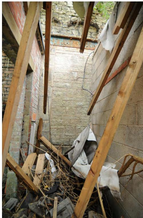
Photograph No : 48 Digital Ref: HOMI_HBR_0114 Direction: W Description: Blocked fenestration in west elevation of Building B and general internal view of ground floor area of addition
