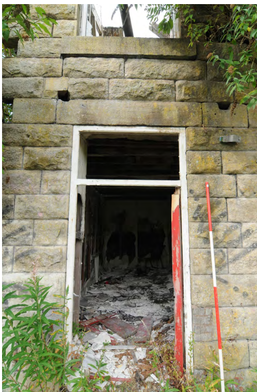
Photograph No : 71 Digital Ref: HOMI_HBR_0009 Direction: W Description: East elevation of Building C, westward view into ground floor
