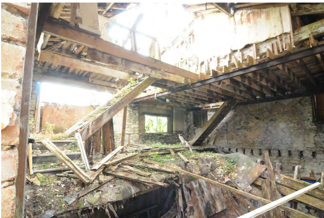
Photograph No : 58 Digital Ref: HOMI_HBR_0054 Direction: SE Description: General SE view of first floor internal area of Building B with stairs
