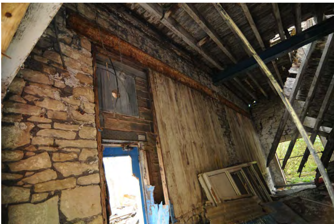
Photograph No : 56 Digital Ref: HOMI_HBR_0051 Direction: SE Description: Opening of east wall of Building B with façade wall beyond
