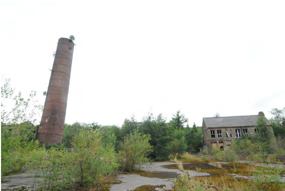
Photograph No : 1 Digital Ref: HOMI_HBR_0089 Direction: W Description: Westward view of site with Building A at north (right), Building B (centre, behind vegetation), Building C and Chimney at south (left)
