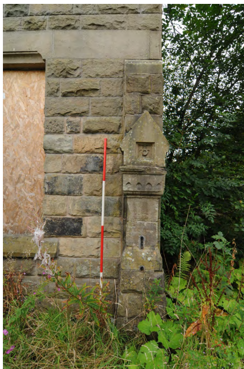
Photograph No : 11 Digital Ref: HOMI_HBR_0075 Direction: W Description: East face of gate post at north extent of east elevation of Building A
