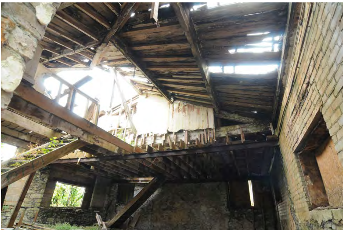
Photograph No : 55 Digital Ref: HOMI_HBR_0056 Direction: S Description: General southern view of first floor internal area of Building B
