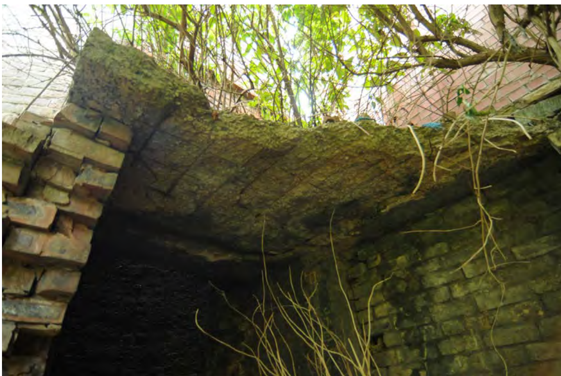
Photograph No : 94 Digital Ref: HOMI_HBR_0036 Direction: NE Description: Reinforced concrete above southern opening in Chimney with west elevation of Building C in back-ground
