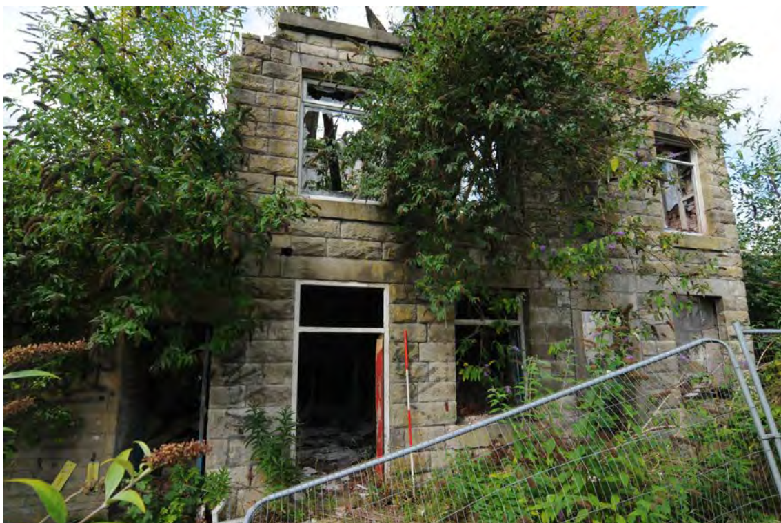
Photograph No : 62 Digital Ref: HOMI_HBR_0003 Direction: W Description: East elevation of Building C
