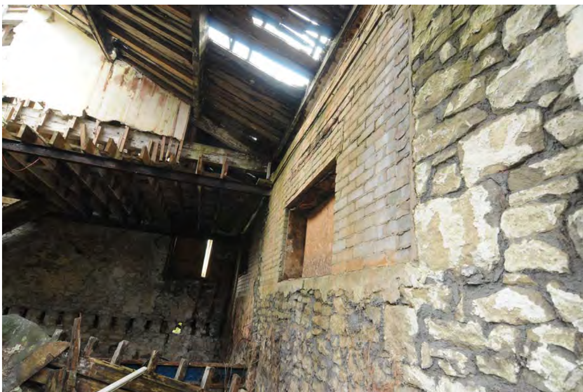
Photograph No : 44 Digital Ref: HOMI_HBR_0055 Direction: SW Description: Brick blocked fenestration at first floor in west wall of Building B
