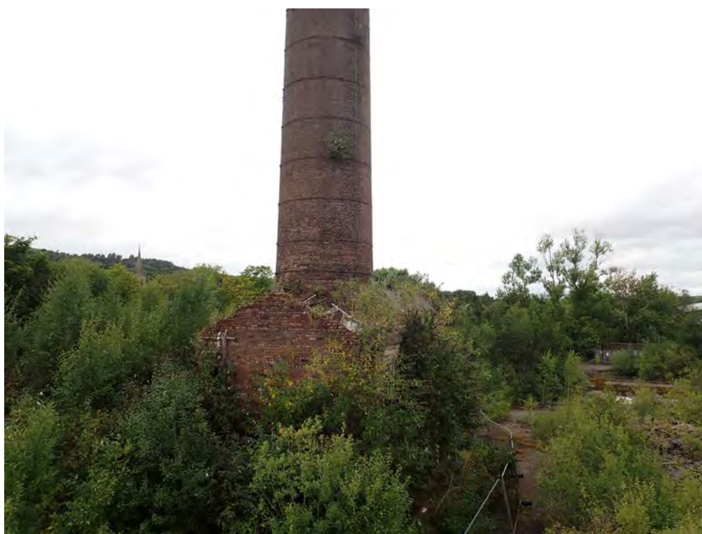
Photograph No : 64 Digital Ref: HOMI_HBR_0097 Direction: N Description: South gable of Building C with chimney in background
