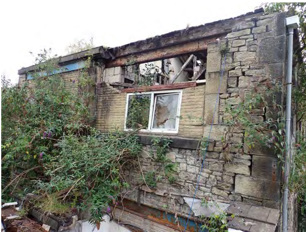
Photograph No : 51 Digital Ref: HOMI_HBR_0099 Direction: SW Description: Blocked window in first floor east elevation of Building B
