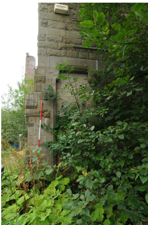
Photograph No : 14 Digital Ref: HOMI_HBR_0079 Direction: S Description: Stone blocked doorway at eastern side of north gable
