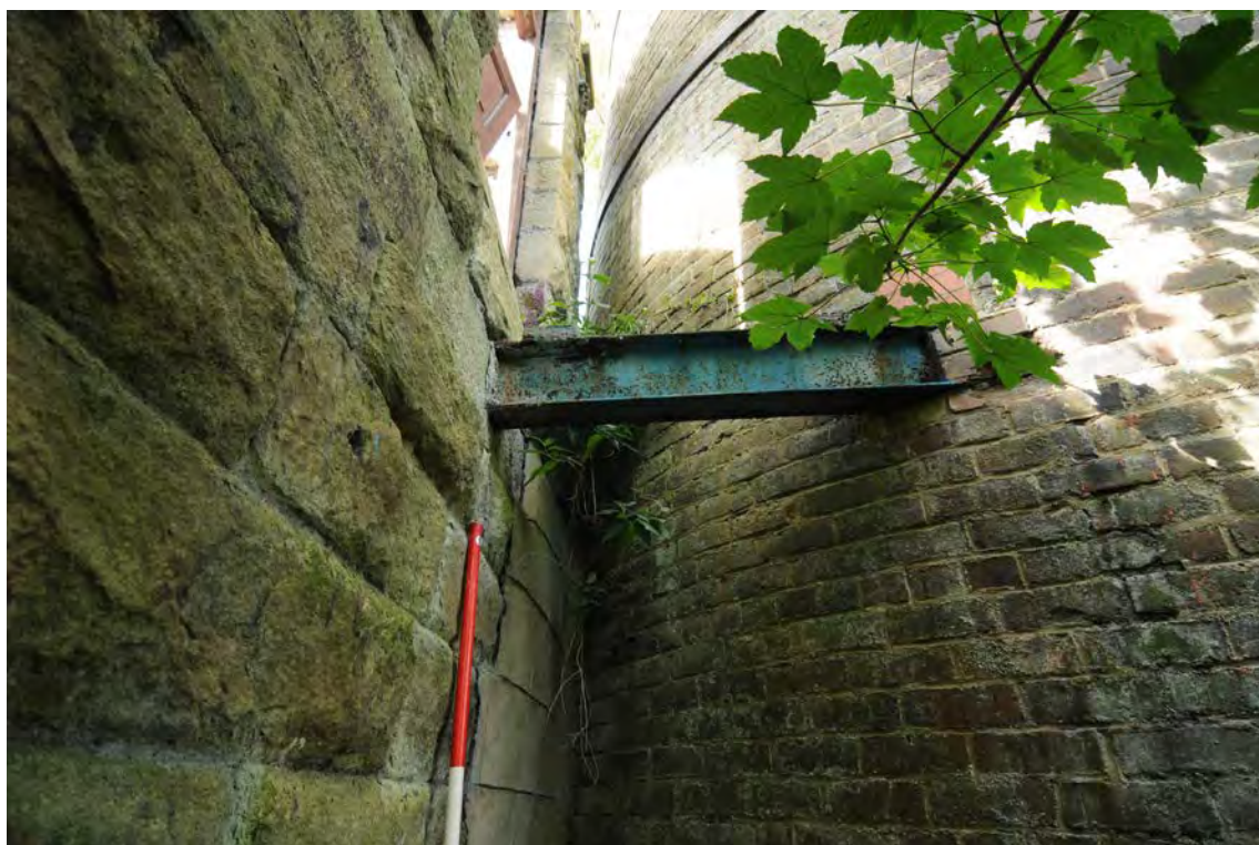
Photograph No : 74 Digital Ref: HOMI_HBR_0024 Direction: SW Description: Detail of steel I-beam between north elevation and chimney
