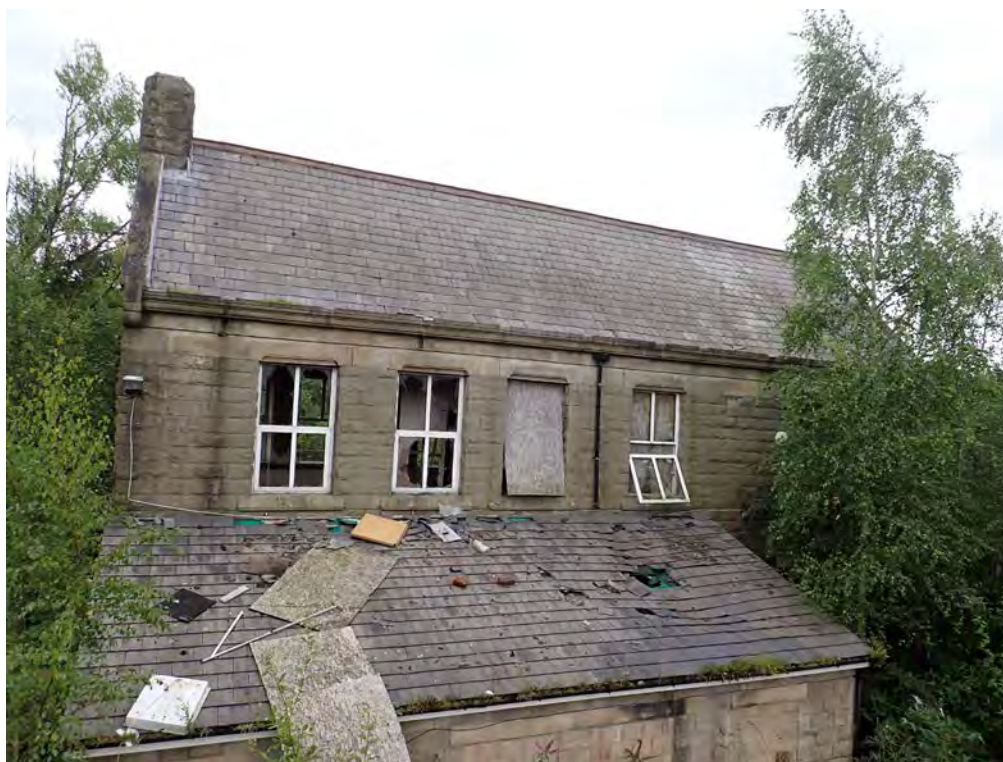
Photograph No : 16 Digital Ref: HOMI_HBR_0110 Direction: SE Description: Chimney, ridge, and first floor windows on west elevation of Building A
