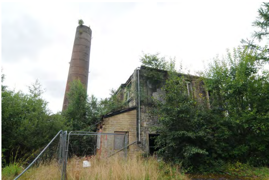
Photograph No : 26 Digital Ref: HOMI_HBR_0041 Direction: S Description: North elevation of Building B with Chimney in background
