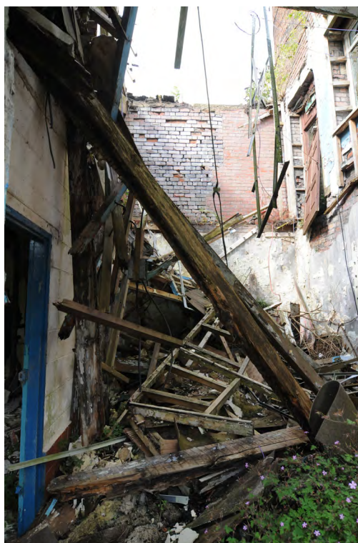
Photograph No : 80 Digital Ref: HOMI_HBR_0015 Direction: W Description: Westward view into ground and first floor of Building C
