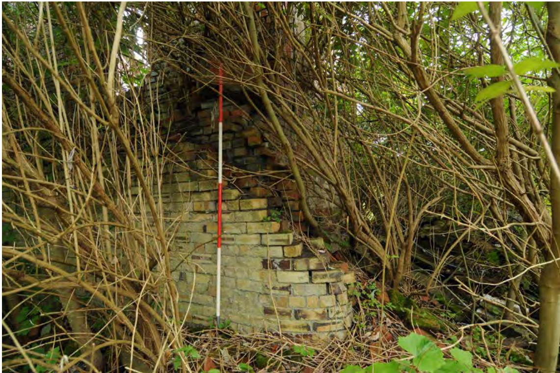
Photograph No : 87 Digital Ref: HOMI_HBR_0038 Direction: NE Description: Curve in brick at ground floor southern extent of west elevation of Building C
