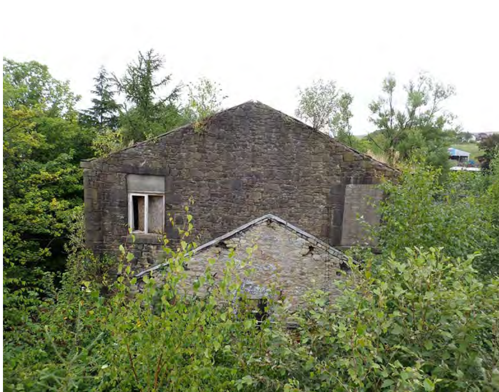
Photograph No : 32 Digital Ref: HOMI_HBR_0100 Direction: N Description: South gable of Building B with blocked fenestration at the first floor and gable scar of former building
