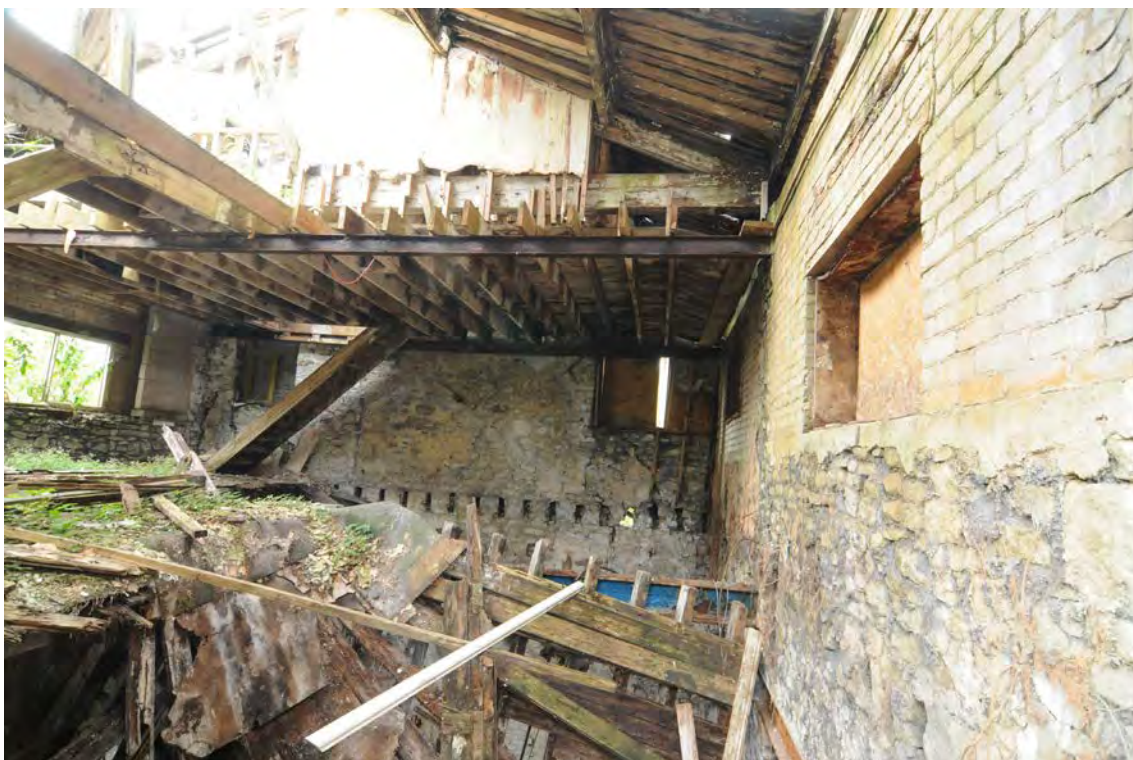
Photograph No : 57 Digital Ref: HOMI_HBR_0053 Direction: S Description: General southern view of first floor internal area of Building B
