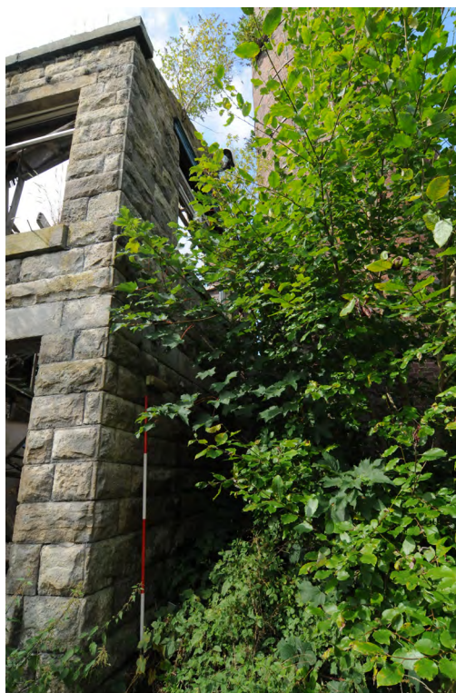
Photograph No : 65 Digital Ref: HOMI_HBR_0019 Direction: SW Description: Oblique view of east elevation (left) and north elevation of Building C with Chimney in background
