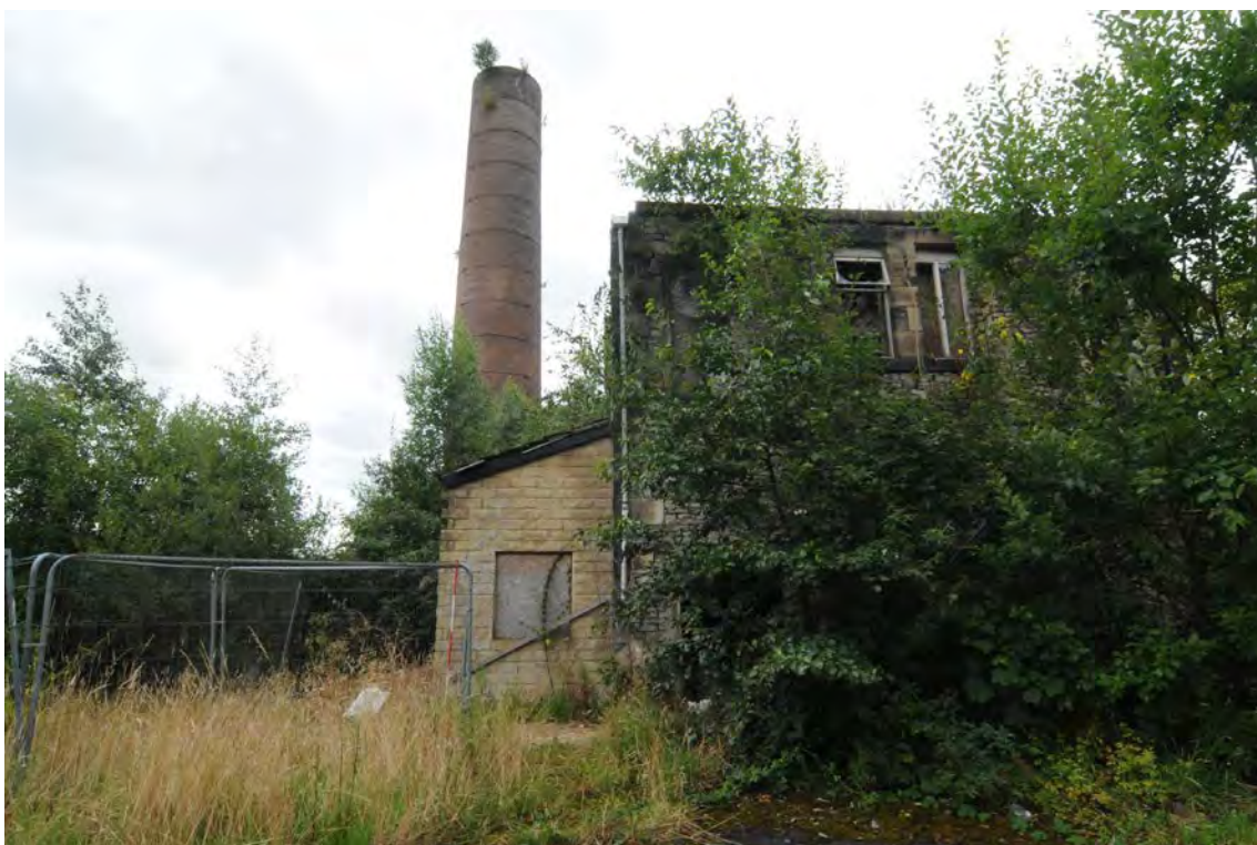
Photograph No : 42 Digital Ref: HOMI_HBR_0042 Direction: S Description: North elevation of Building B with Chimney in background
