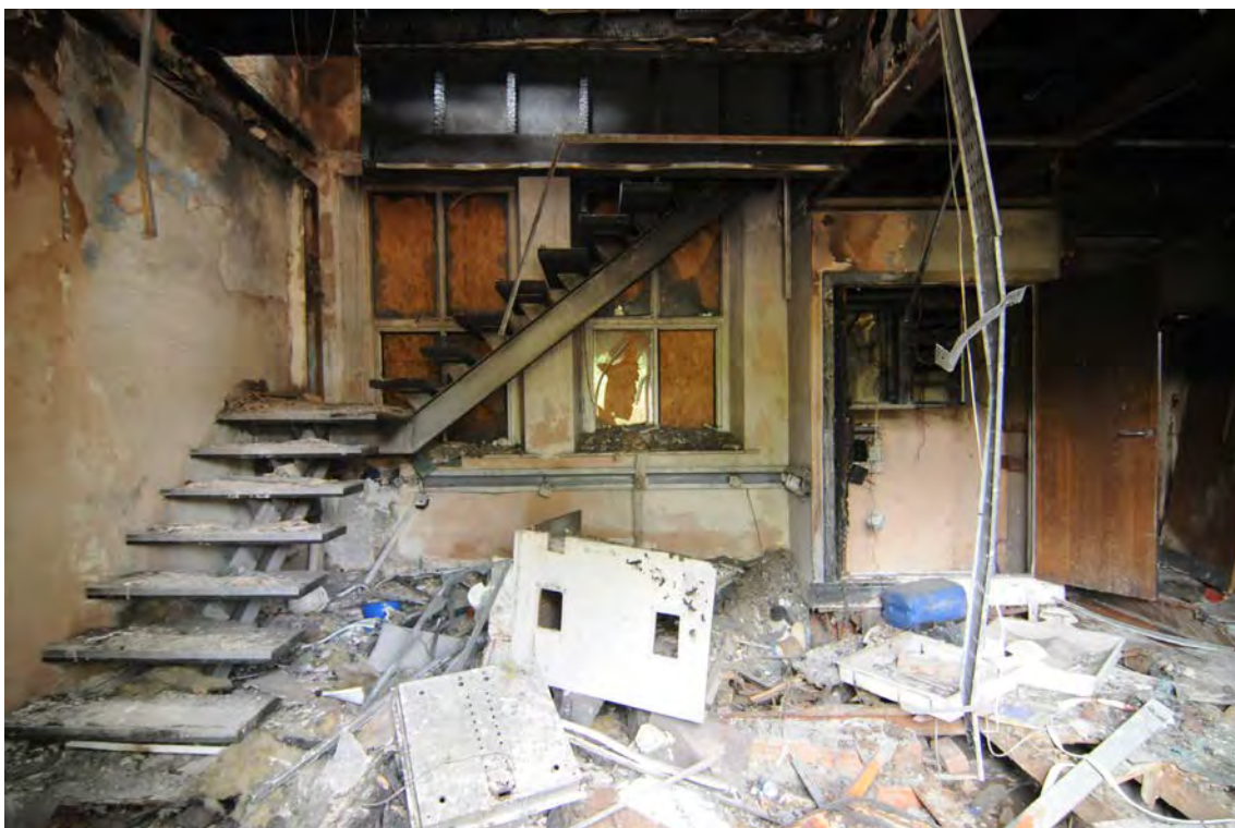
Photograph No : 19 Digital Ref: HOMI_HBR_0067 Direction: W Description: Internal ground floor of Building A with stairs in SW corner
