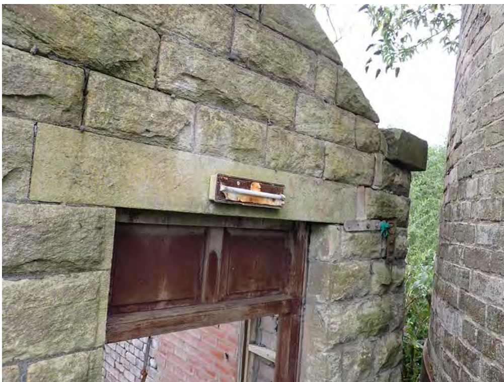
Photograph No : 69 Digital Ref: HOMI_HBR_0095 Direction: SW Description: Detail of lintel above first floor doorway in north gable of Building C with chimney at west (right)
